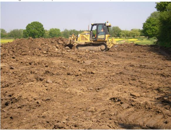
Plate 1. Bulldozer stripping topsoil
