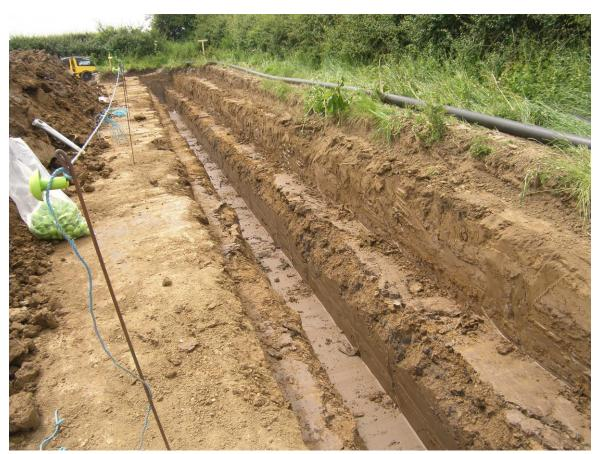
Plate 2. Sample section of pipe trench showing boulder clay
