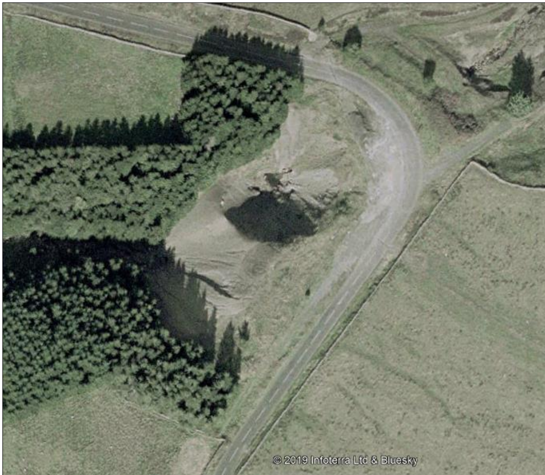
Figure 2. Crater within spoil heap caused by broken culvert, as depicted on Google Earth © 2019 Google © 2019 Infoterra Ltd & Bluesky
