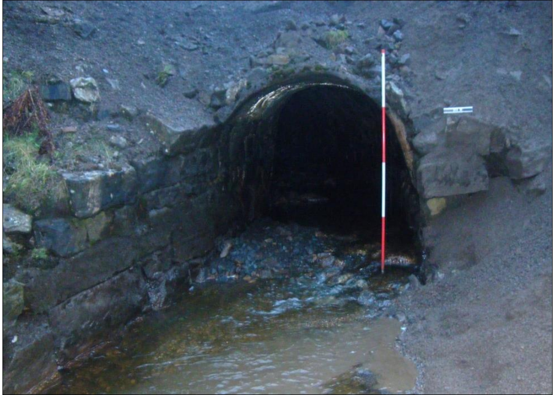
Plate 2. Entrance to western section of culvert looking eastwards
