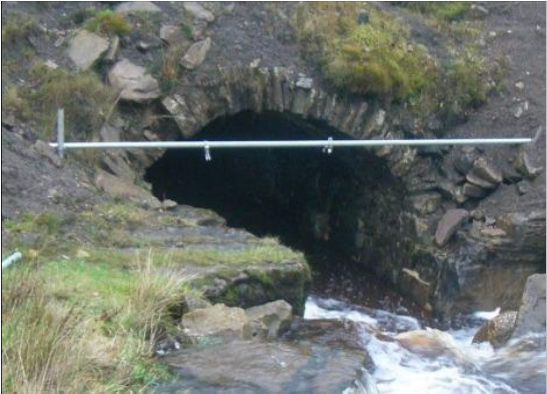
Plate 3. Culvert arch to north of road
