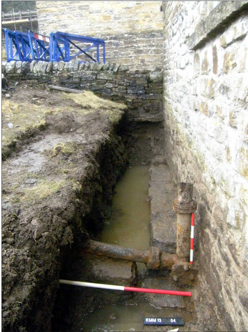
©NAA 2013 North of England Lead Mining Museum, Killhope: Plate 3 cast iron pipe 04
