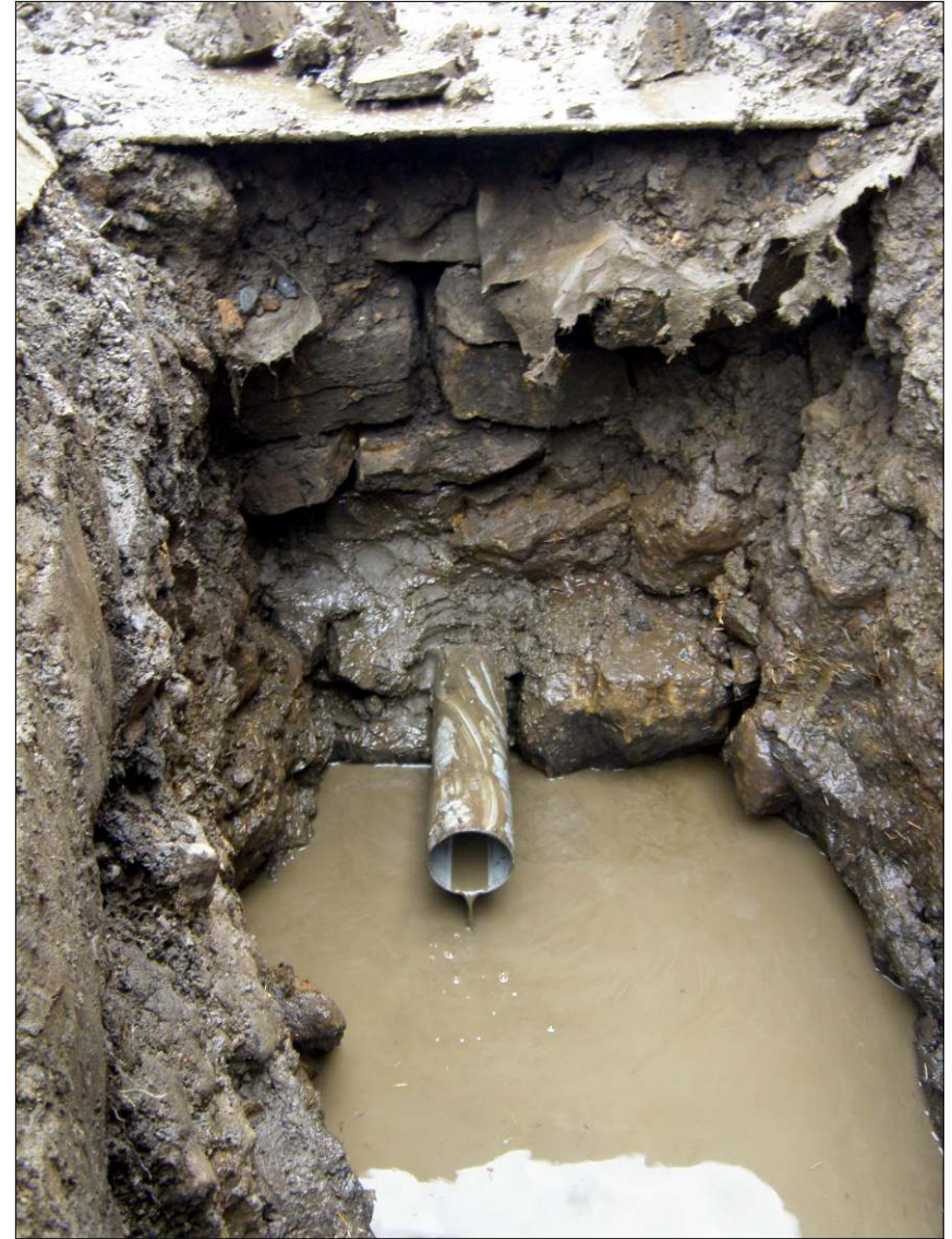
North of England Lead Mining Museum, Killhope: culvert 9 with pipe duct
