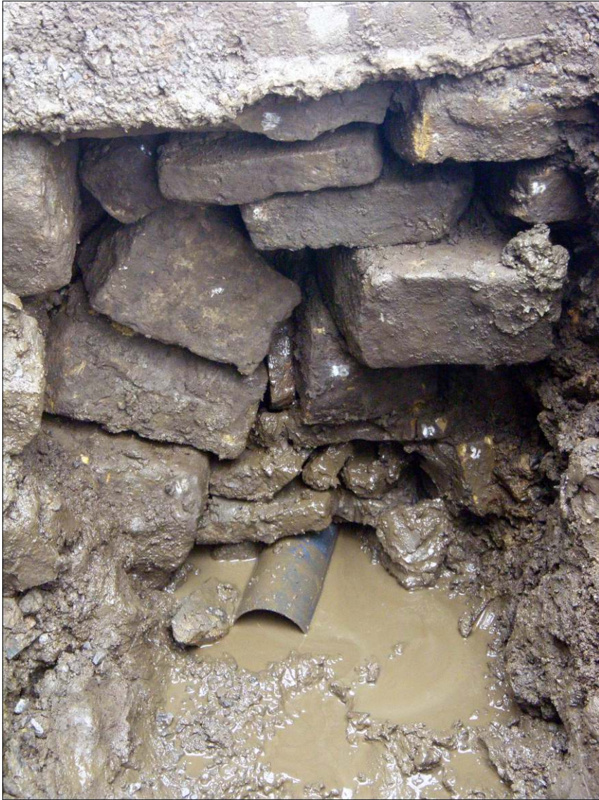
North of England Lead Mining Museum, Killhope: culvert 7 with pipe duct
