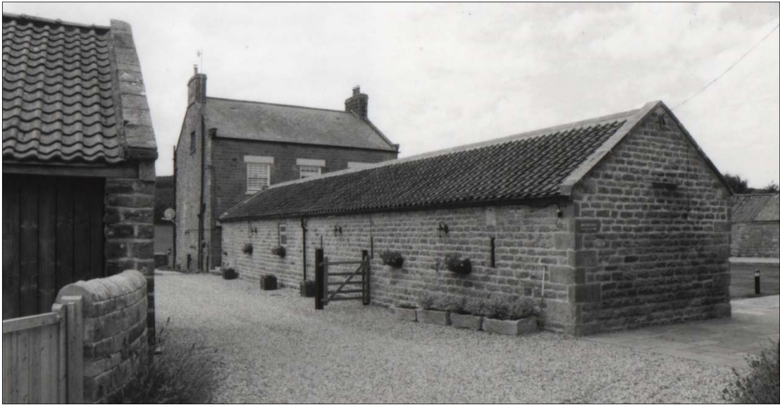
Plate 8: east elevation of the east range looking south west. (Photo by CS Archaeology 2018).
