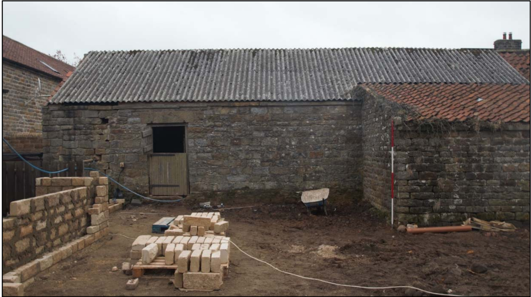
Plate 21: north end of west elevation (1300), showing northern door (101).
