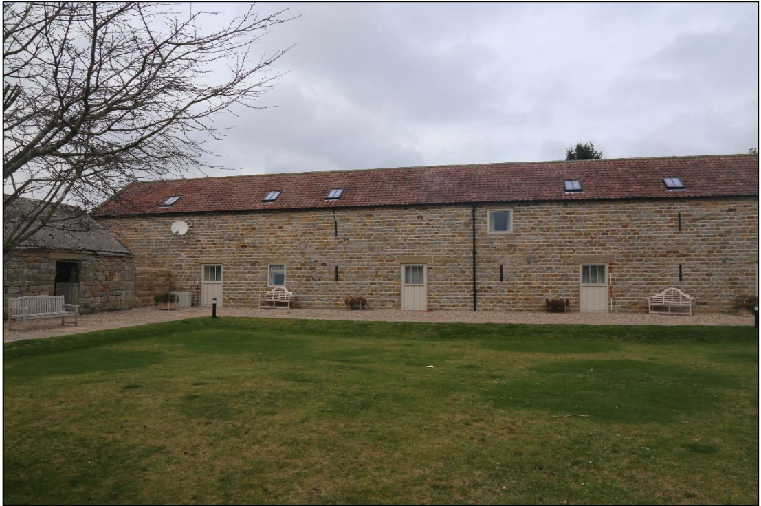
Plate 9: south elevation of the barn showing ventilation slits, indicative of hay lofts, granaries and a cattle byre.
