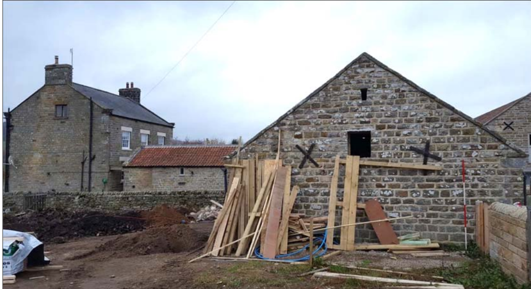
Plate 55: east facing elevation (3300) of cart shed.
