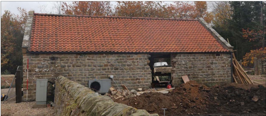
Plate 56: south elevation (3400) of the cart shed, showing opening on east side.
