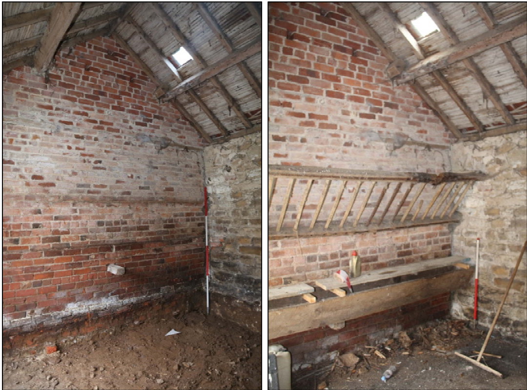
Plates 49 and 50: (left) the east partition wall of the west room is brick whereas the south is stone. The remains of a trough (2103) and hay rack (2105) are evident as wall scars and (right) both recorded by CS Archaeology 2018. (photo by CS Archaeology 2018).
