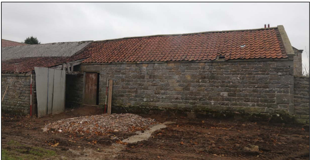
Plate 22: south end of west elevation (1300), showing southern door (301) and outshot (600).
