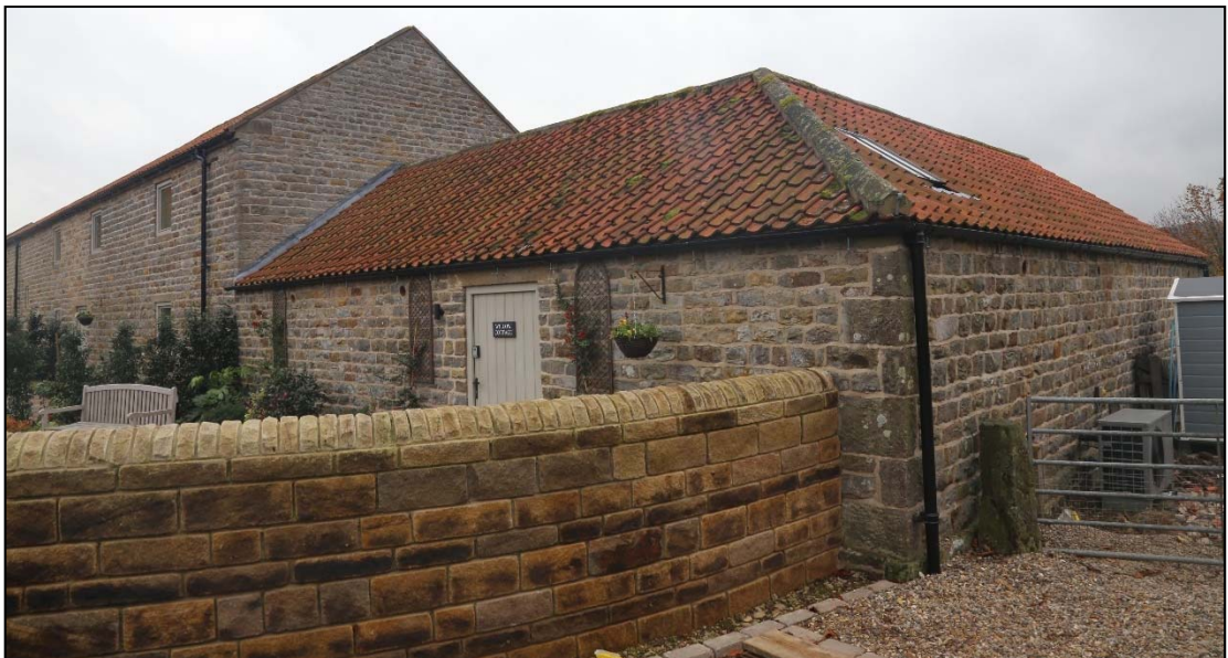
Plates 12: north facing elevation of north-west range (second cart shed).
