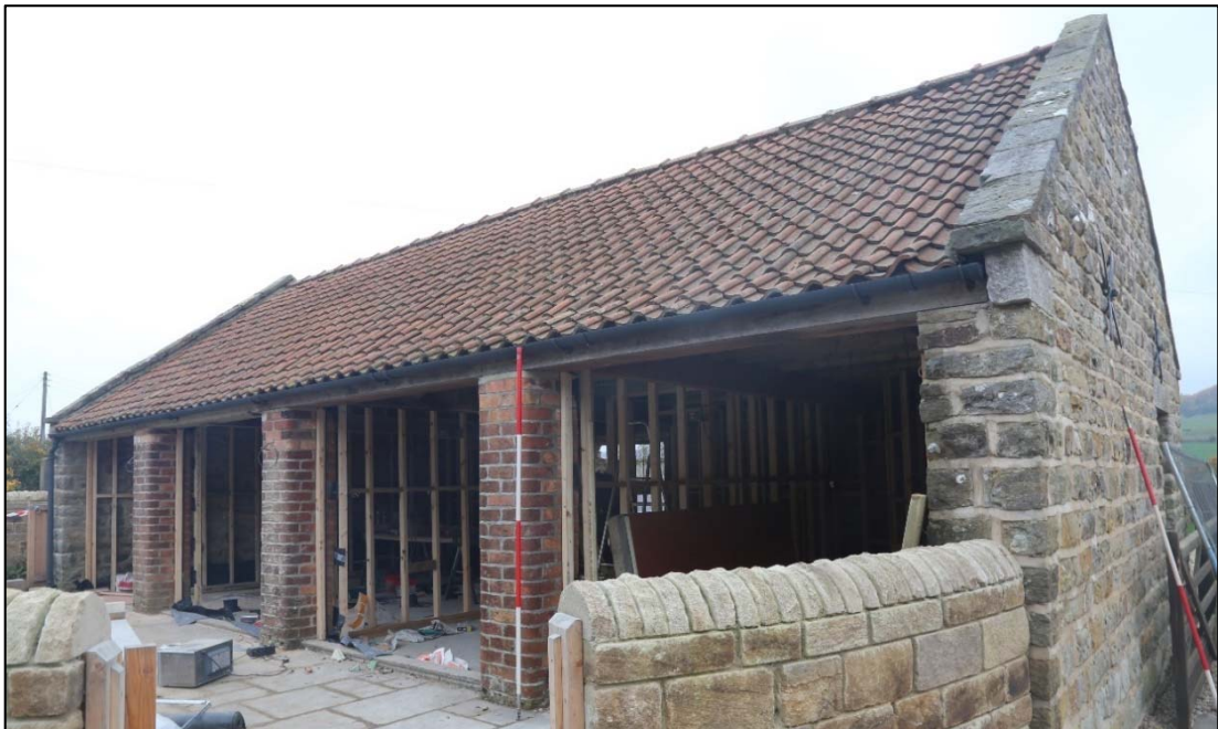
Plate 54: north elevation of the cart shed.
