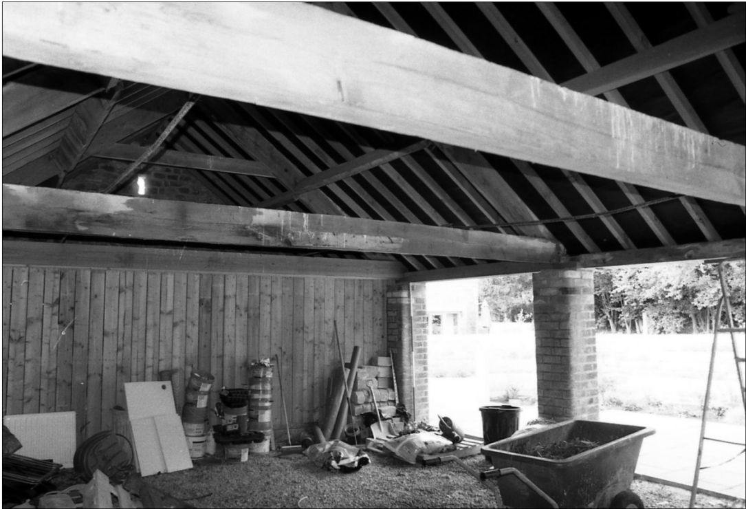
Plate 59: interior of the cart shed looking north-west. (Photo by CS Archaeology 2018).
