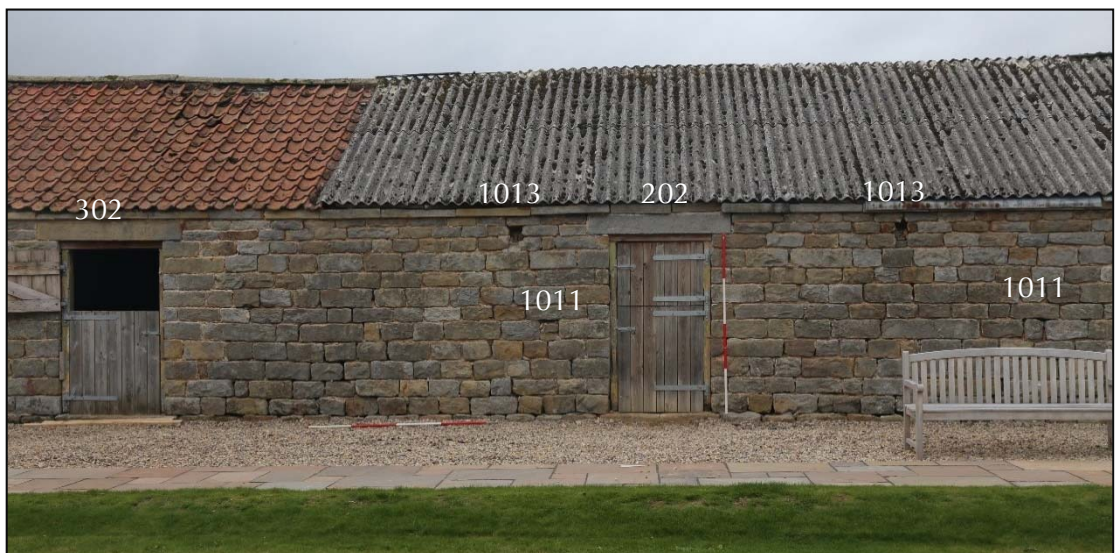
Plate 19: centre of the east elevation (1010) of the west range. Visible ventilation holes (1013) flank door 202.
