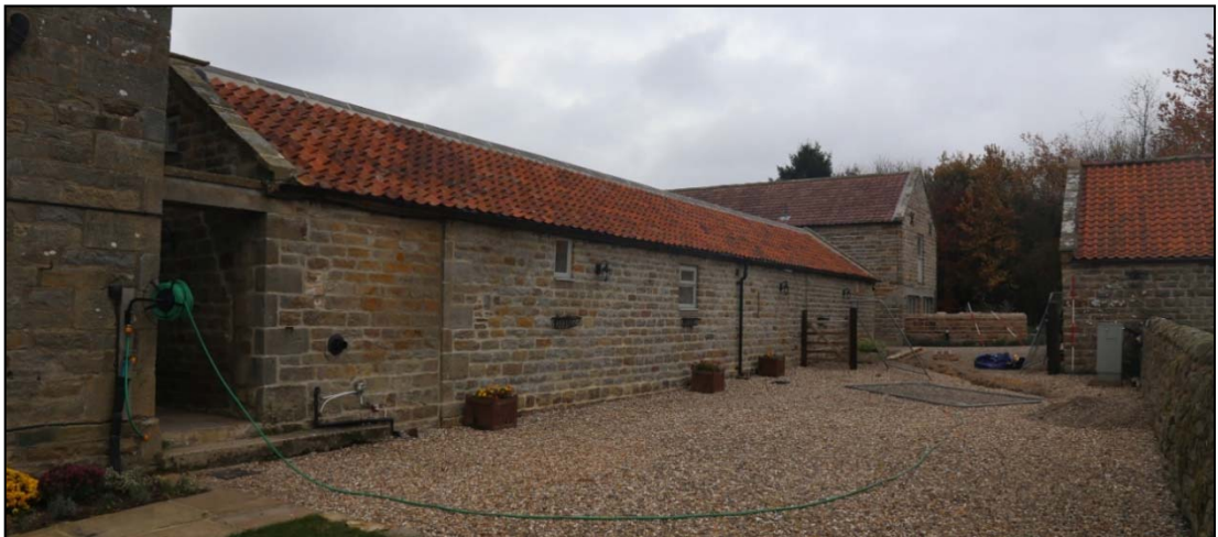
Plate 7: east elevation of the east range seen connecting to the farmhouse on the left. The southern extension of the building is visible as a wall scar and variation in build at the south end of the range (nearest the farmhouse). On the right of the picture the west end of the cart shed is just visible.
