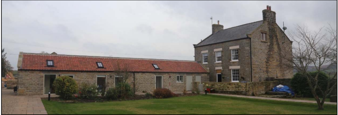
Plate 6: west elevation of the east range, looking east, with the north elevation (rear) of the farmhouse directly to the south.
