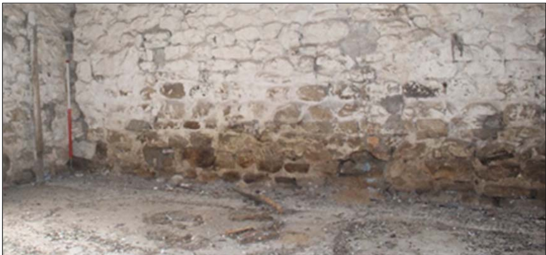
Plates 29 and 30: photograph taken during the earlier survey showing (top) in-situ brick feeding trough lining the north wall, looking north-west and (bottom) the scar in the floor showing the former location of a wooden feeding trough along the south wall, looking south-east, note the timber upright (205) to the left. (Photos by CS Archaeology 2018).
