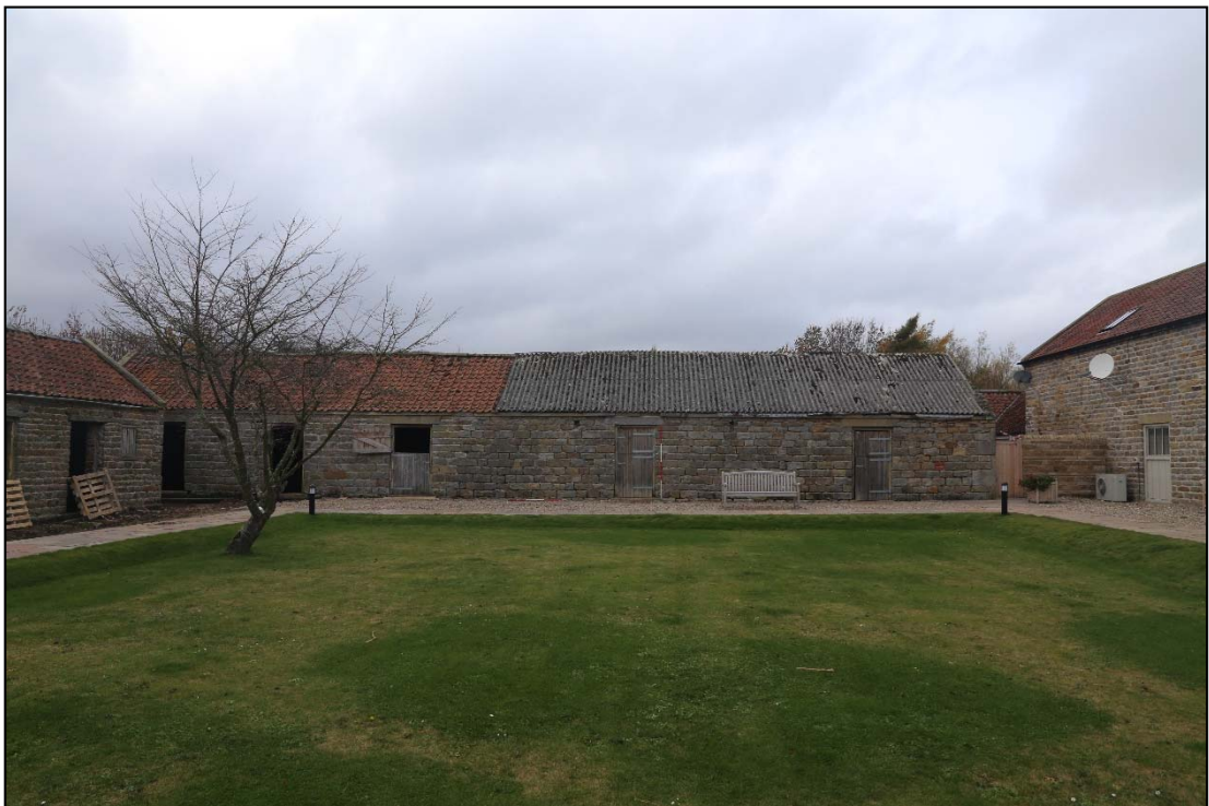
Plate 15: east facing elevation (1010) of the west range overlooking the central foldyard viewed from the east range looking west.
