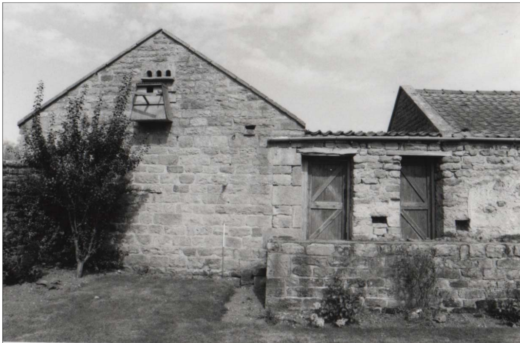
Plate 20: south elevation of the west range. The dovecot sits near the top of the gable. Photo also shows structure 2700. (Photo by CS Archaeology 2018).
