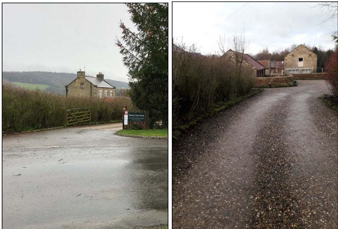
Plates 1 and 2: (left) access to Thirley Cotes is from the east along Waite Lane onto an access road (right) on the north-east side of the farmstead.
