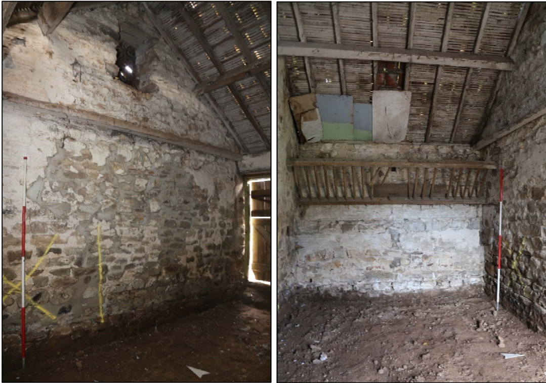
Plates 36 and 37: (left) oblique view looking north-east along the north wall, room 400 (loose-box). The former floor beam is clearly visible, as well as window (405) set below the apex; and (right) looking west towards the hay rack (402) and trough remain (403).
