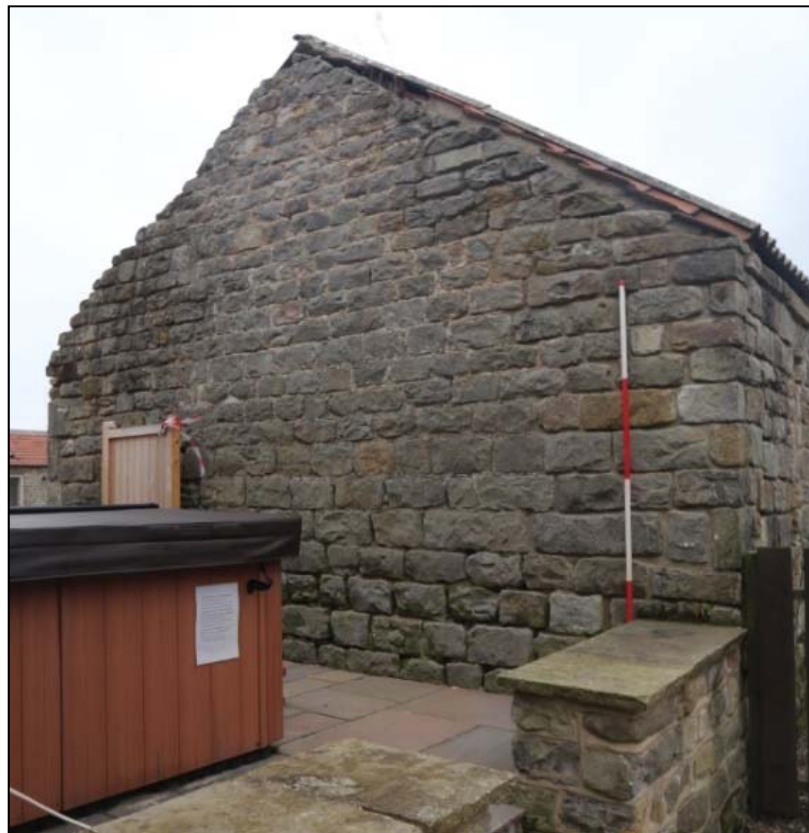
Plate 24: north elevation (1400) of the west range looking south-east.
