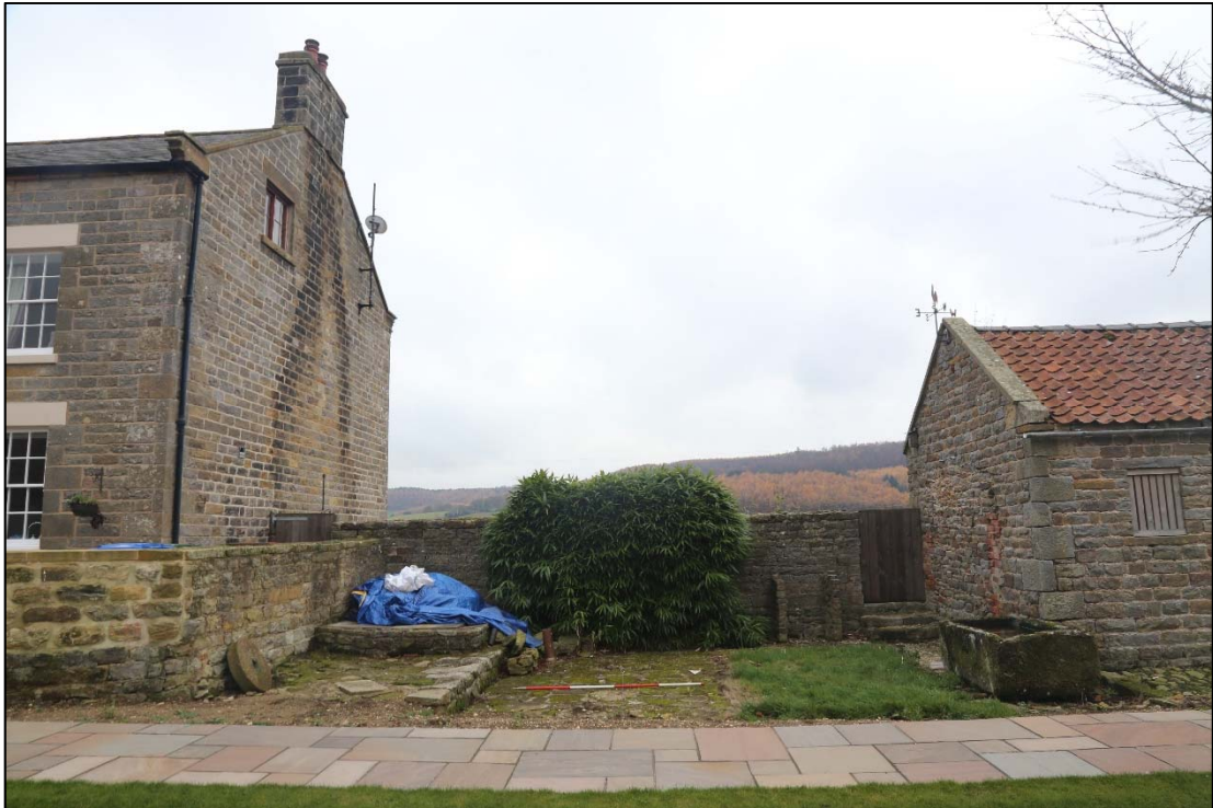
Plate 61: building footings between the south range and farmhouse associated with the south range extension. This building may have originally served as an implement shed or pigsty.
