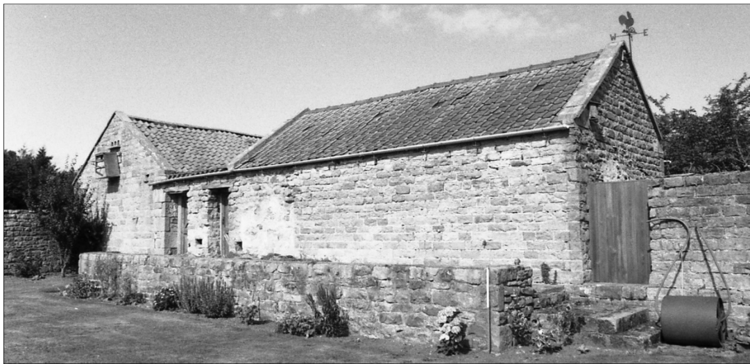
Plate 45: former greenhouse (2700) built against the southern wall of the south range (2000). This structure served as a greenhouse during its final phase of use, the associated wall (2704) can be seen standing 1.00m high at the time of the CS Archaeology survey. (Photo by CS Archaeology 2018).
