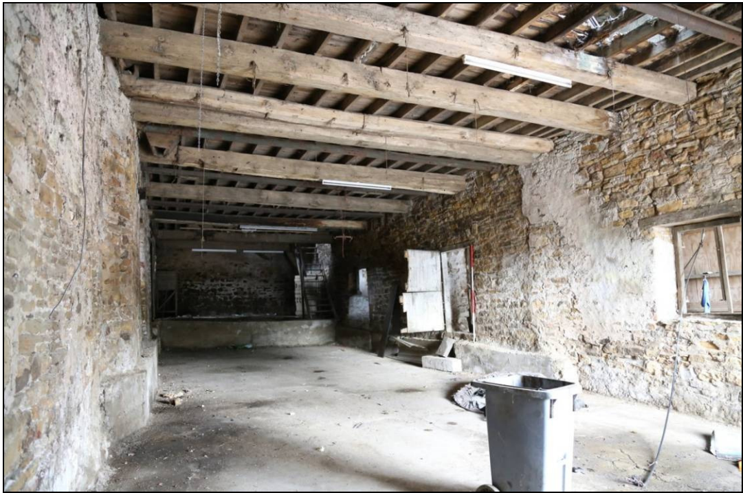
Plate 12: the interior of the Granary looking north-east, showing the change in wall thickness towards the earlier part of the building and the paired beams supporting the loft above
