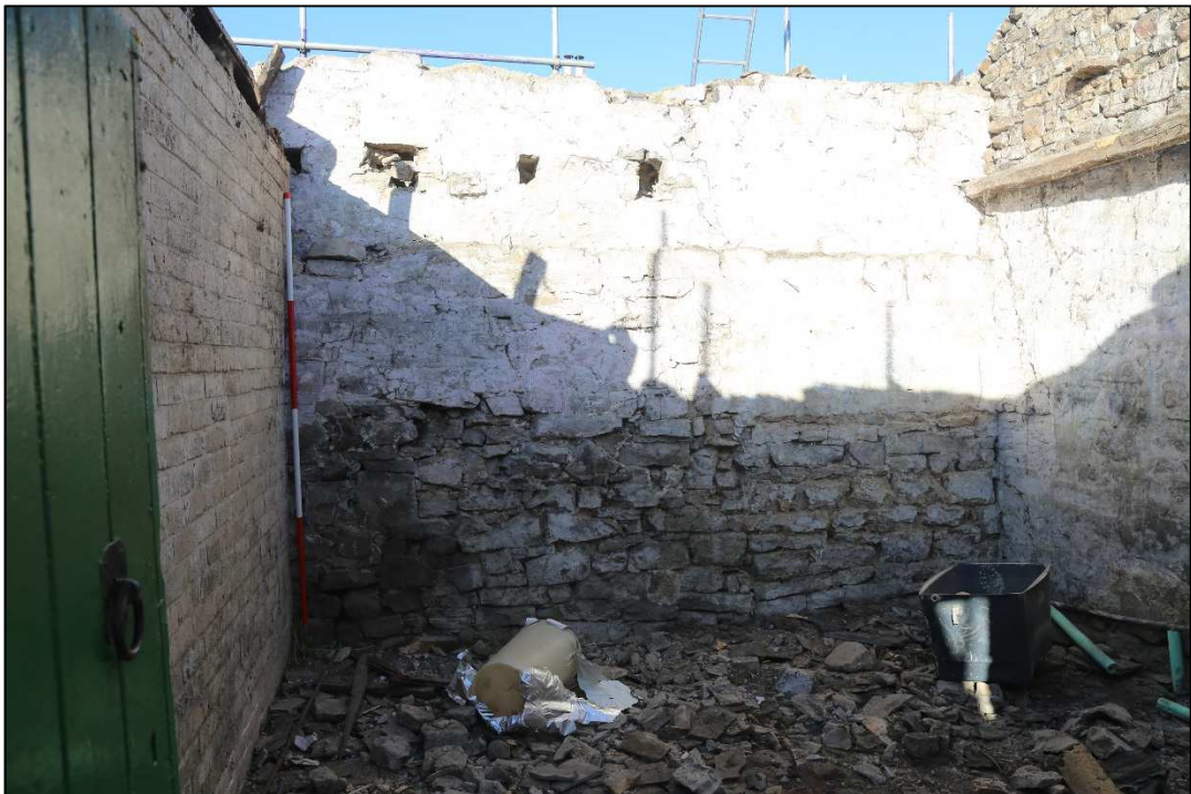
Plate 15: Rear wall of the store room showing early wall and infilled doorway
