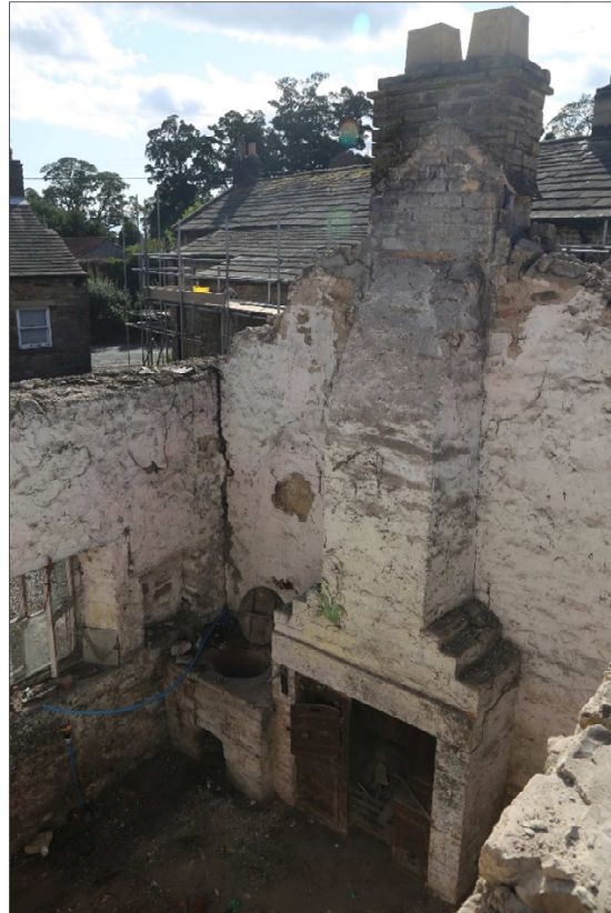
Plate 12: The chimney stack, range and copper in the 'kitchen' room.
