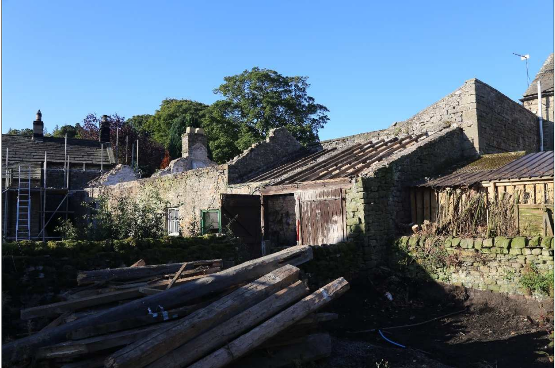
Plate 6: Front elevation of the outbuilding from the north-east
