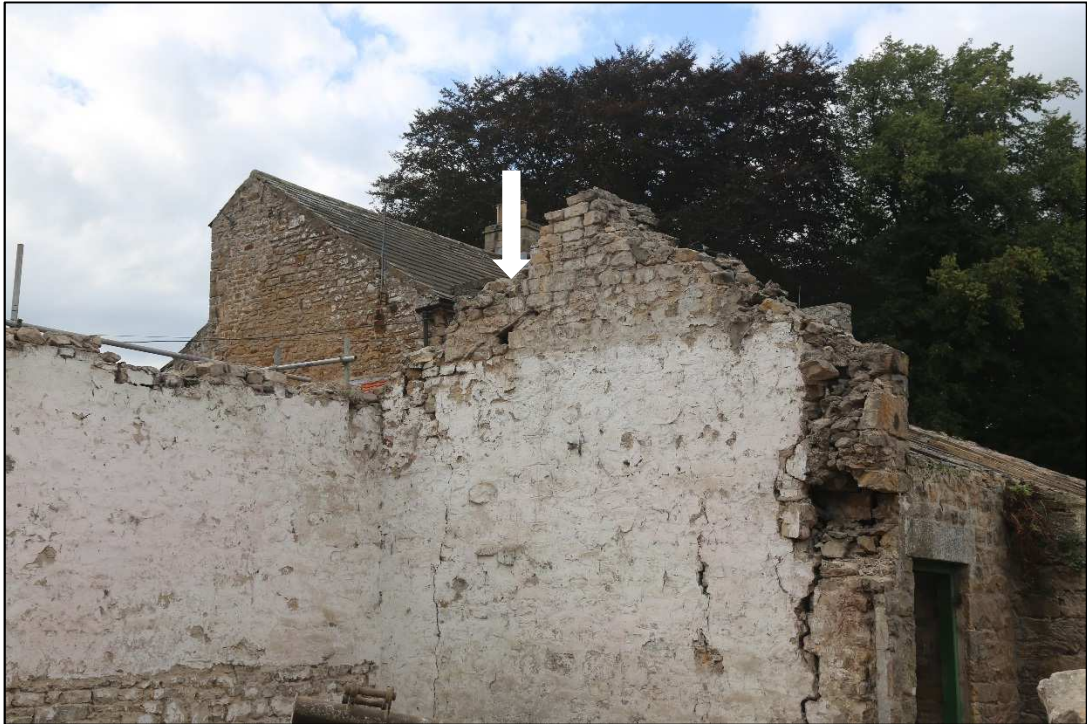
Plate 19: The southern wall of the coal store showing the sloping remnant of an early roof
