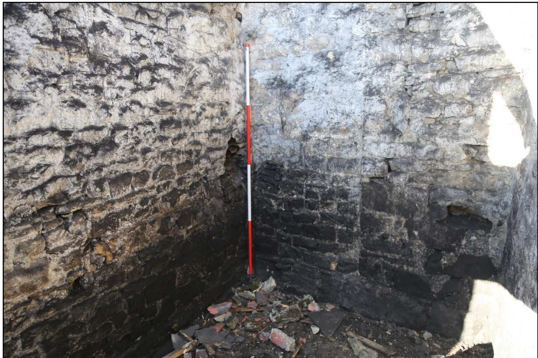
Plate 17: blocked entrance in the rear wall of the coal store
