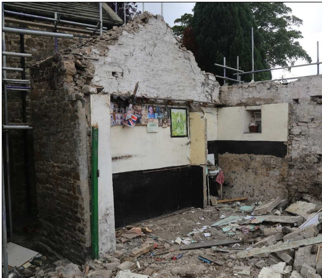
Plate 16: The gent's toilet partly demolished showing plaster facing and partition wall
