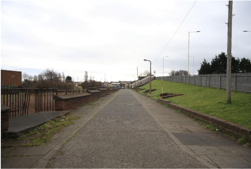
Plate 21: walkway allowing access to Moreton Station, facing south.
