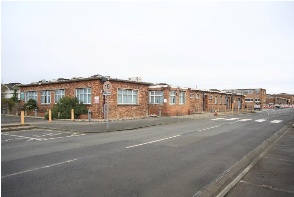
Plate 11: Block F: facing north-east.
