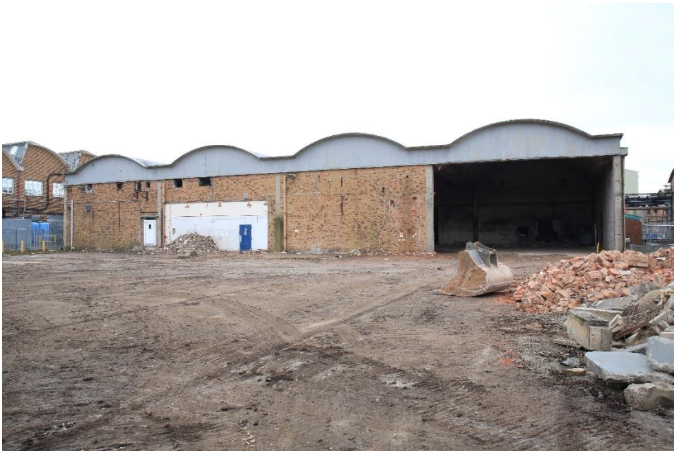
Plate 16: Block G3: north side, facing south.
