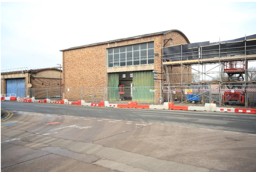
Plate 14: Block G2: south side, facing north-west.
