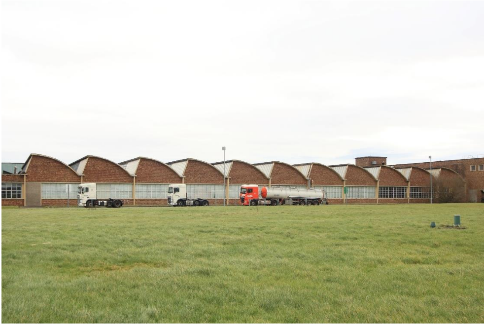
Plate 1: Block A: saw-tooth roof, west elevation facing east.
