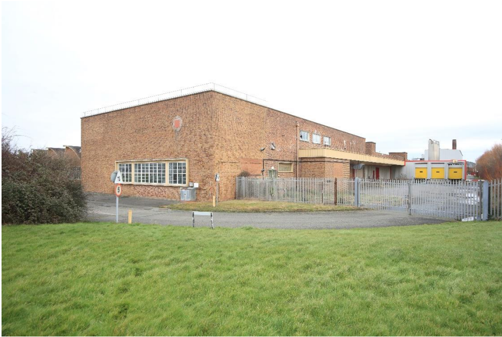
Plate 3: Block A: flat-roofed block with loading bay.
