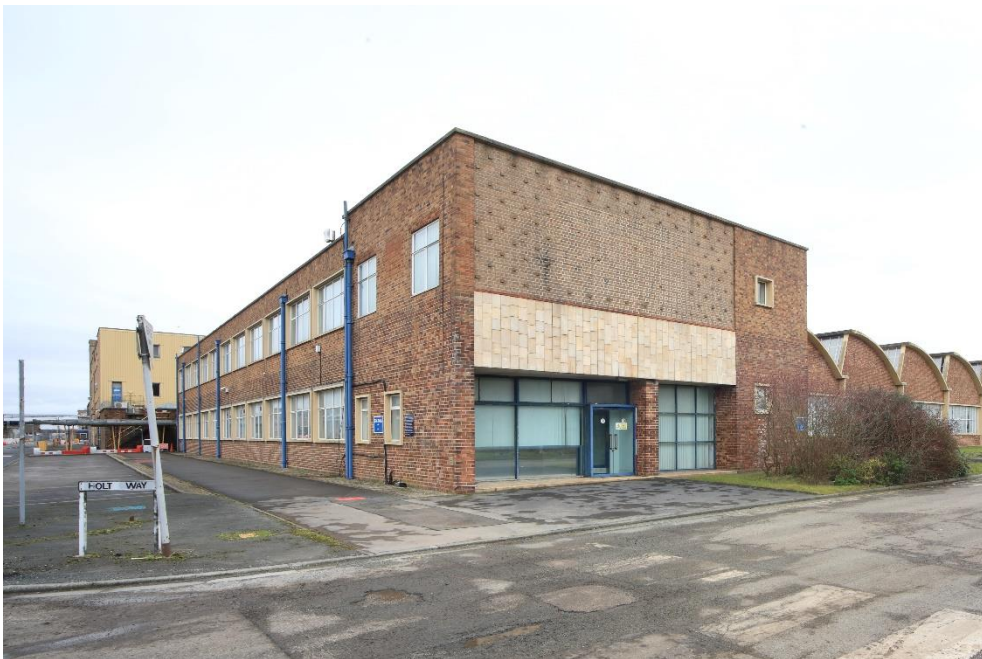
Plate 2: Block A: flat-roofed office block, facing south-east.
