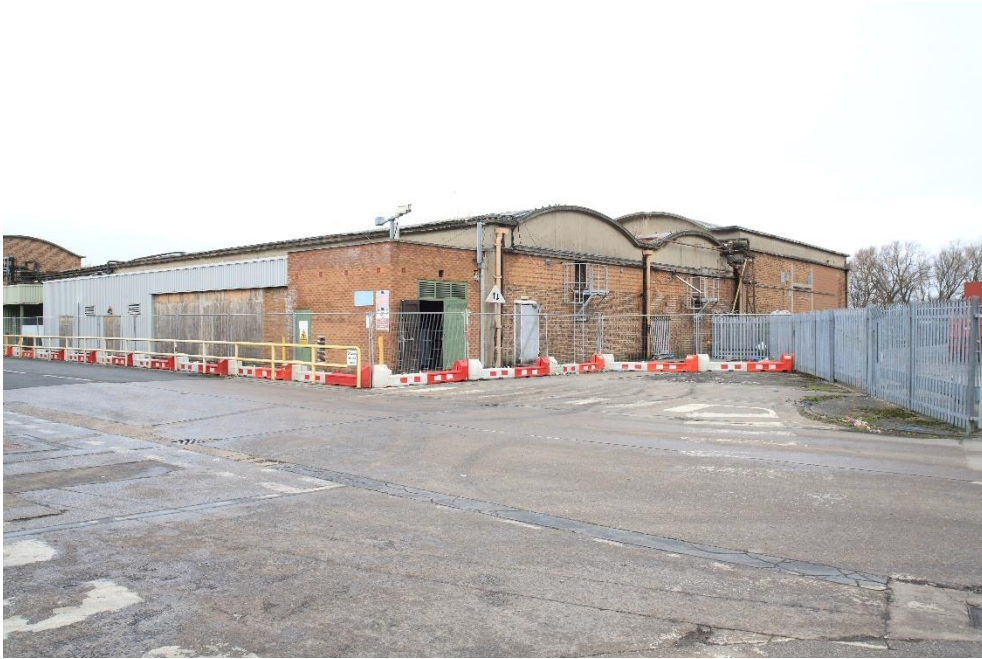
Plate 17: Block G3: south-east corner, facing north-west.
