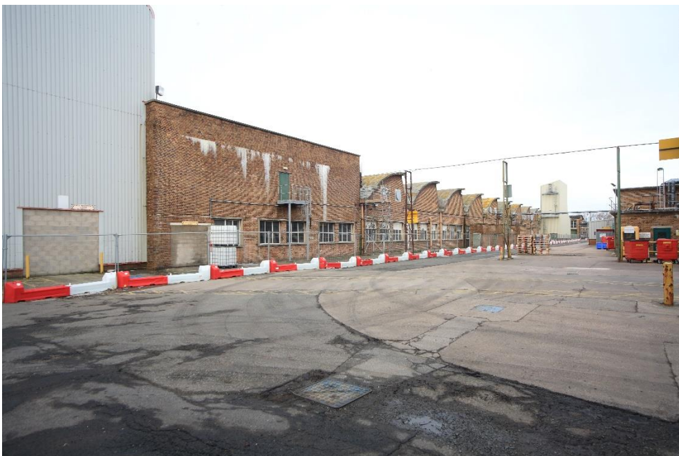
Plate 10: Block C; south-east corner, facing north-west.
