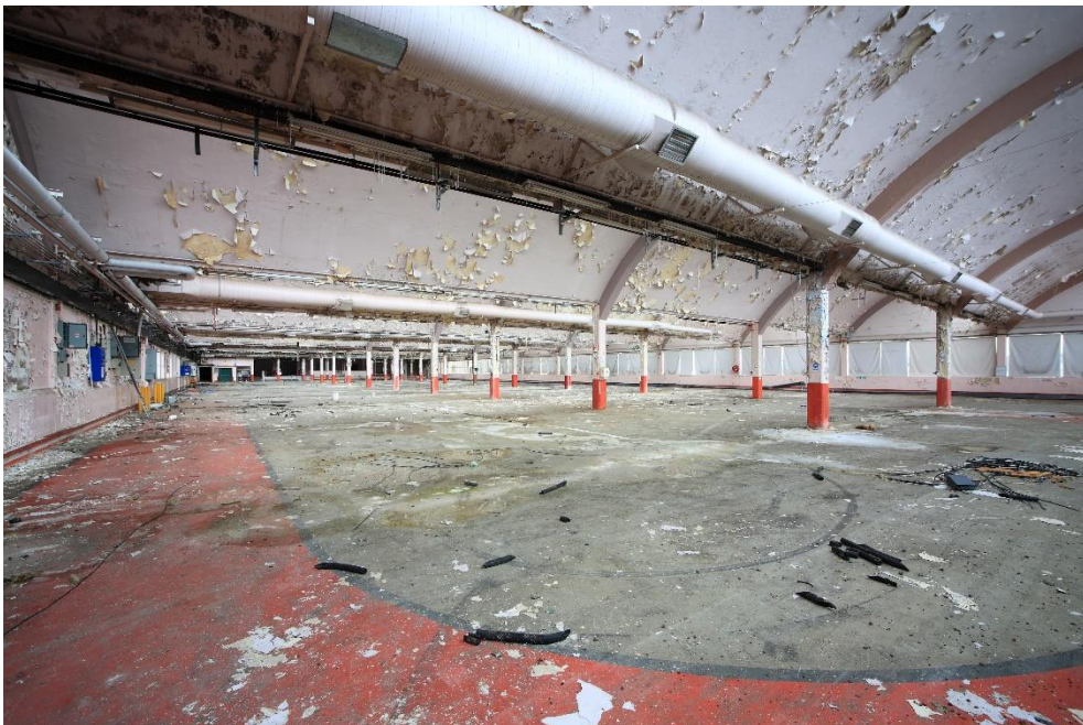
Plate 4: Block A: interior view, facing south-west.
