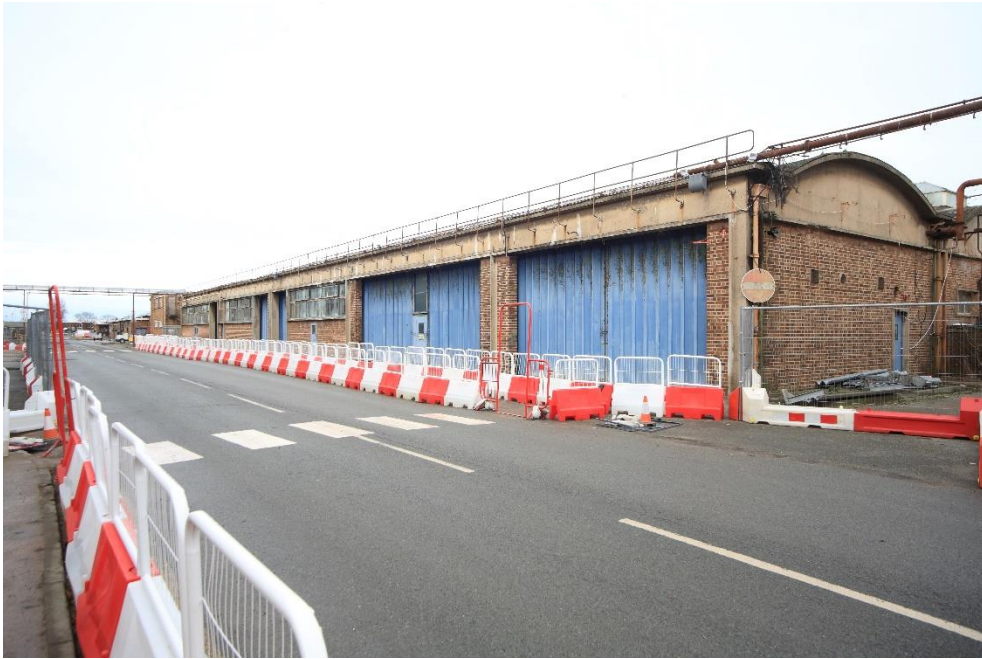
Plate 13: Block G1: south side, facing north-west.
