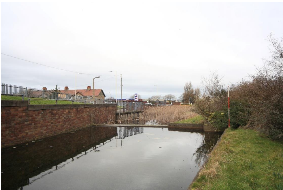
Plate 18: the 'Jellicoe Weir' (1), facing north.
