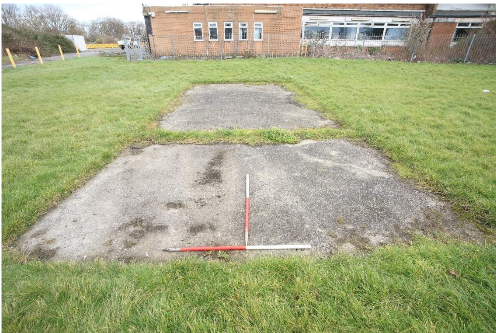
Plate 26: concrete building platform (4) to the east of Block F, facing east.
