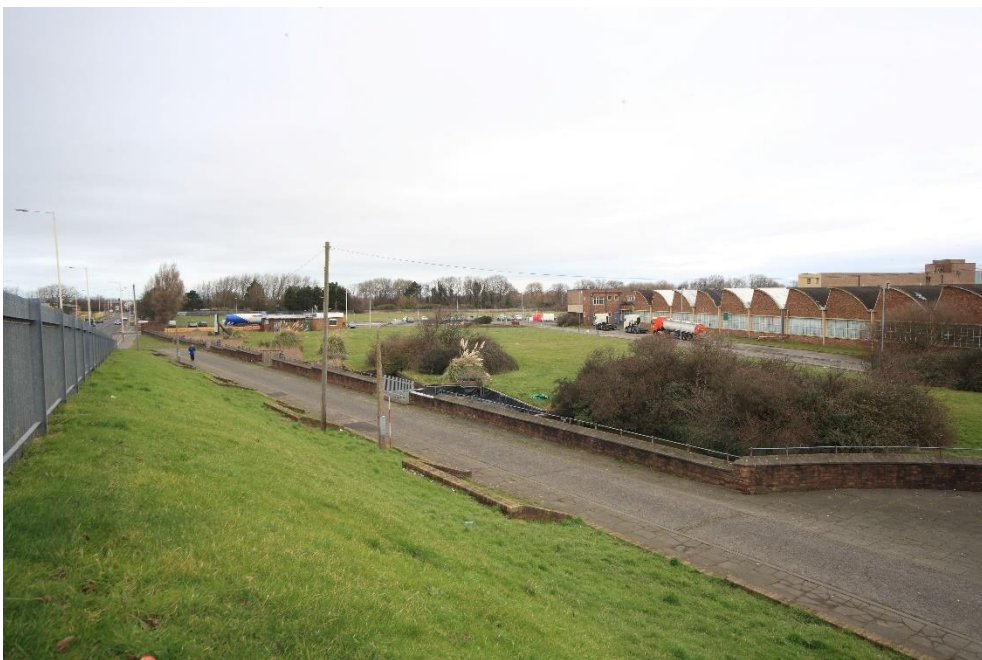
Plate 20: the 'Jellicoe Weir' (1), facing north.
