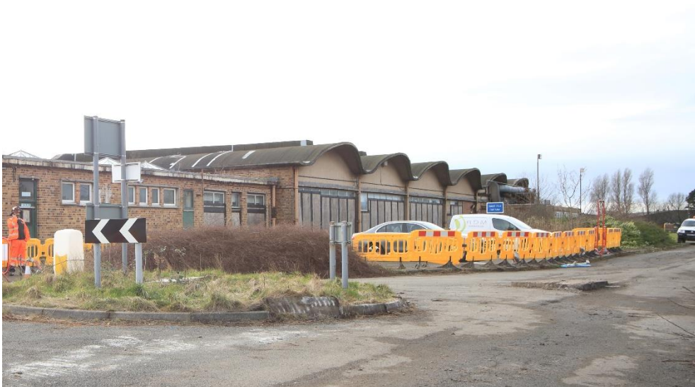
Plate 12: Block F: barrel-vaulted roofs, facing west.
