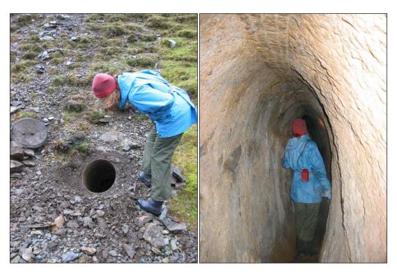
Plate 29: entrance to the coffin level (left) and inside the level (right) (photo: Lund 2020).
