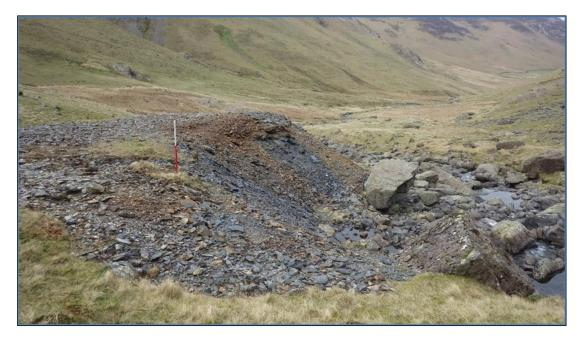
Plate 65: washed-out section of mining waste at the entrance to adit 182671. Newlands Beck is to the right.
