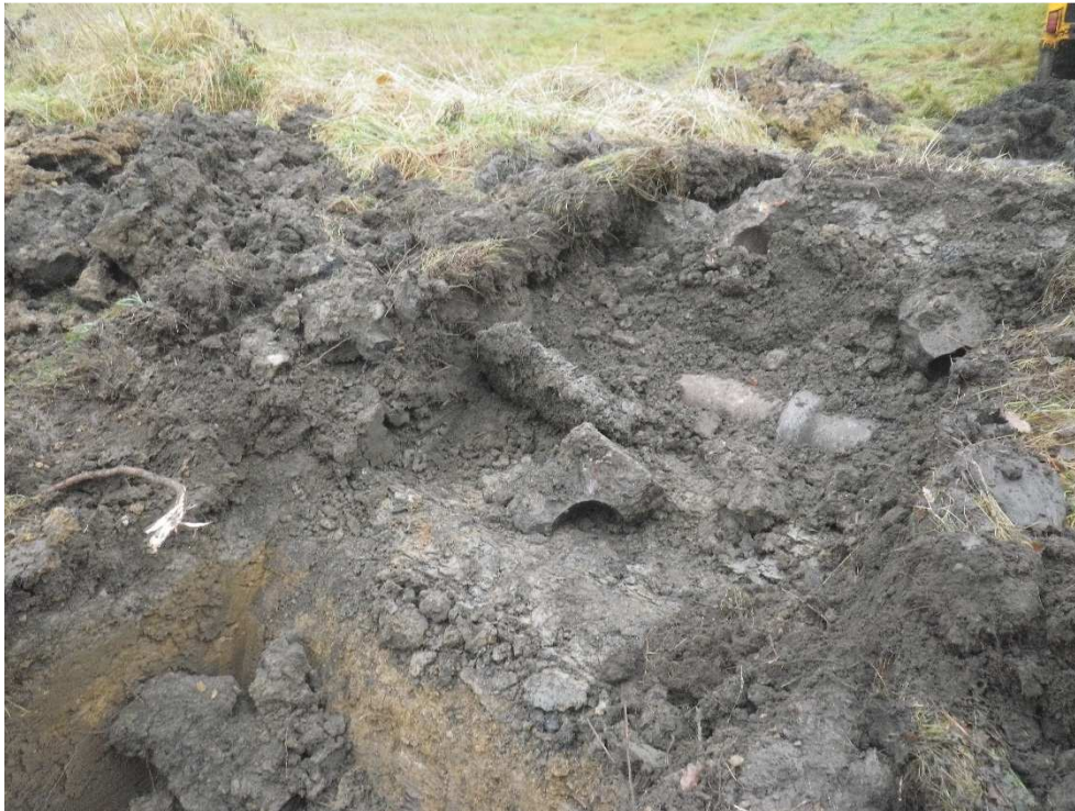
Plate 1: view of service pipe 105 in earthwork, exposed in trench 1, facing south-east.
