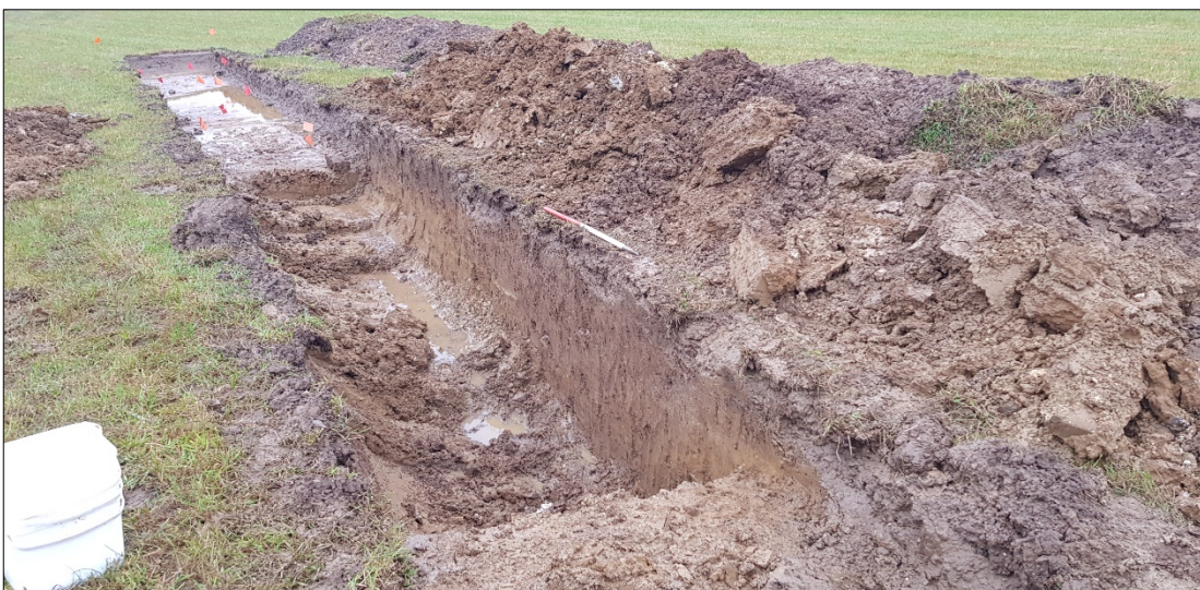
Plate 8: overview of ditch 75 within Trench 8, looking south-east (scales shown 1m).
