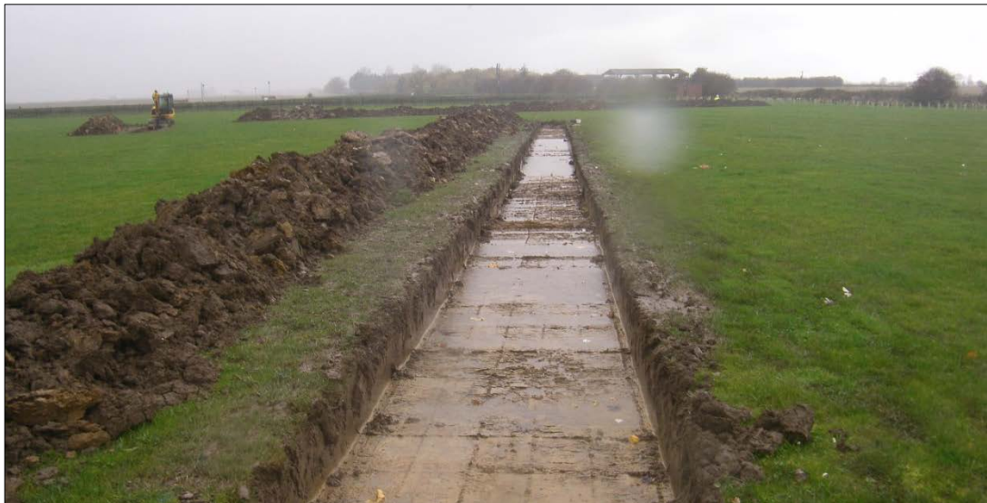
Plate 37: overview of Trench 25, looking west.
