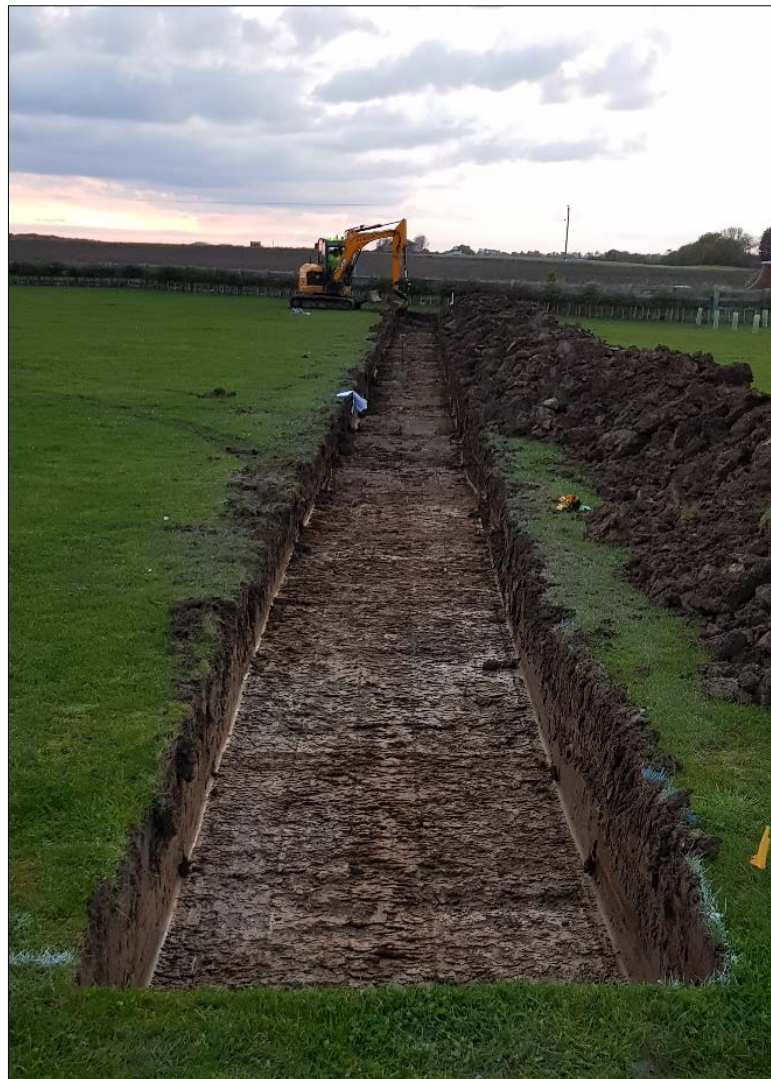
Plate 24: overview of Trench 18, looking south-west.
