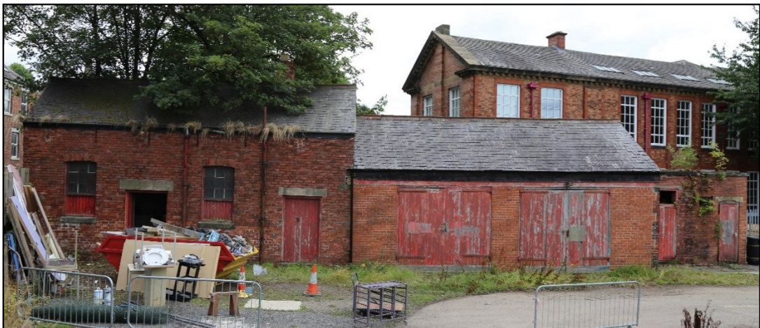
Plate 2: front elevation of the stable and cart shed associated with the former industrial laundry.
