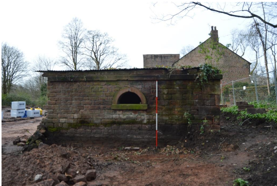
Plate 9: east elevation with Beech Cottage in the background. View looking west
