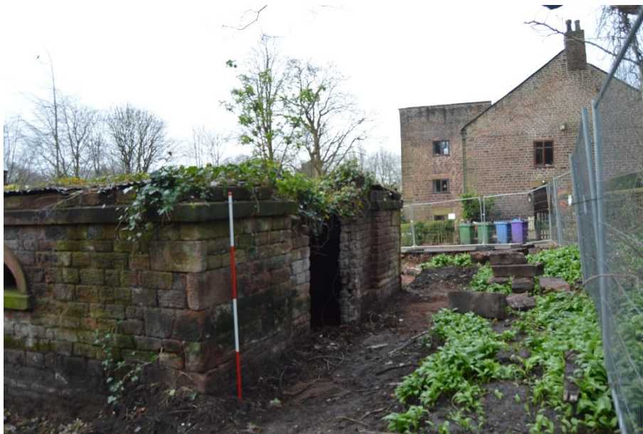
Plate 5: north elevation with Beech Cottage in background. View looking west
