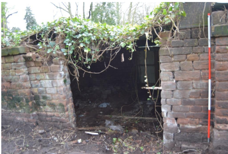
Plate 6: doorway in north elevation. View looking south
