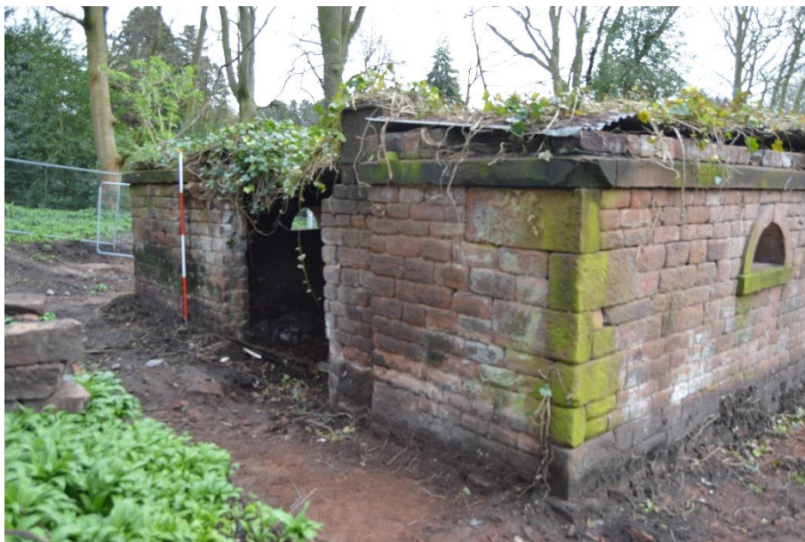
Plate 3: north elevation. View looking south-east (scale = 2m)
