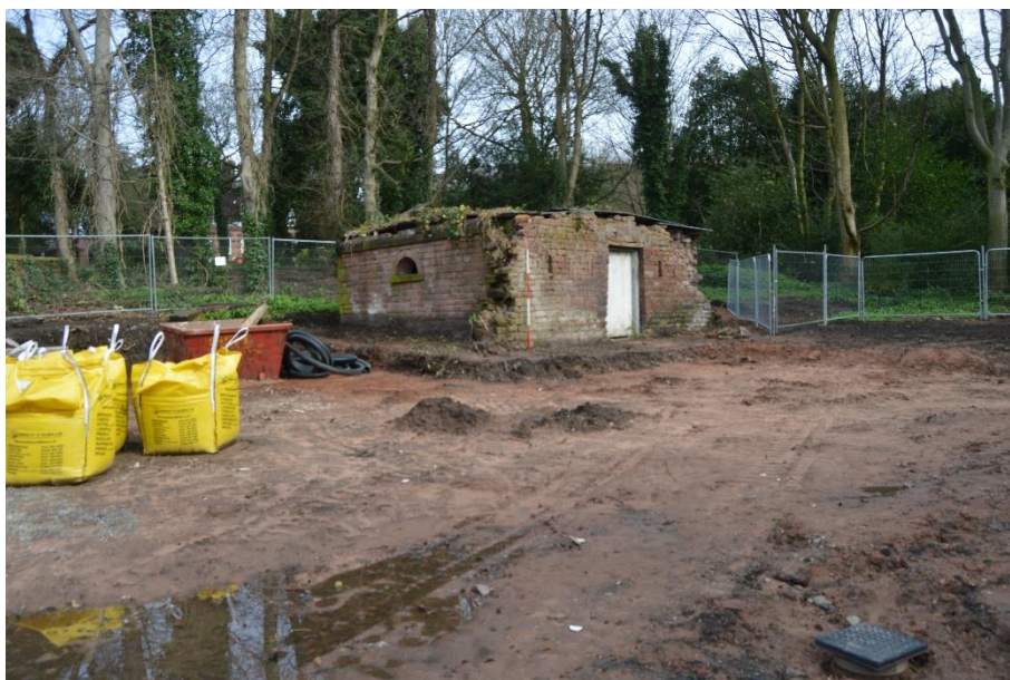
Plate 19: view looking north-east showing groundworks undertaken from driveway
