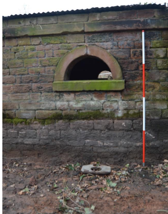
Plate 10: detail of lunette window, east elevation. View looking west
