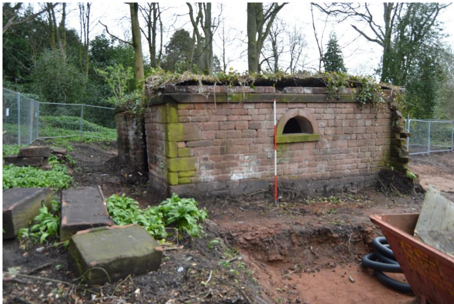
Plate 17: west elevation. View looking east (scale = 2m)
