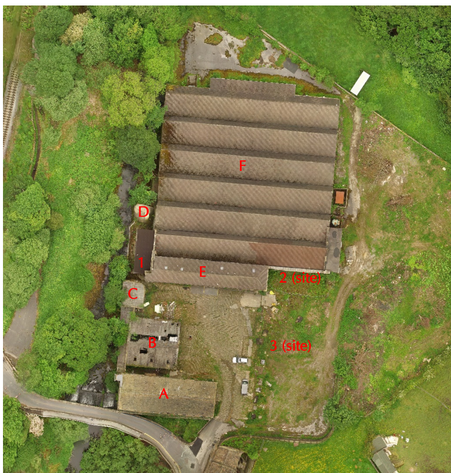
Plate 2: Layout of Ebor Mills with building numbers highlighted (north is at the top of the image)
