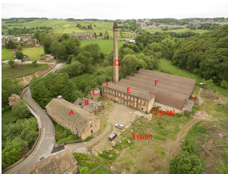
Plate 1: Ebor mills, facing north-west with building numbers highlighted
