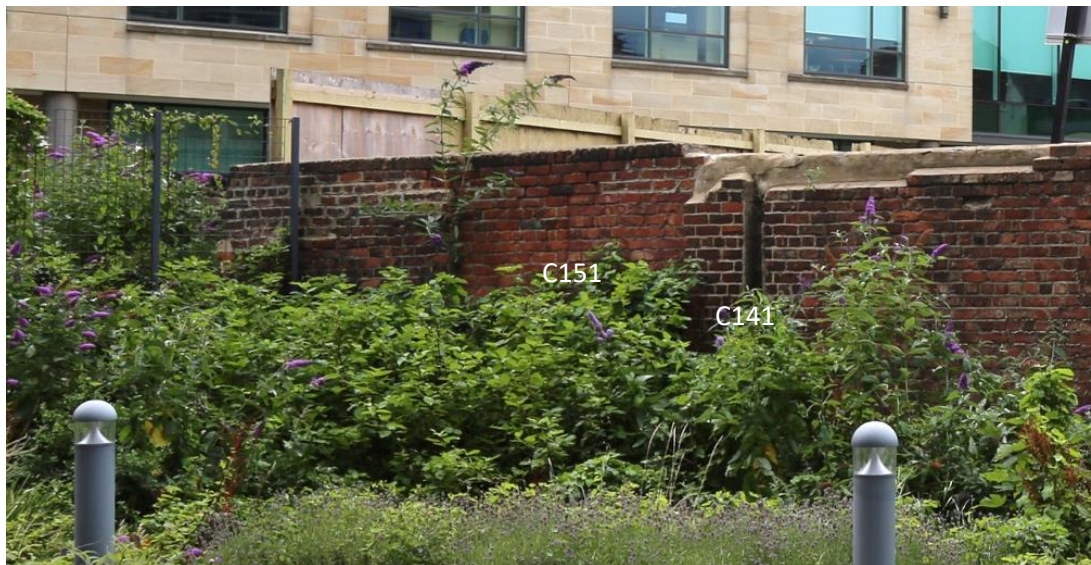
Plate 7: The rear of wall C100. The scar C151 is visible extending down into the foliage. It is located just south of the groove C141.
