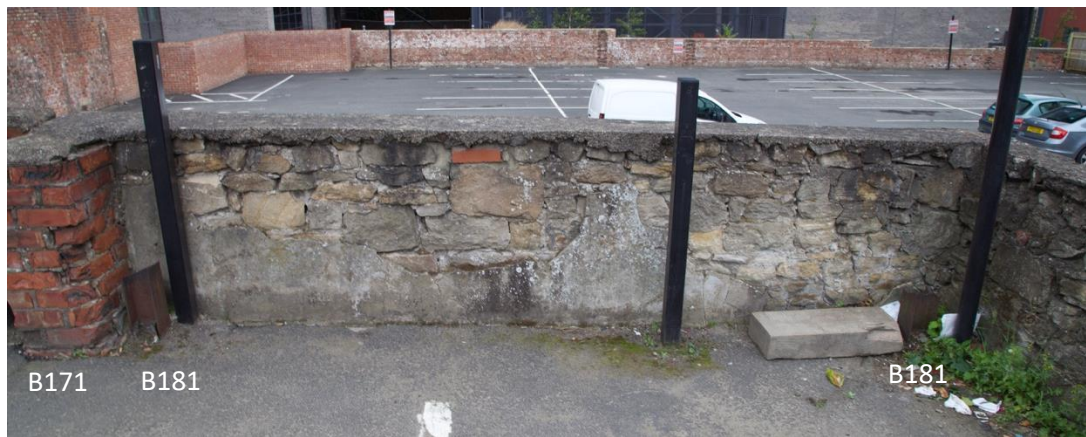
Plate 5: Wall elevation B180 looking east. The wall plinth B171 is visible on the left along with the iron beams, B181 , on either side of wall B180 .
