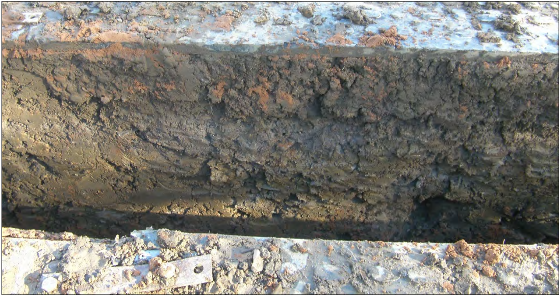
Plate 7: West-facing section of 121, potential return of gully 39.
