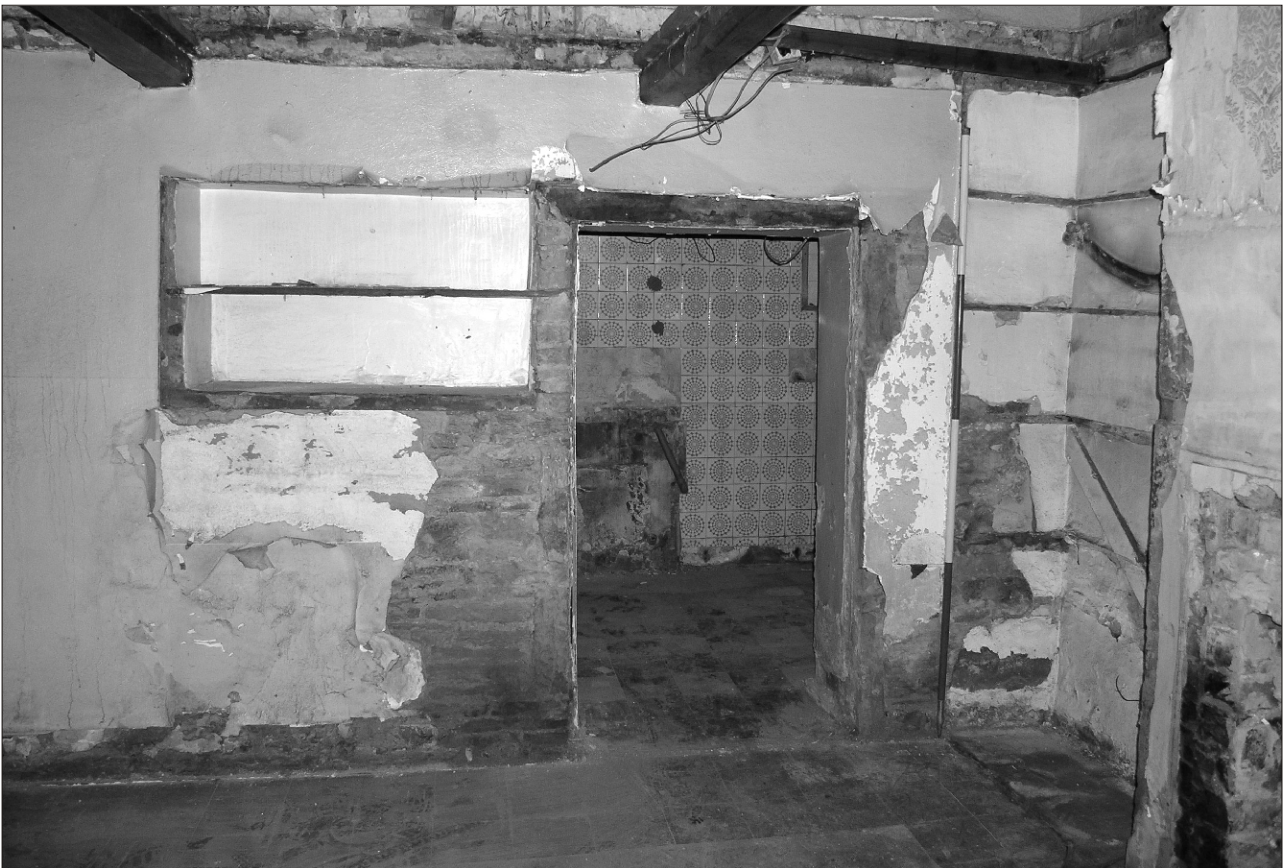
Plate 4 Lane Head Farm South, Capitol Park, Barnsley: original north wall of 'cottage' showing doorway leading to outshot beyond
