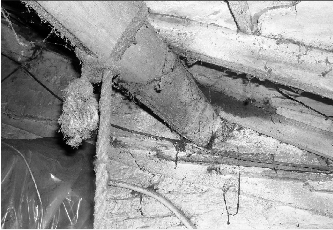
Plate 23 Lane Head Farm South, Capitol Park, Barnsley: earlier roof line visible in eastern gable of 'cottage'/outshot below later barn roof.
