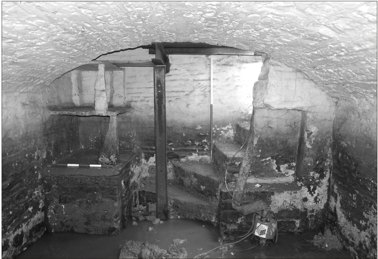
Plate 21 Lane Head Farm South, Capitol Park, Barnsley: cellar, looking north with stone shelves in northwest corner
