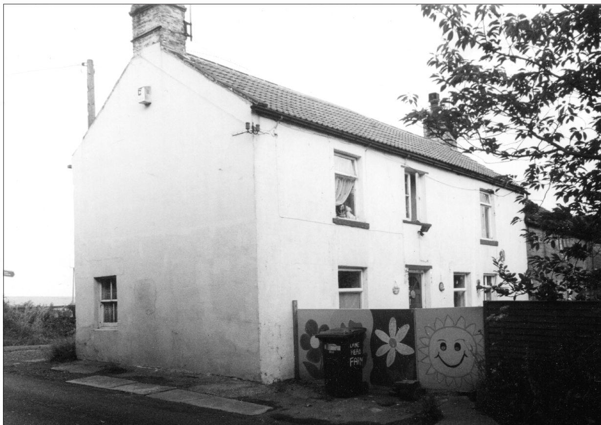
Plate 1 Lane Head Farm South, Capitol Park, Barnsley: main farmhouse before removal of render
