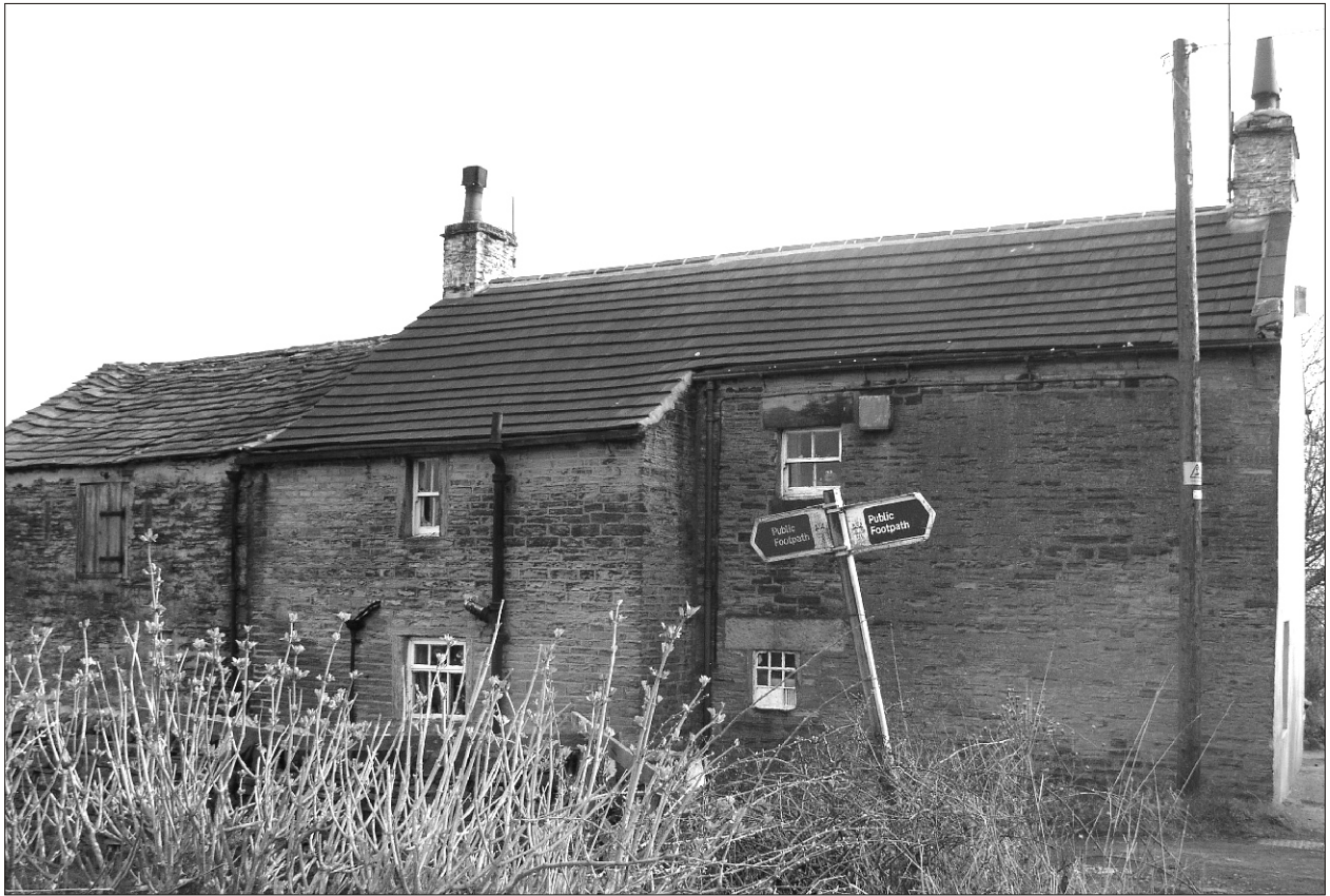
Plate 13 Lane Head Farm South, Capitol Park, Barnsley: rear of linear range showing north-facing elevation of western extension
