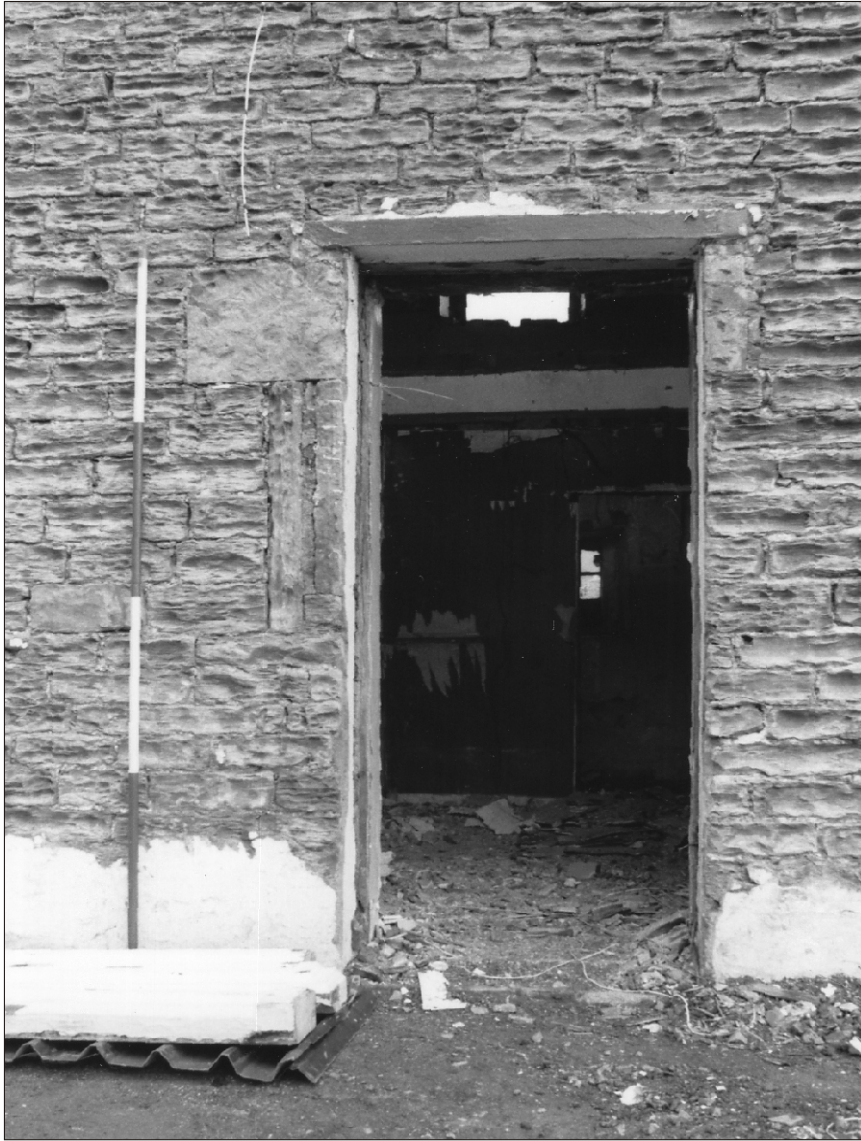
Plate 11 Lane Head Farm South, Capitol Park, Barnsley: later doorway into farmhouse with fragment of earlier window to the left
