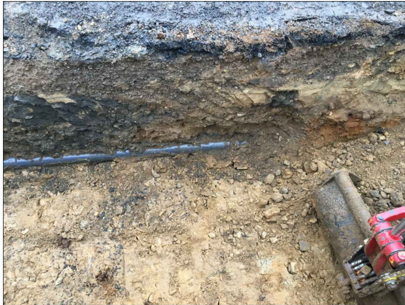
Plate 1: sample section of road trench showing depth of disturbance
