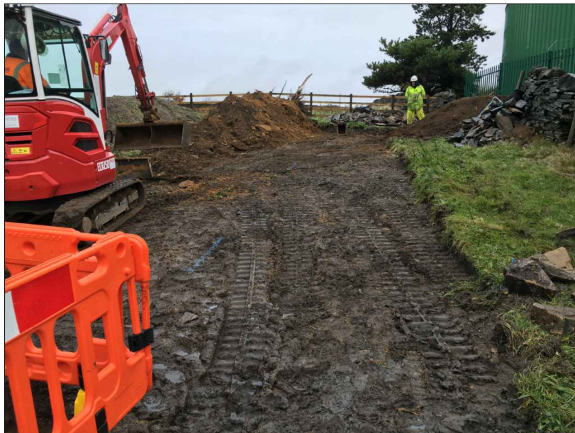
Plate 2: area in field during stripping, facing NE
