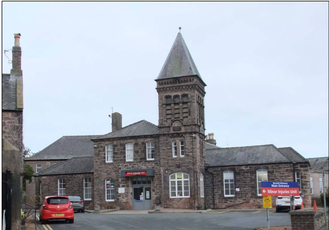
Plate 4: The original two-storey section with the attached bell tower, with single-storey wards either side.
