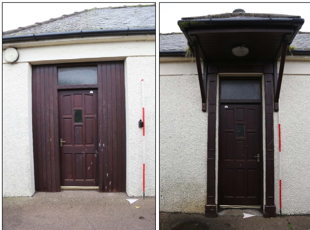
Plate 22: mortuary doors in the eastern elevation 6200.
