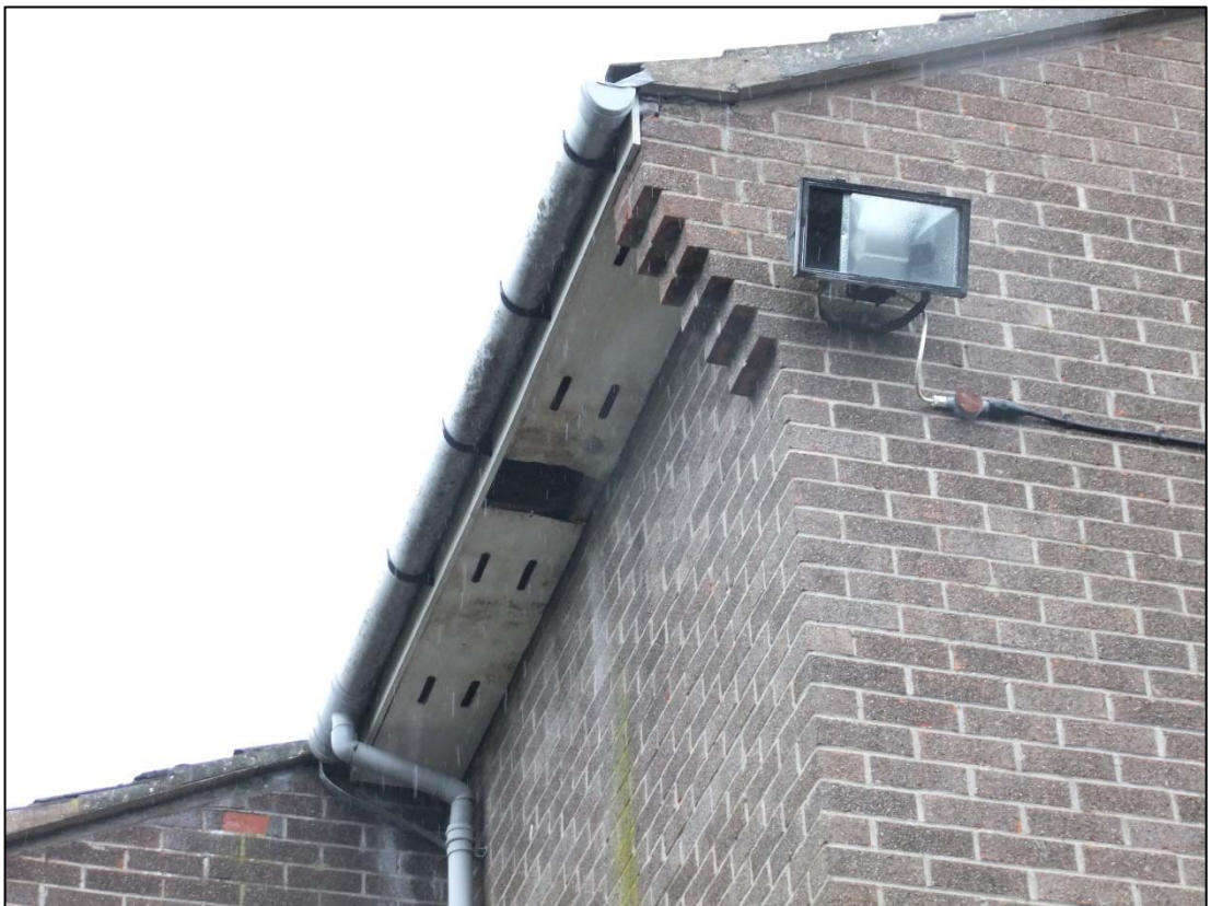
Plate 33: showing the soffits and the kneelers on the ward building.
