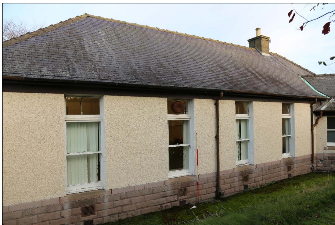
Plate 16: southwest-facing elevation showing the original windows within the main part of the Jane Richardson Ward – elevation 1130.
