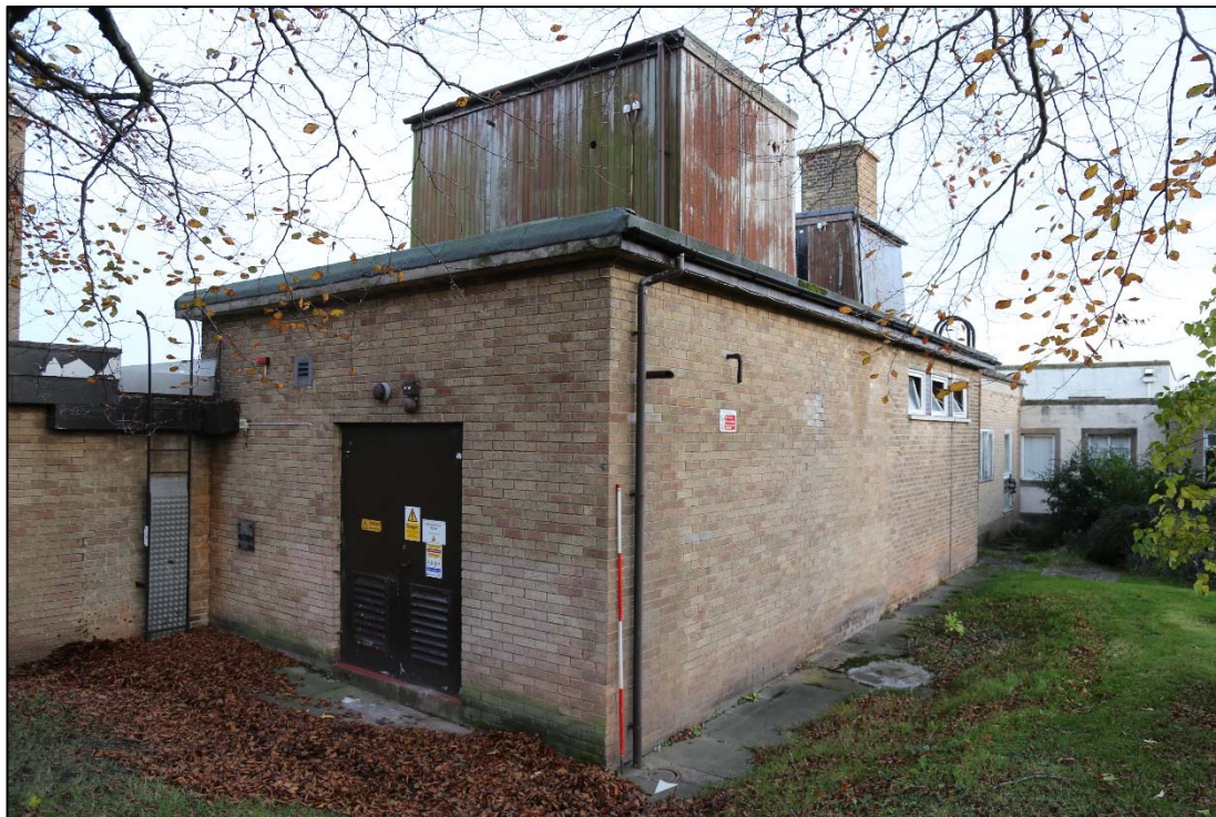
Plate 27: vacuum-plant room (2500 and 2600) with water tanks on top.
