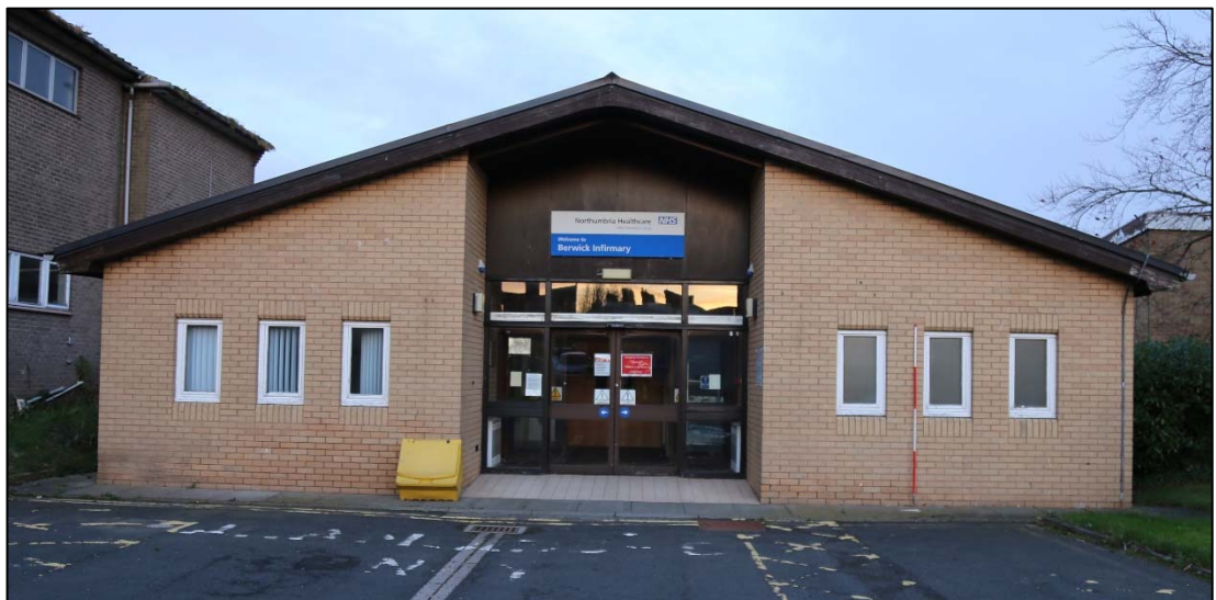
Plate 30: the main entrance 3180 showing the recessed doors.
