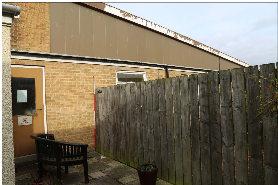
Plate 25: part of elevation 2700 showing the sloping roof.
