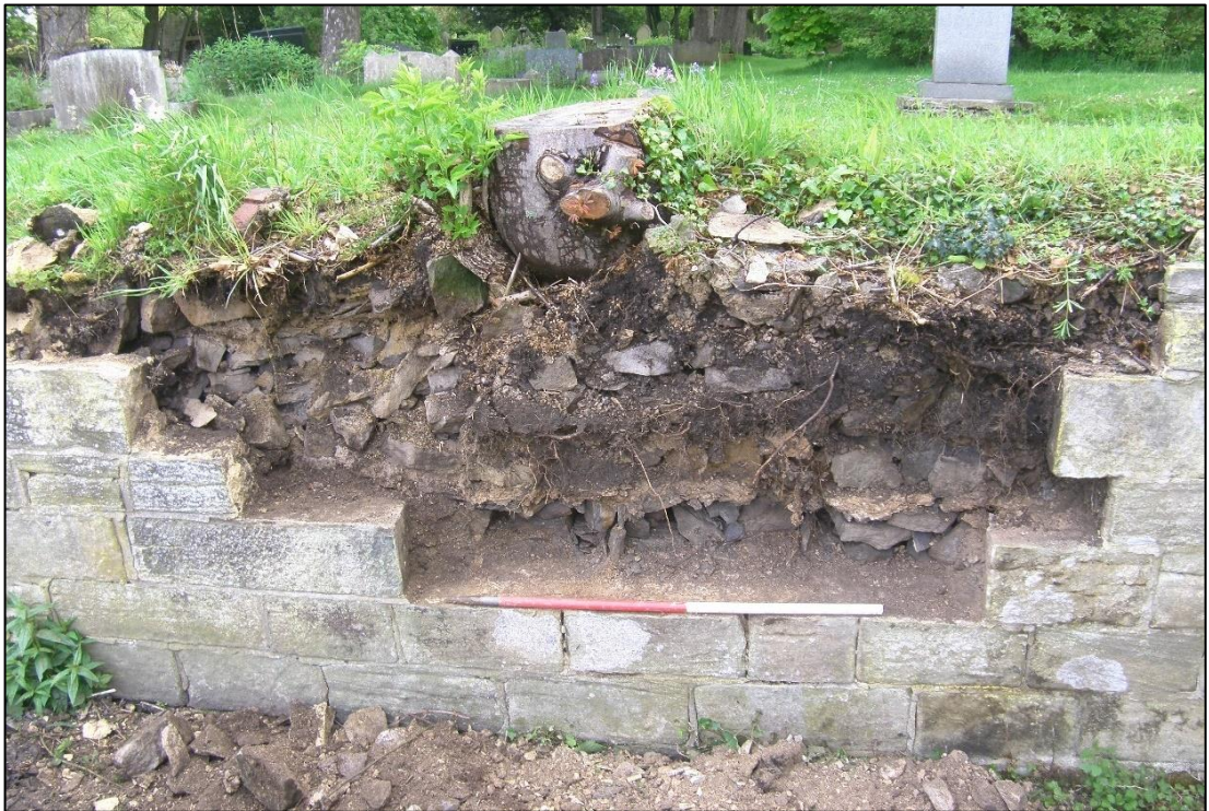
Plate 24: Section 3 of the west ha-ha after removal of the ashlar facing.
