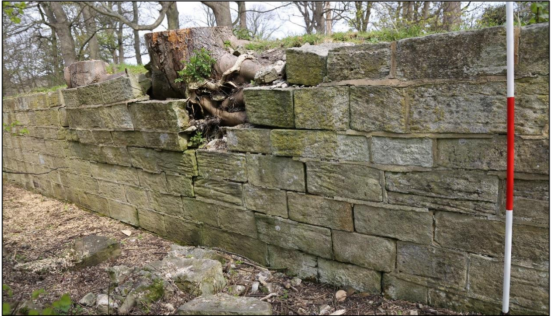
Plate 21: pre-intervention photograph of Section 2.
