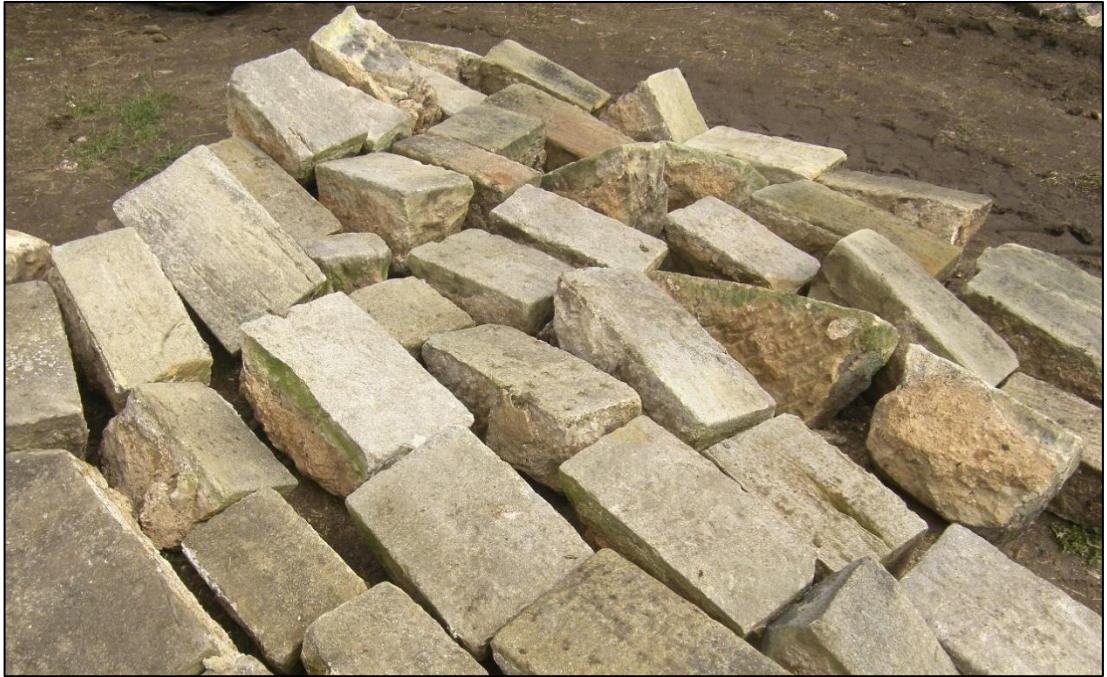
Plate 7: south-west bastion ashlar, stored in courses and displaying trapezoidal form of blocks with roughly tooled rear faces.
