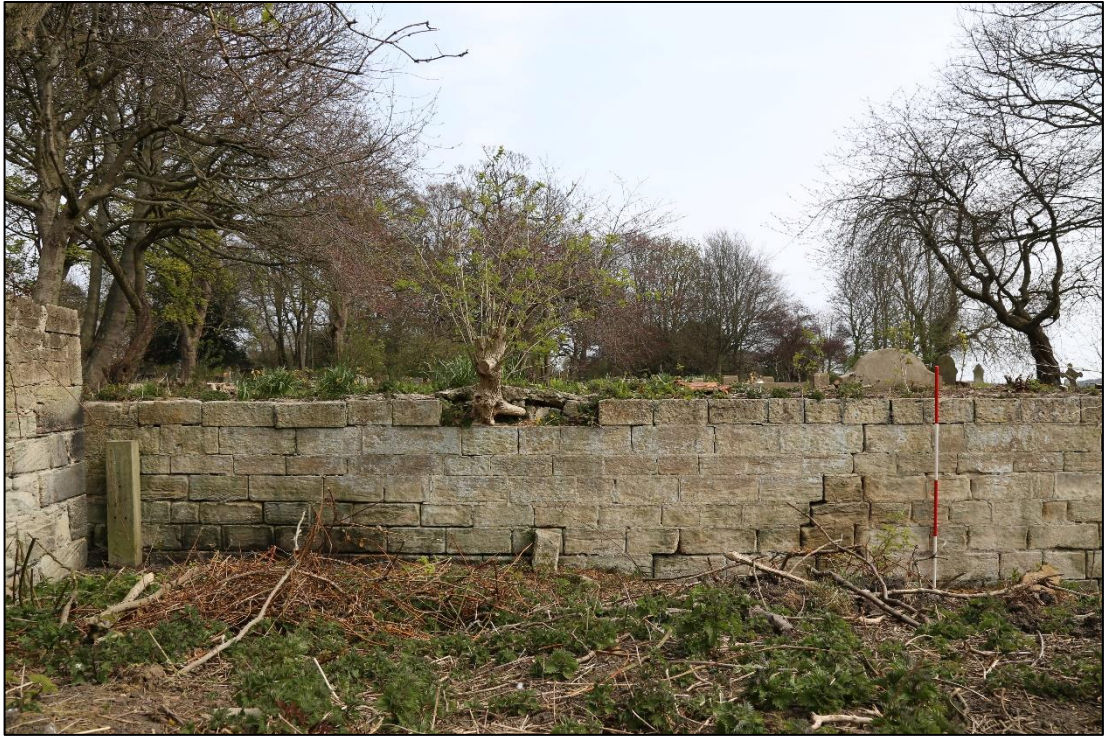
Plate 28: pre-intervention photograph of Section 5.
