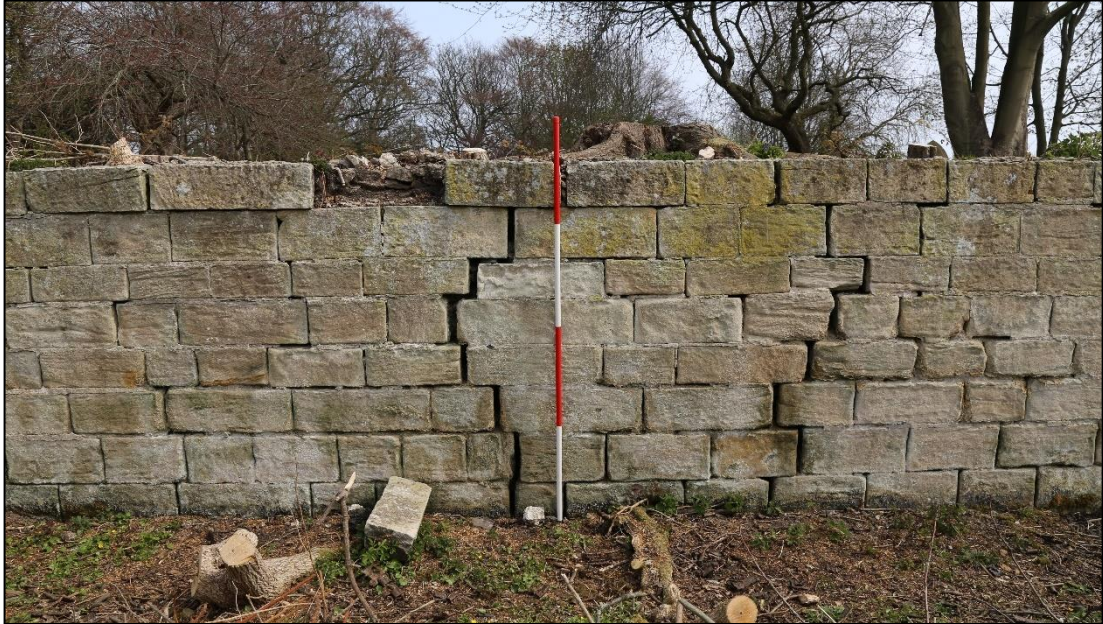
Plate 30: pre-intervention photograph of Section 6.
