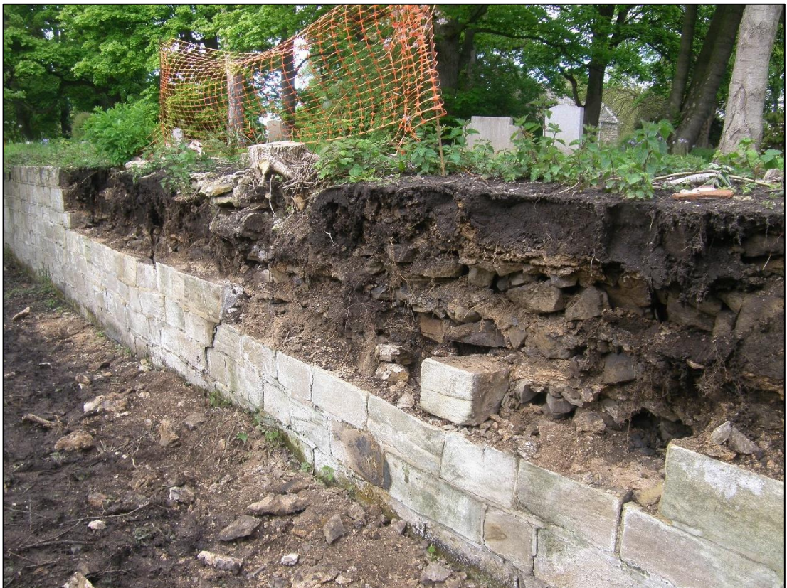
Plate 26: Section 4 of the west ha-ha after removal of the ashlar facing.
