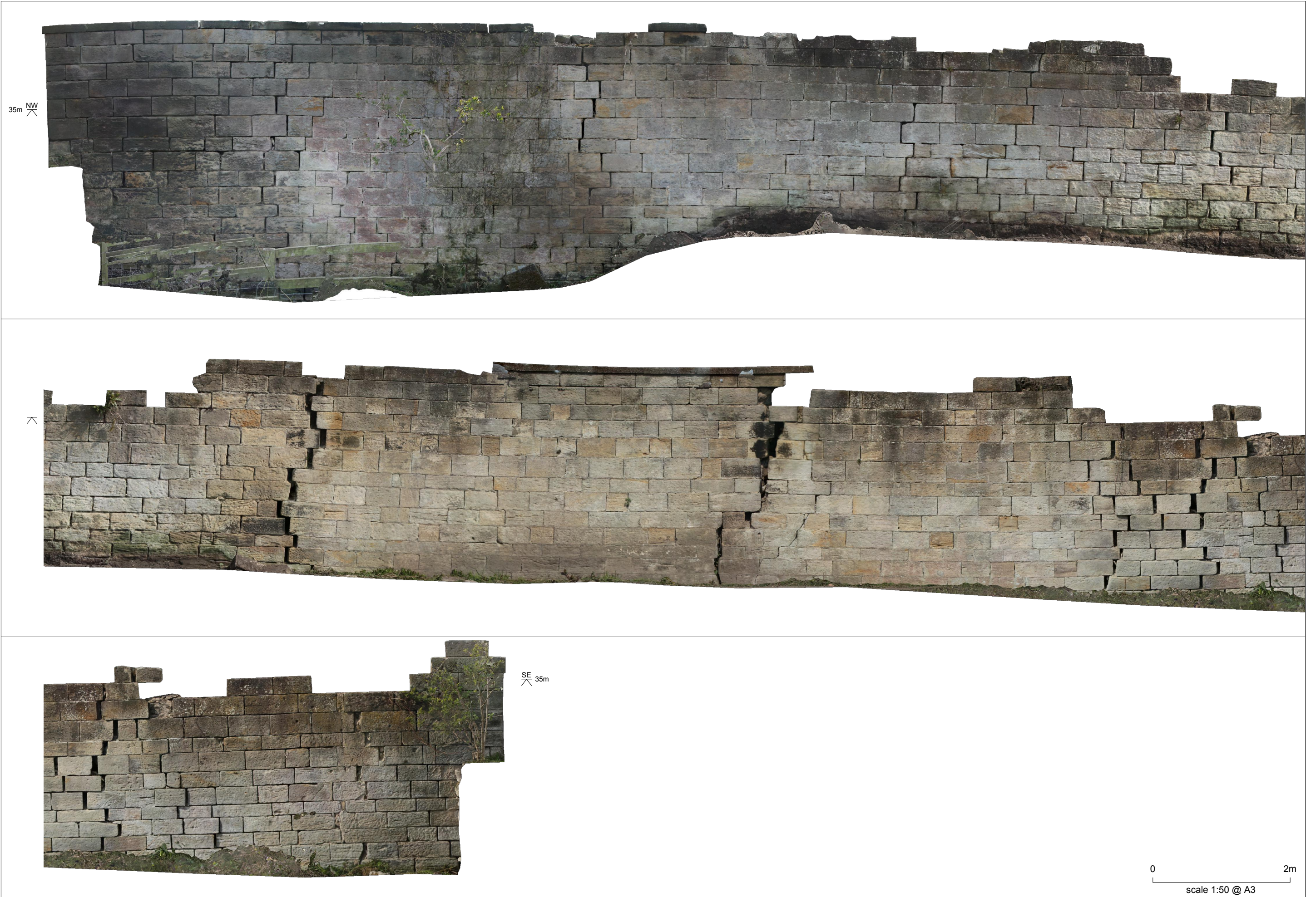
Church of Our Lady, Seaton Delaval: pre-intervention survey, south-west bastion external elevation
