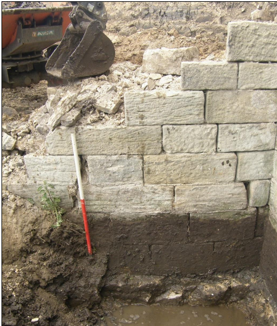
Plate 9: external foundation of the south-west bastion and southern ha-ha at the base of ditch 15.
