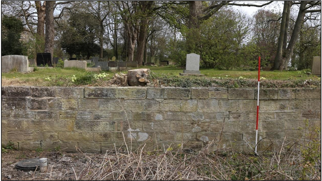
Plate 23: pre-intervention photograph of Section 3.
