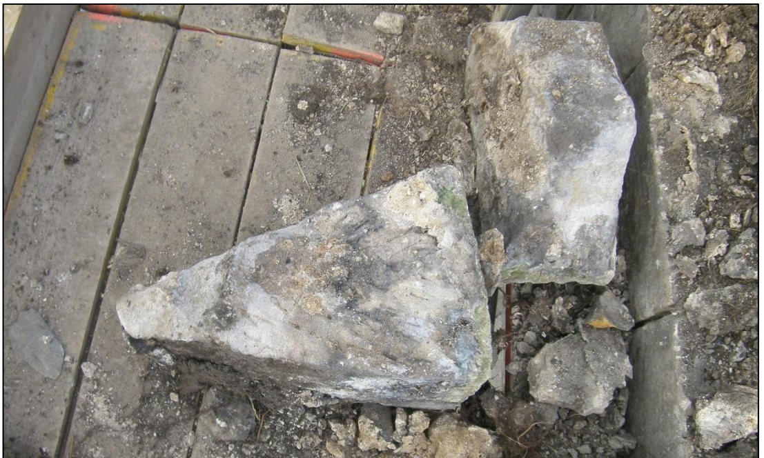
Plate 8: example of a tapering, triangular through-stone.
