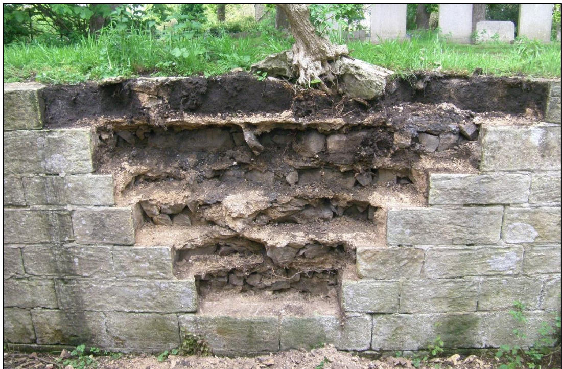
Plate 20: Section 1 of the west ha-ha after removal of the ashlar facing.
