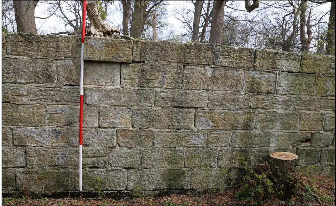
Plate 19: pre-intervention photograph of Section 1.
