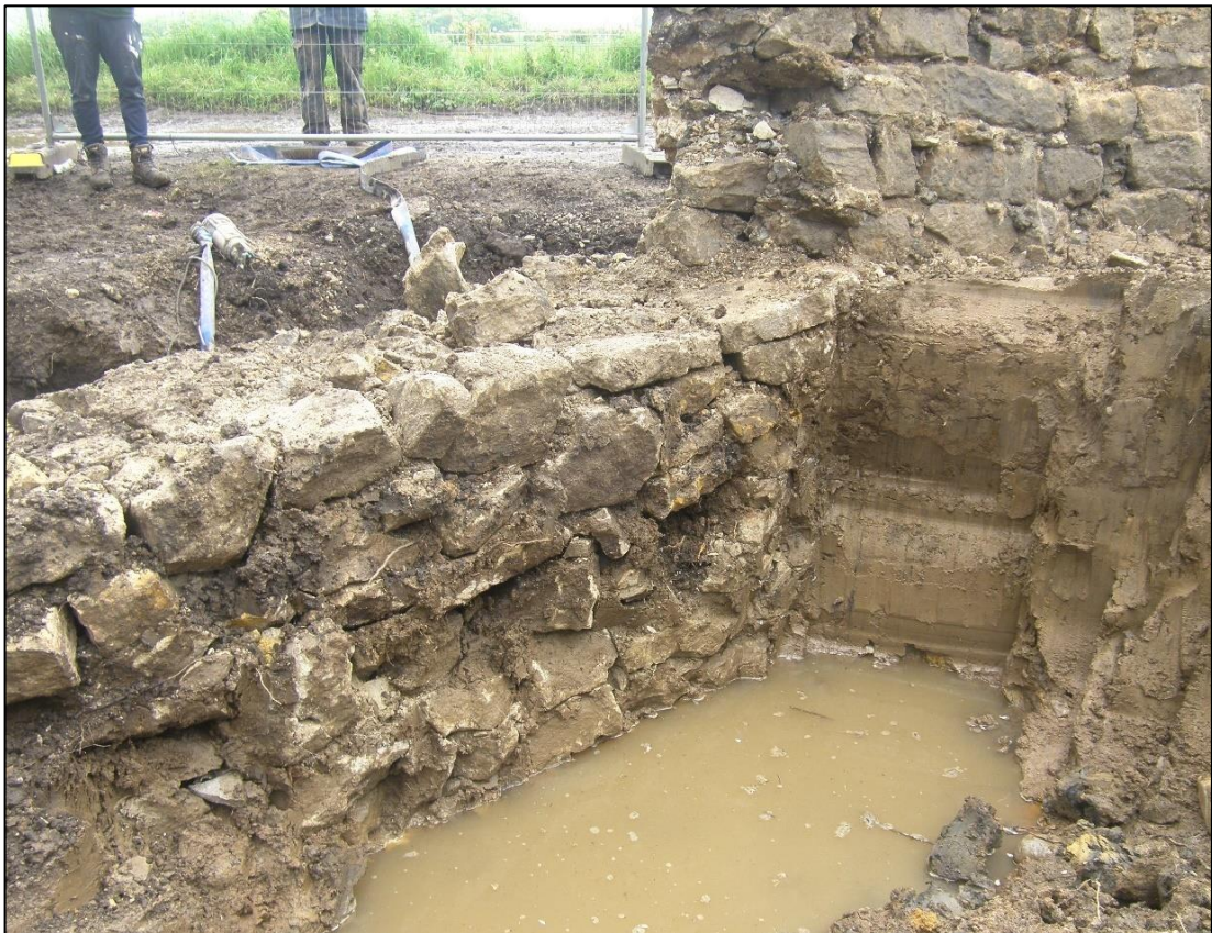
Plate 10: inner foundation of the south-west bastion, cut into natural clay.
