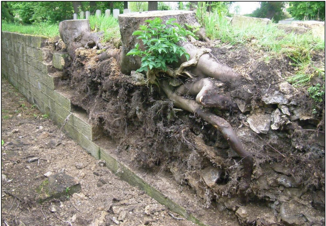
Plate 22: Section 2 of the west ha-ha after removal of the ashlar facing.
