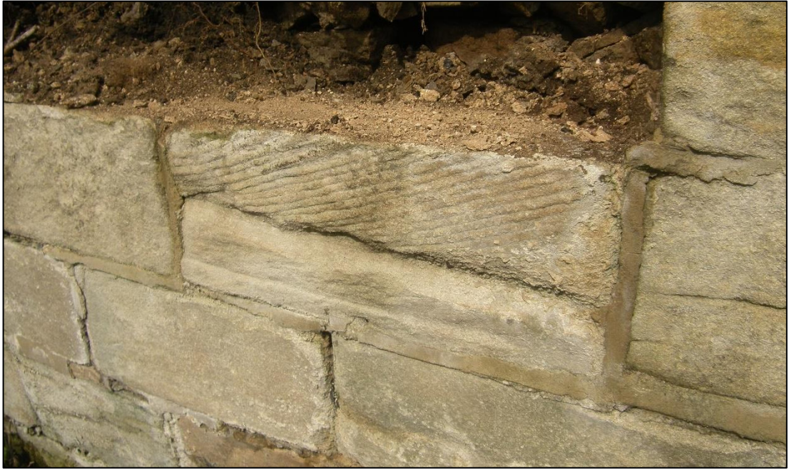
Plate 27: potentially reused facing stone in Section 4 of the west ha-ha.
