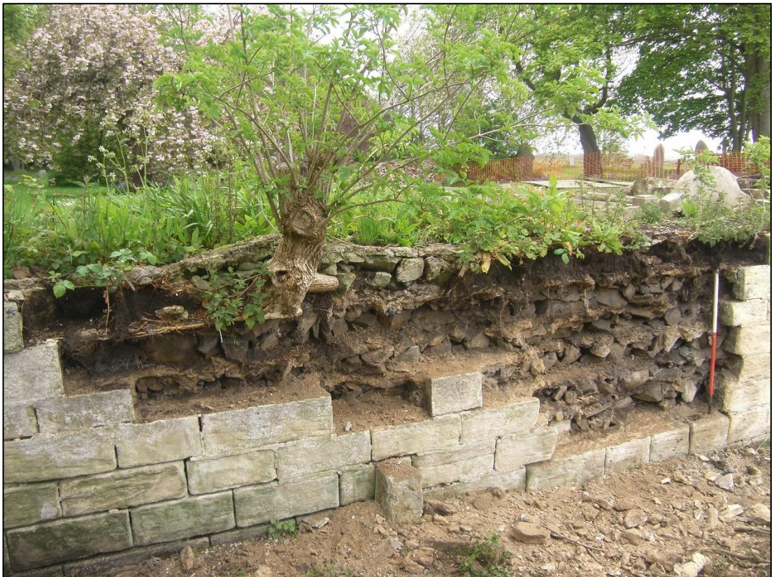
Plate 29: Section 5 of the west ha-ha after the removal of the ashlar facing.
