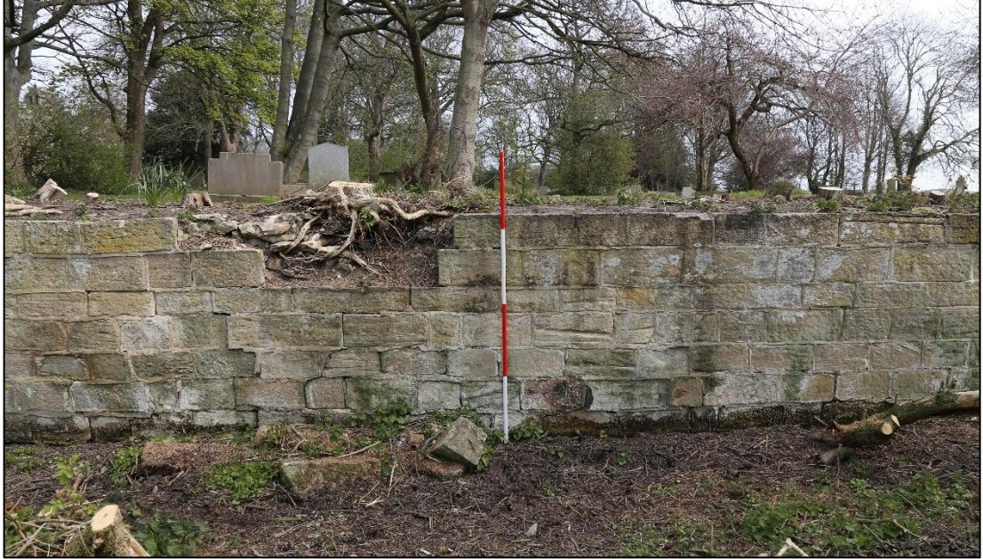
Plate 25: pre-intervention photograph of Section 4.
