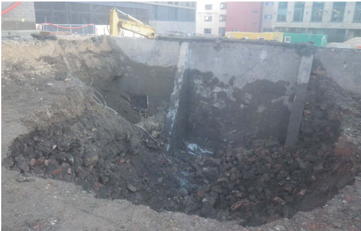
Plate 2: reinforced concrete wall and brick rubble infill in the western half of Plot A.
