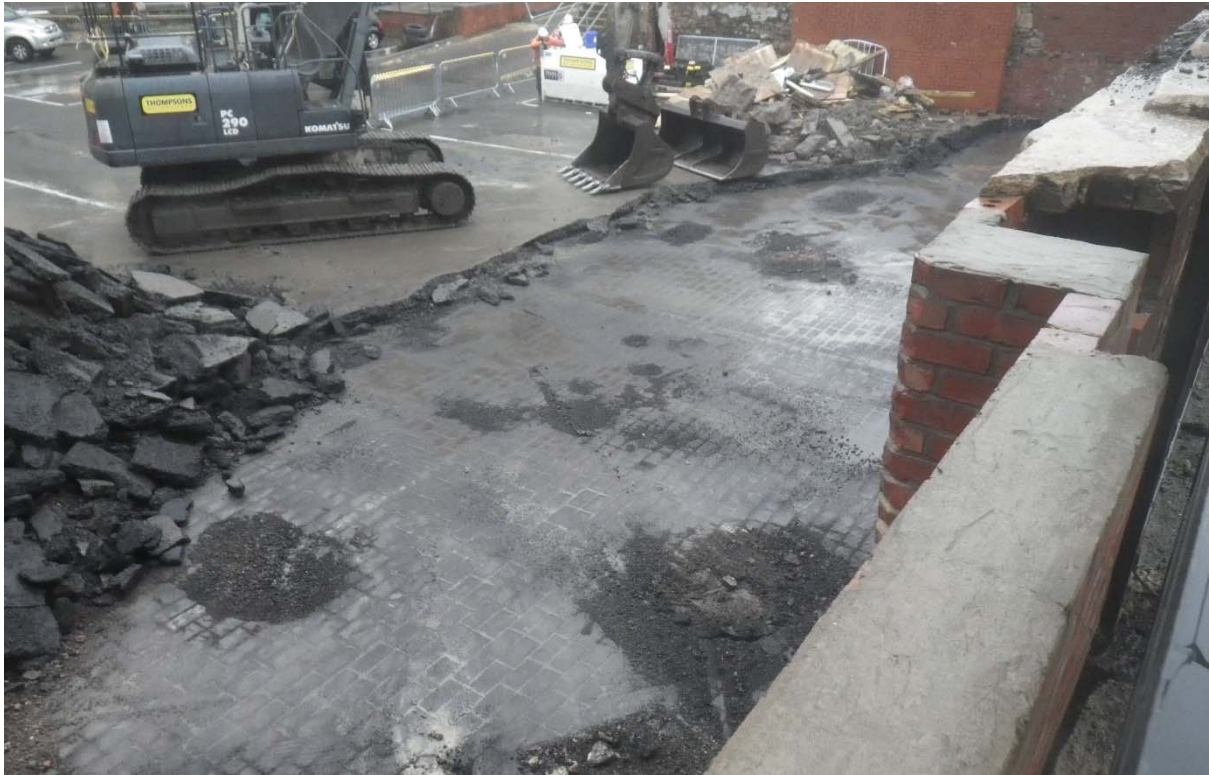
Plate 4: concrete yard surface beneath the modern carpark in Plot C.
