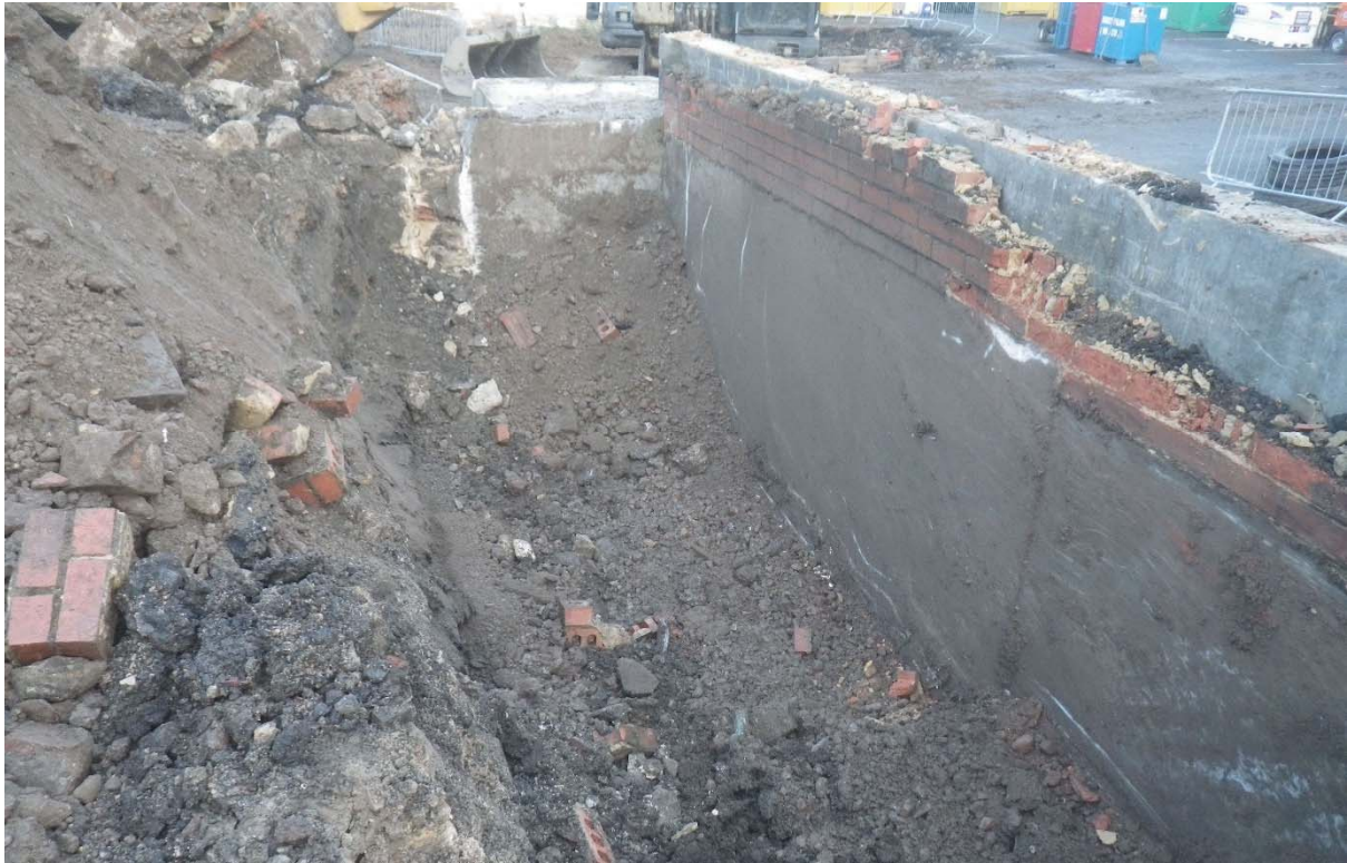
Plate 3: remains of 19th-century terrace wall in the southern extent of Plot B, with reinforced concrete wall on the right.
