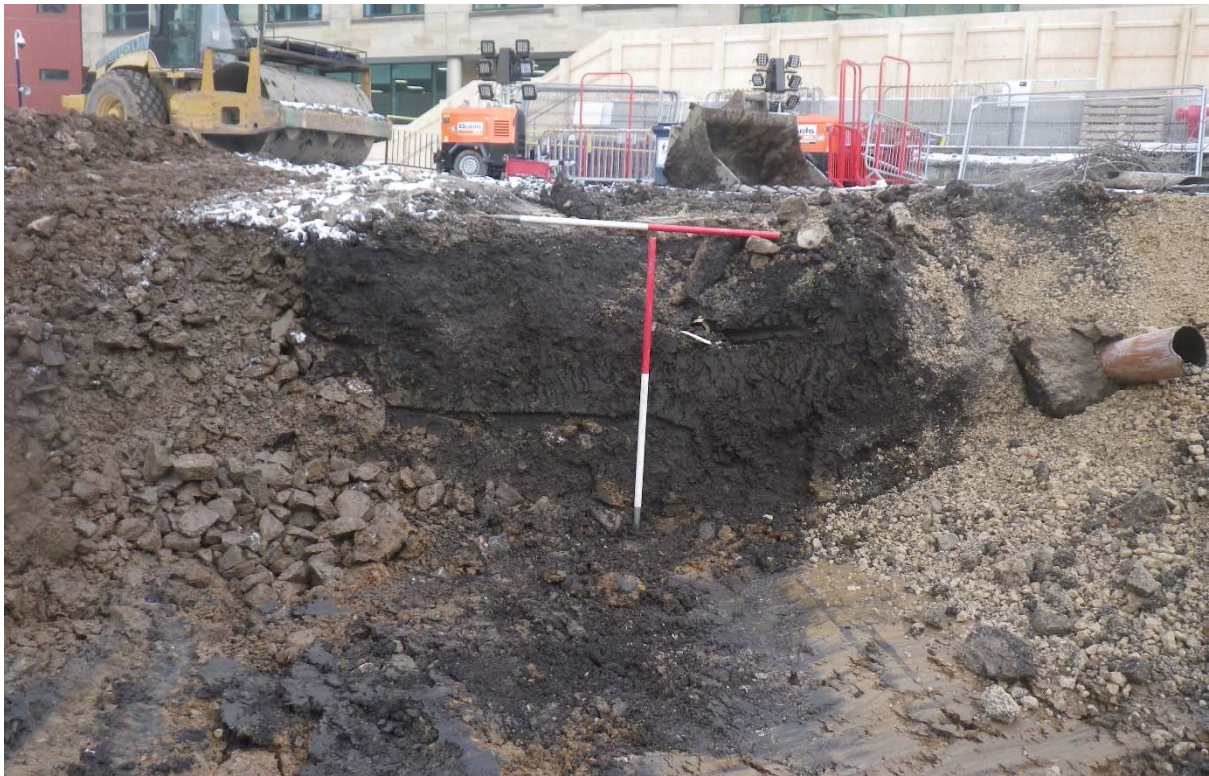
Plate 6: depth of garden soil 2 surviving within the walls of the 19th-century sawmill.
