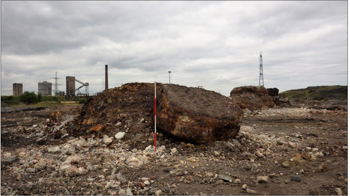
Plate 10: blast furnace 03 , facing north (furnaces 02 and 01 in the background); displaced salamander in the foreground
