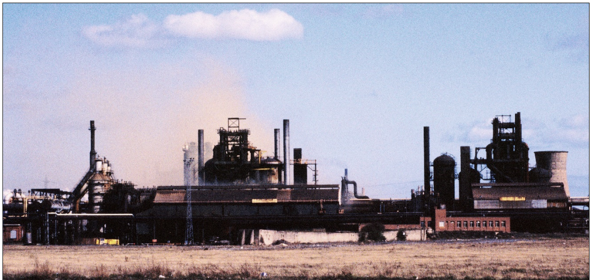
Plate 5: The Cleveland Steel Works in 1993, No 4 is in the middle, No 5 to the right, and gas cleaning plant to the left.
