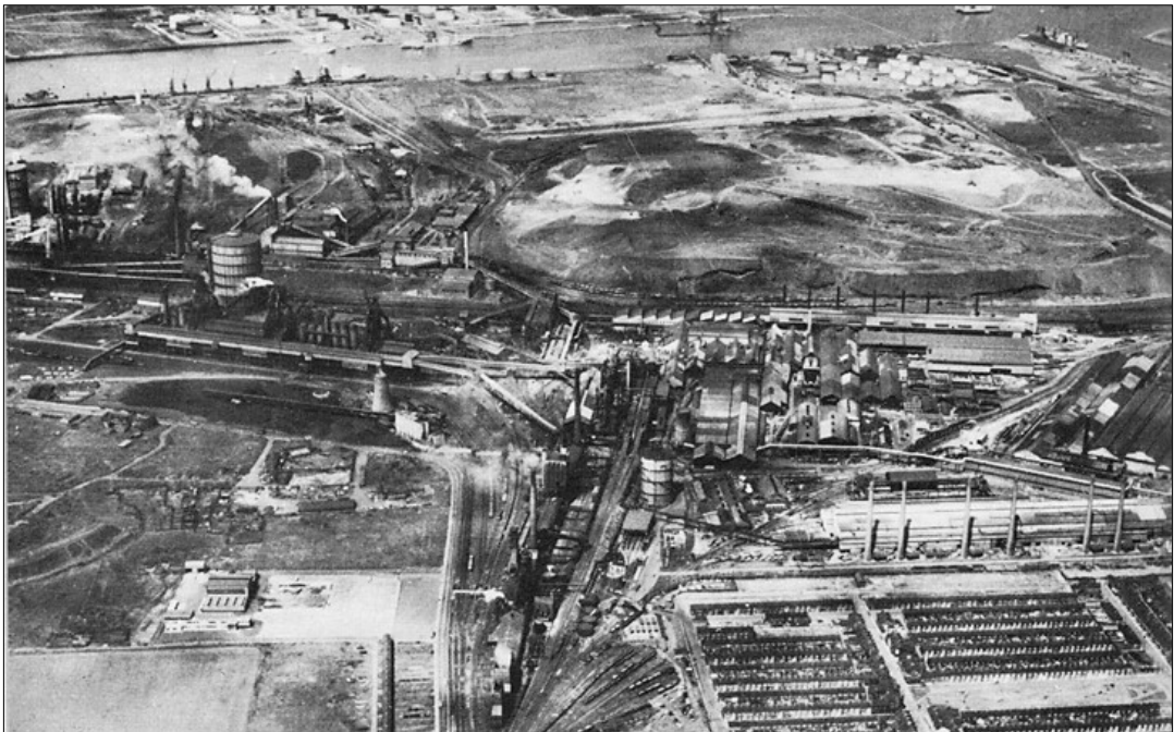
Plate 1: aerial photo of Dorman Long Cleveland Works from mid 1960s; the bank of blast furnaces run up the centre of the photograph
