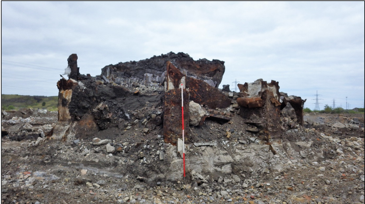
Plate 8: the northern blast furnace base 01 – No. 4. Facing north
