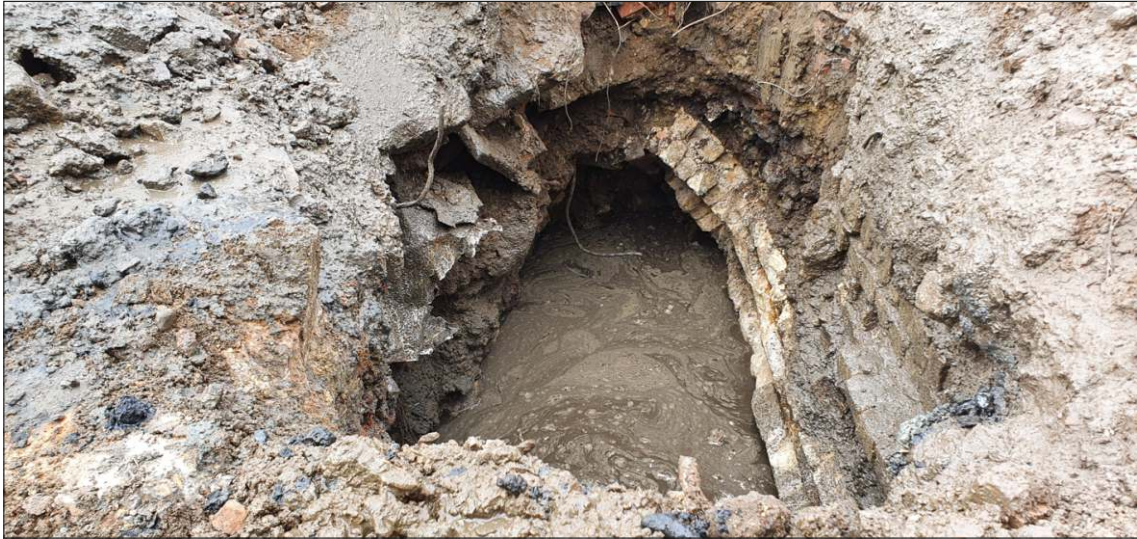
TVERF, Grangetown: DS15 showing brick-built tunnel or flue
