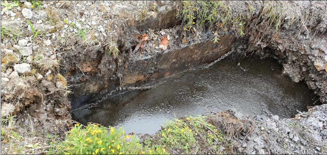
TVERF, Grangetown: DS1b / TP17 showing concrete lining of possible chamber and chain
