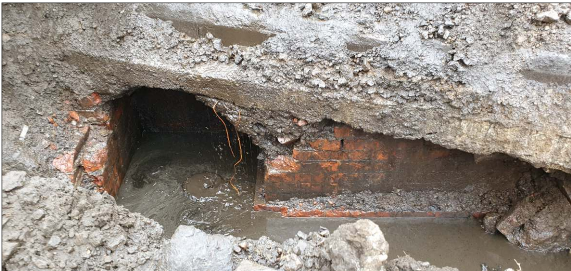
TVERF, Grangetown: TP6b showing brick-built tunnel or flue
