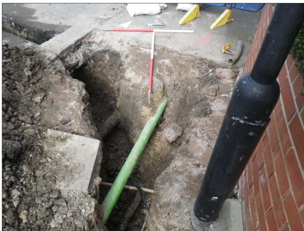
Plate 2: Trench cut through footpath showing existing services
