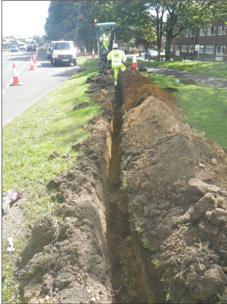
A69 Lighting, West Denton: trenching through bedrock south of A69 Plate 7
