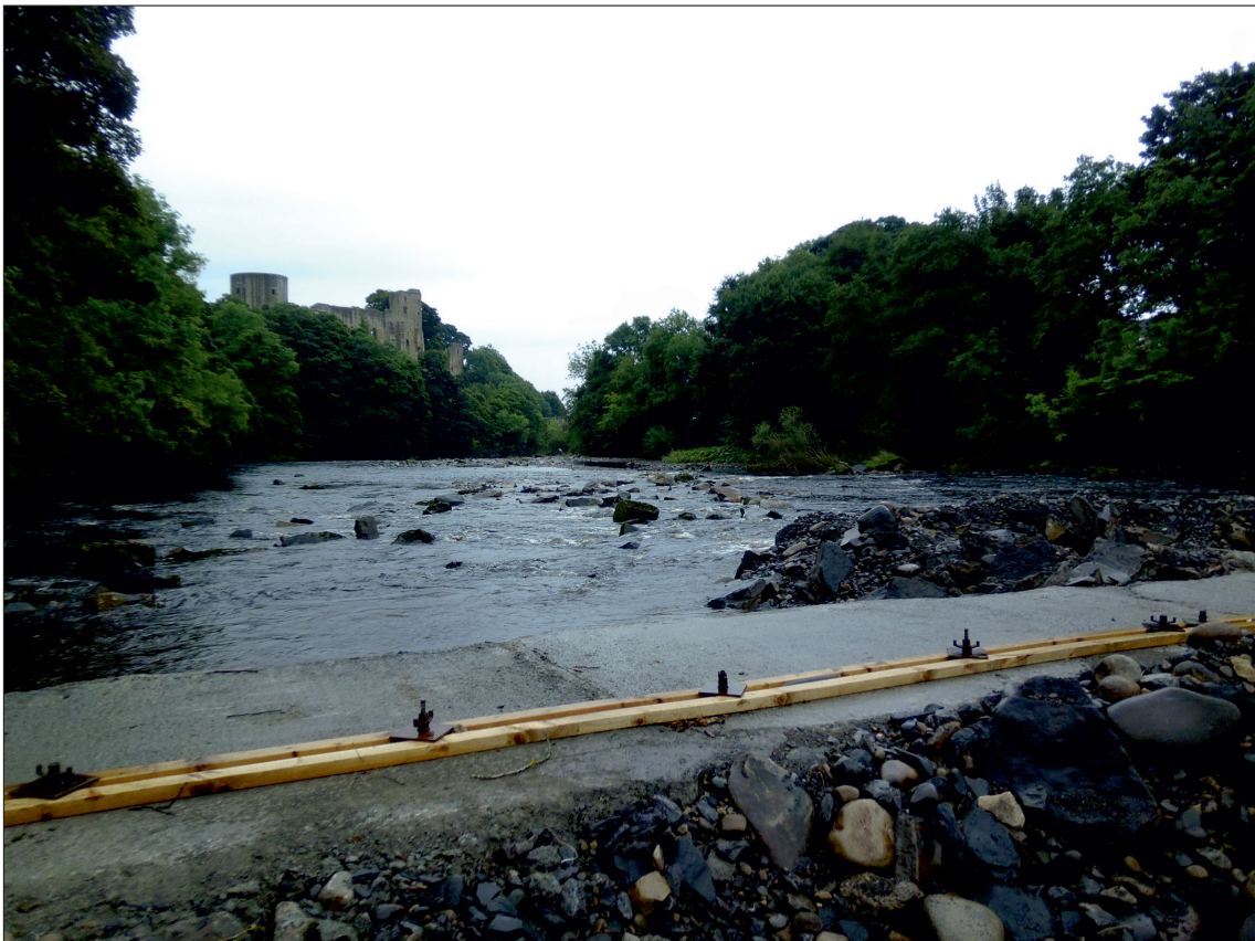
Barnard Castle Weir: temporary wall in River Tees
