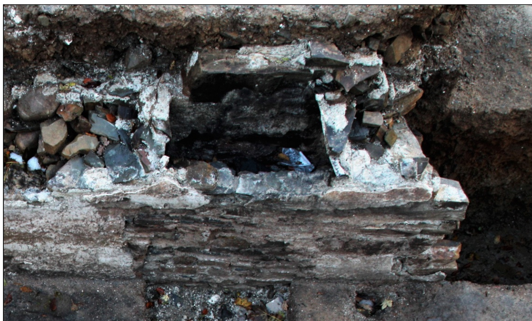
Plate 4: overview of blocked fireplace and chimney built into wall 1060
