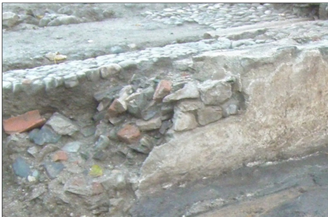
Plate 9: detail of masonry 1081 blocking embrasure within wall 1080
