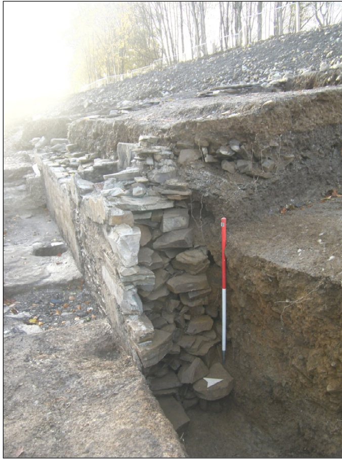
Plate 2: oblique view of construction cut 1023 containing wall 1060
