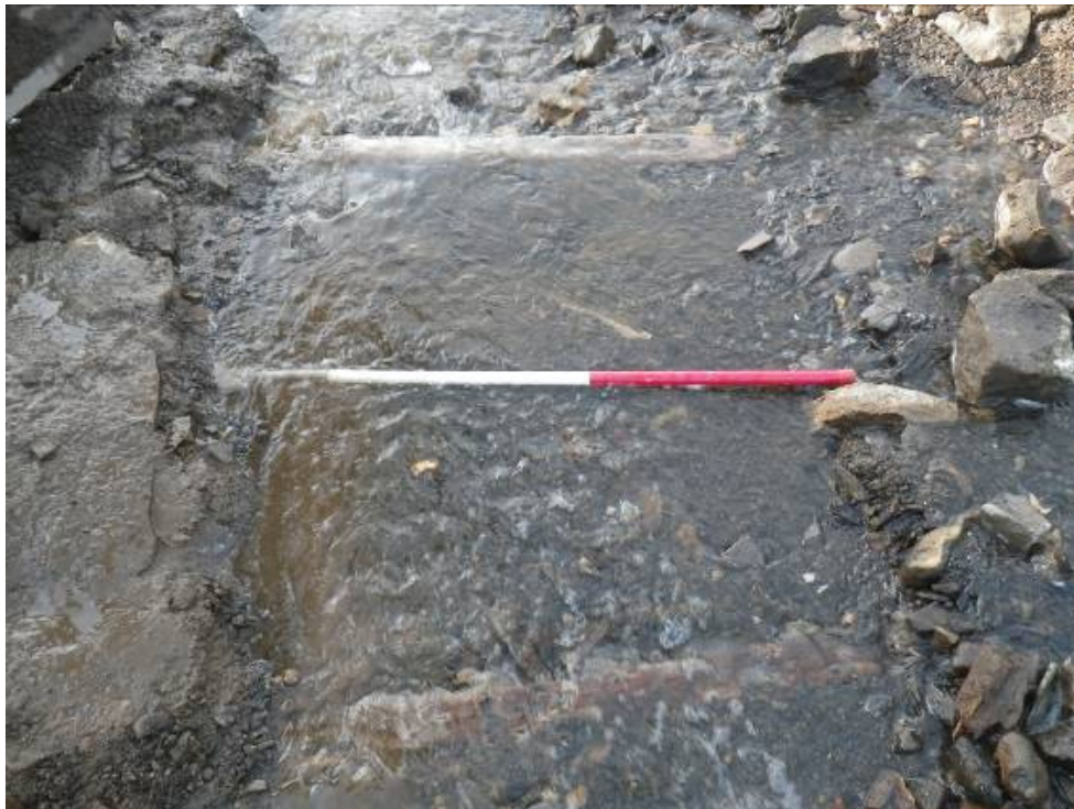
Plate 63: In situ timber set into wall footing.
