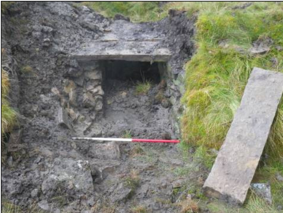
Plate 46: Removal of fallen lintel to expose collapsed wall.
