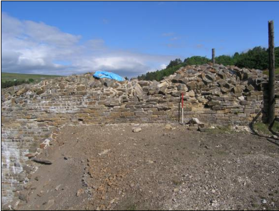
Plate 34: Pre-intervention image of Spine Wall Feature 4 to be rebuilt.
