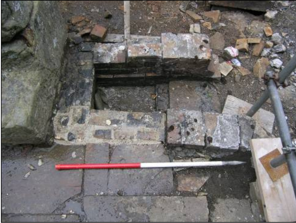
Plate 5: Reconsolidation of structure with scaffolding to the right.
