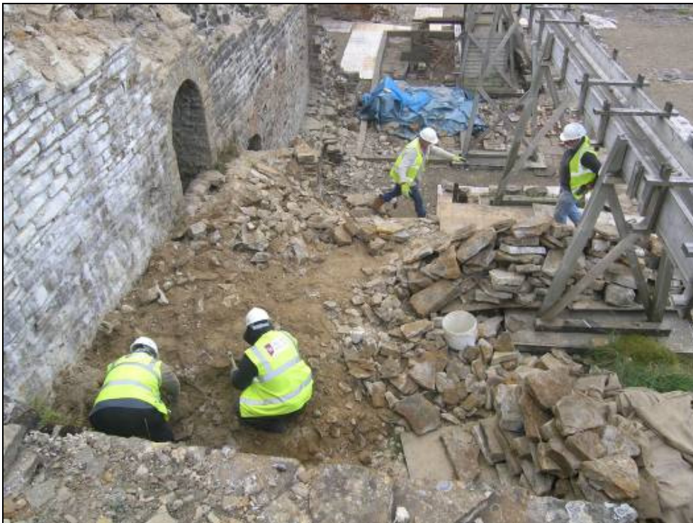
Plate 7: Smelt Mill Feature 4 debris clearance.
