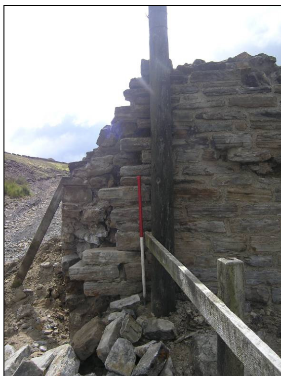
Plate 37: Spine Wall Feature 5 – corner - during dismantling.
