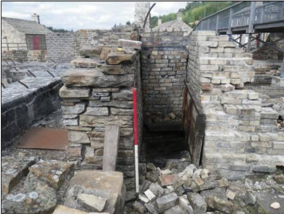
Plate 27: Feature H3 northwest elevation pre-intervention.
