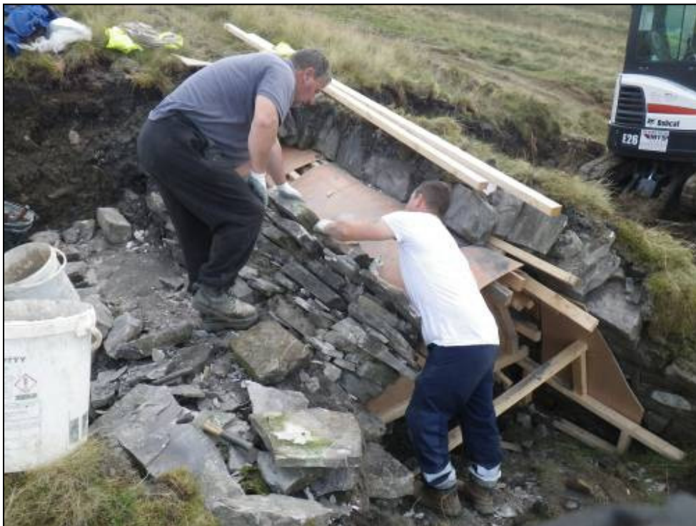
Plate 50: Flue 05 being rebuilt around timber former.
