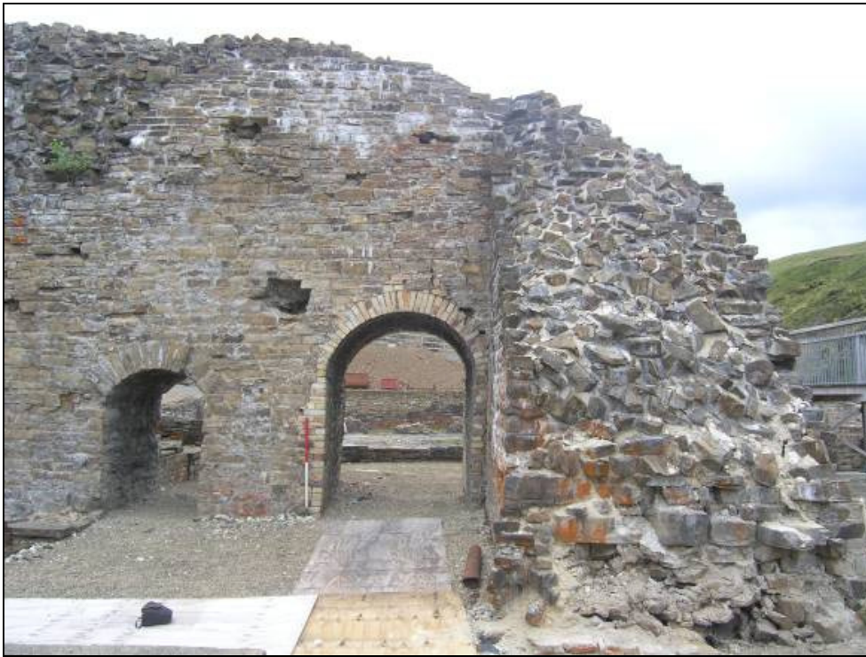
Plate 41: Spine Wall Feature 6. Section of bulging spine wall above archway with series of voids.
