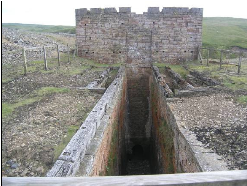
Plate 58: Stagg Condenser wheel pit.
