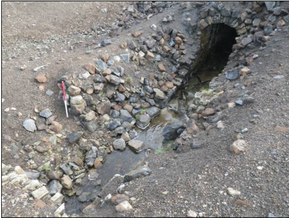
Plate 64: Western section of Rampgill Burn culvert pre-intervention.
