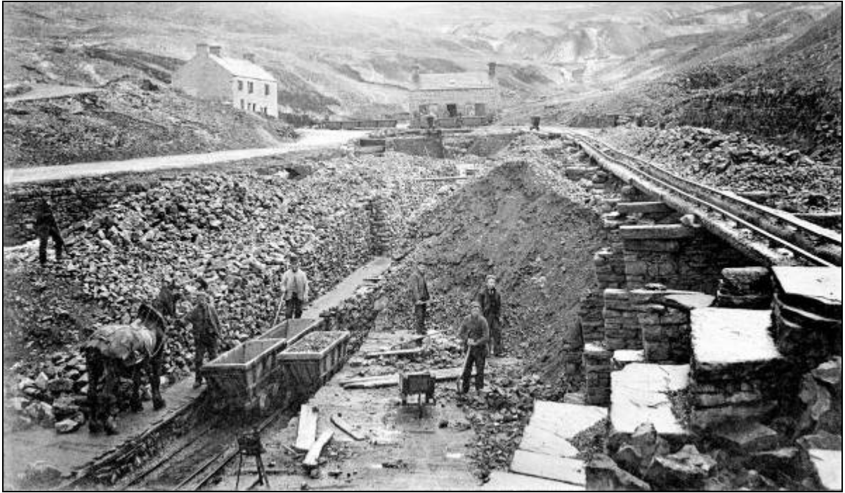
Plate 54: Construction of Smallcleugh culvert.
