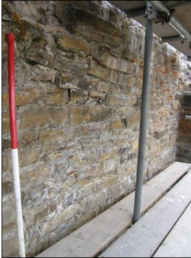
Plate 42: Spine Wall Feature 6 post intervention (area at top of image).
