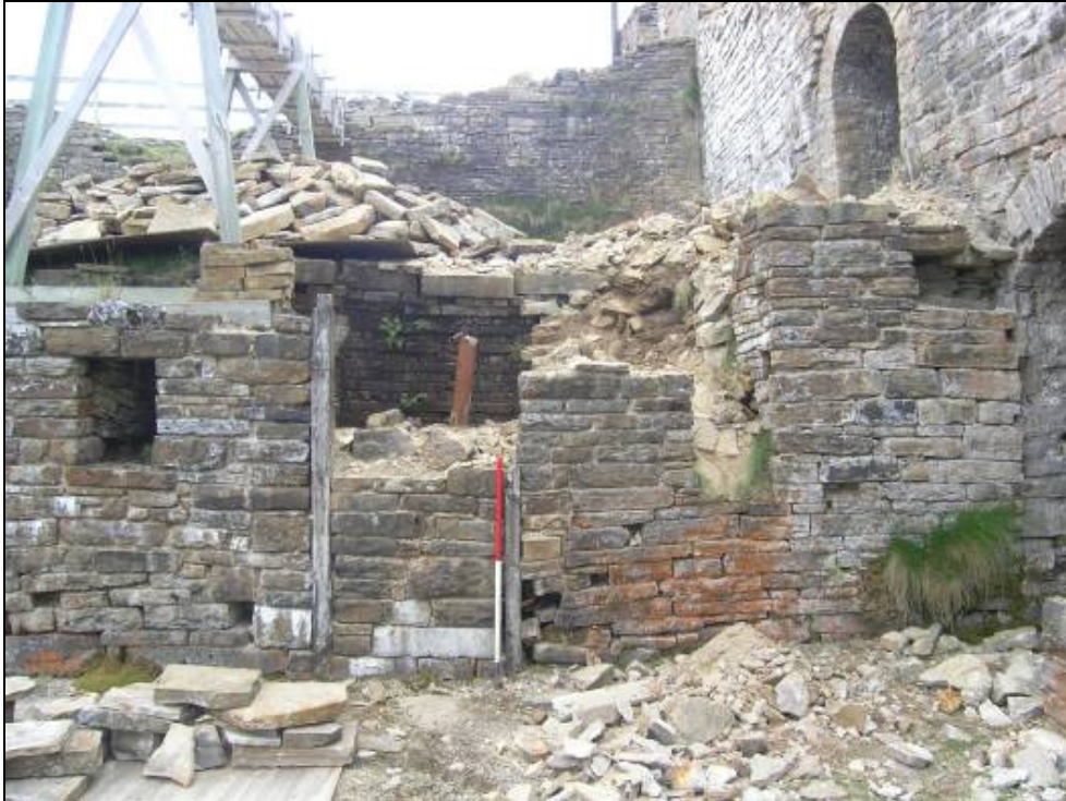
Plate 6: Smelt Mill Feature 4 showing bricked up door and timber frame.
