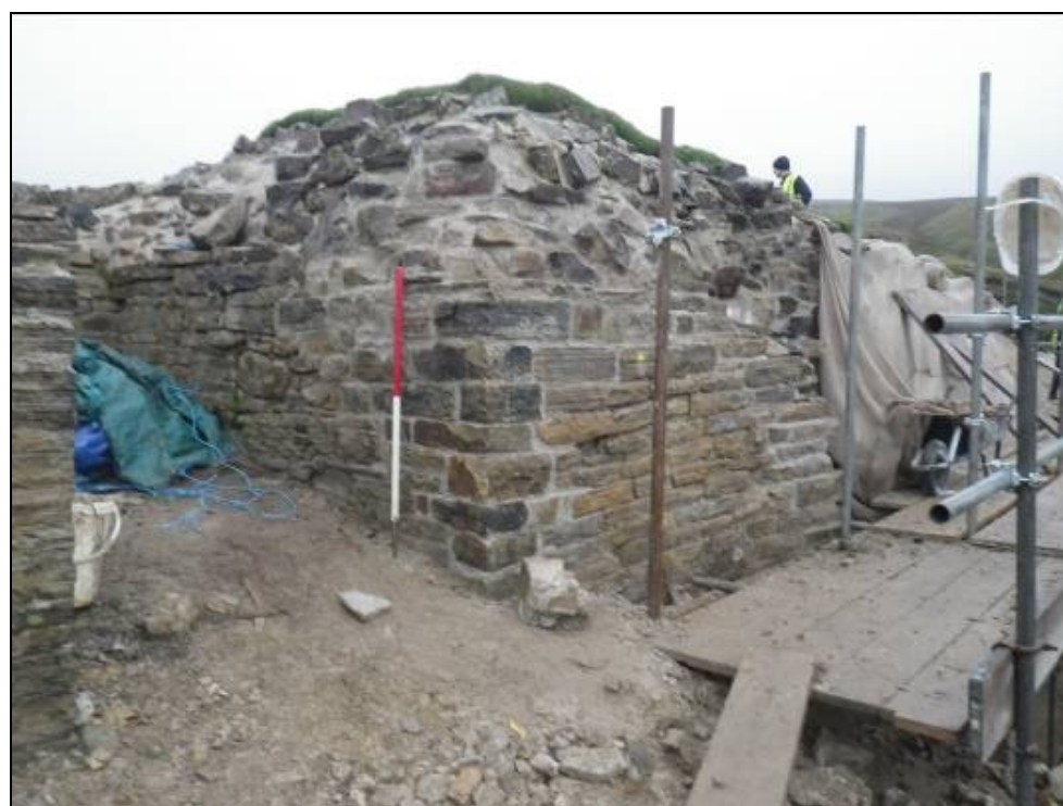
Plate 40: Rebuilt corner and face of spine wall.
