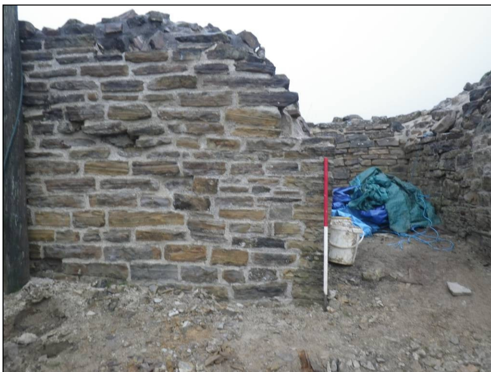
Plate 36: Spine Wall Feature 5 - wall - post intervention.
