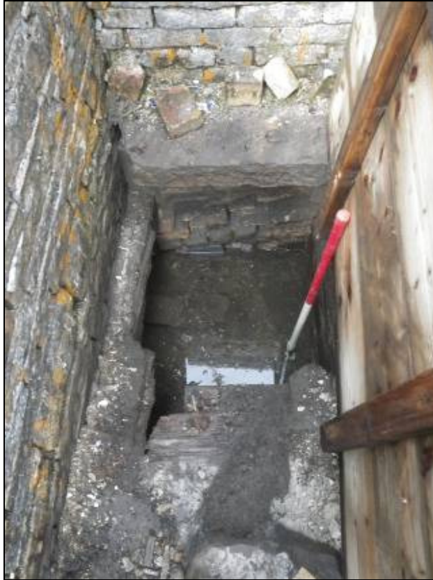
Plate 26: Drain structure beneath Feature H2.
