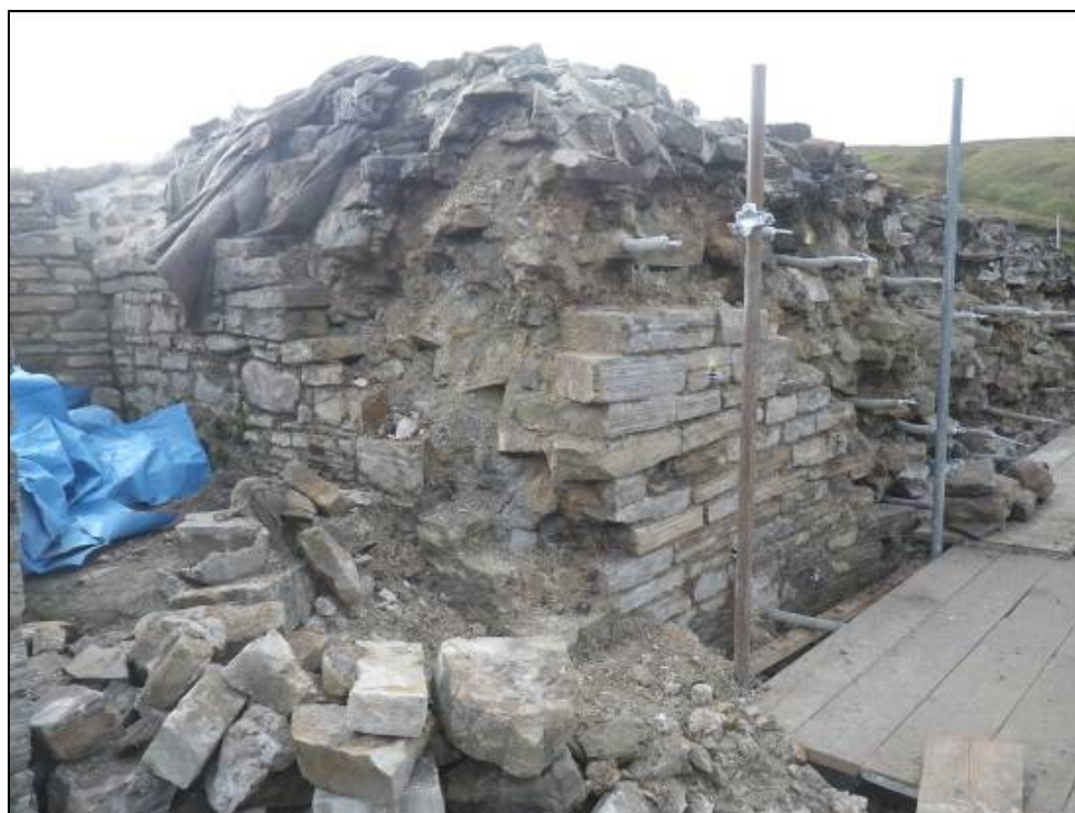
Plate 39: Site visit 21/10/14 showing dismantled corner.
