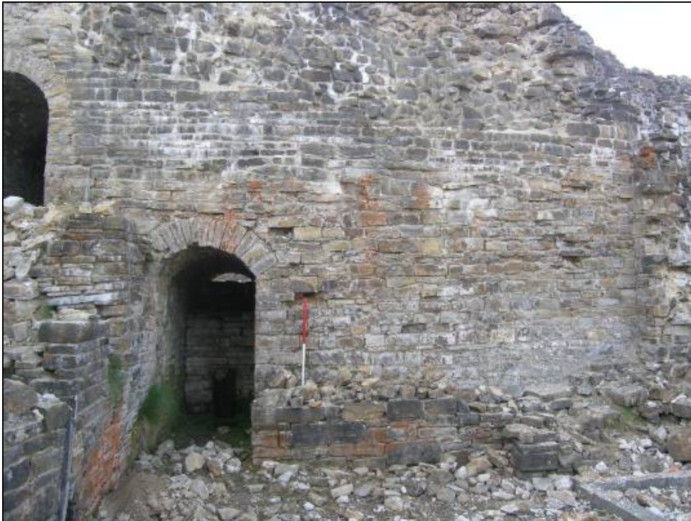
Plate 11: Smelt Mill Feature 7 showing wall butting against northwest face of spine wall.
