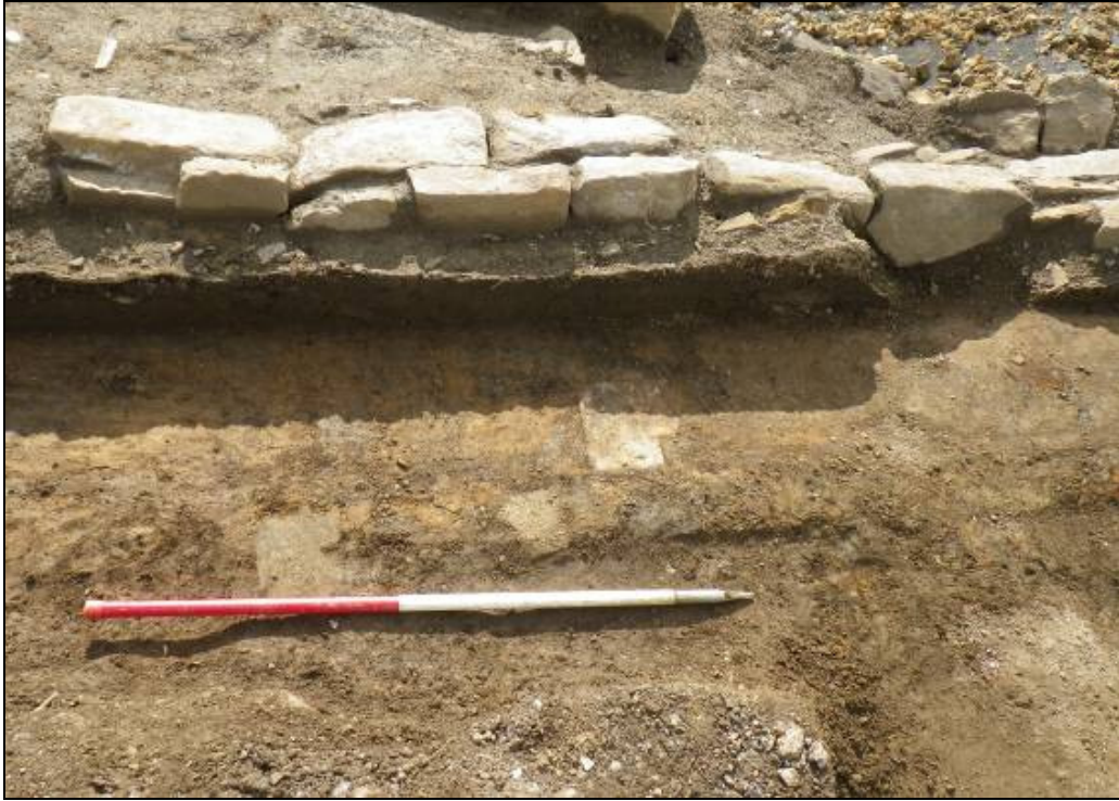
Plate 70: Retaining wall for chute.
