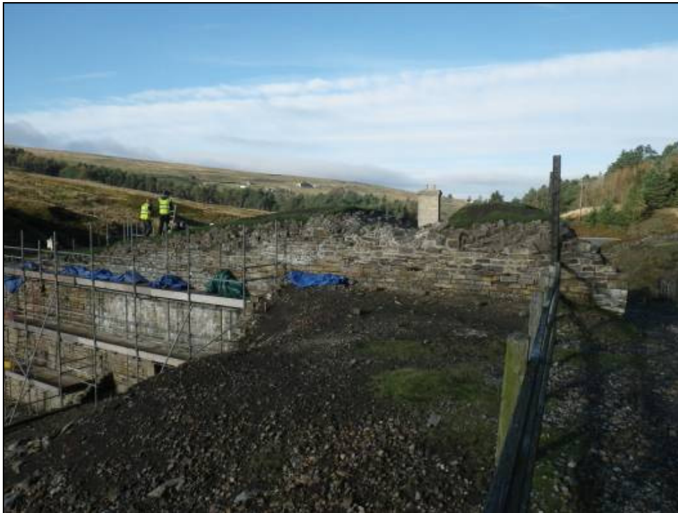
Plate 44: Installation of spine wall soft capping.
