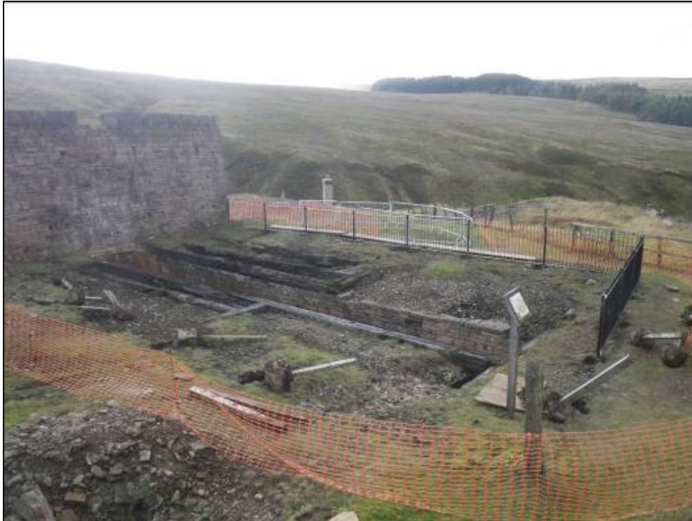
Plate 59: Photograph taken during fence installation.
