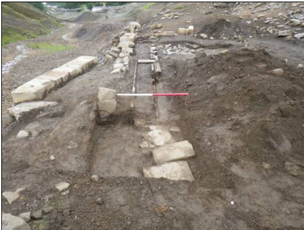
Plate 66: Timber chute looking northwest towards smelt mill complex.
