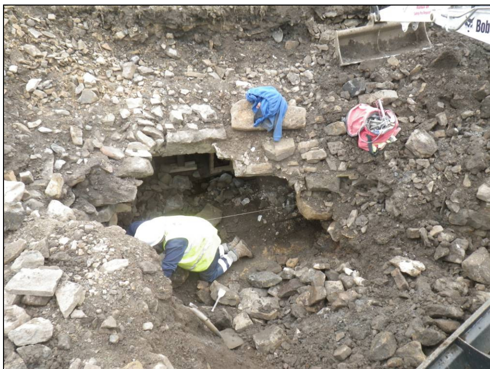
Plate 57: Wall (017) removed down to the bed of the culvert.
