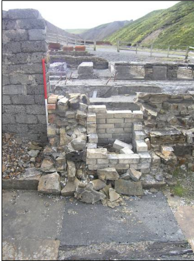
Plate 17: Feature C1 (Pattinson House) pre-intervention.
