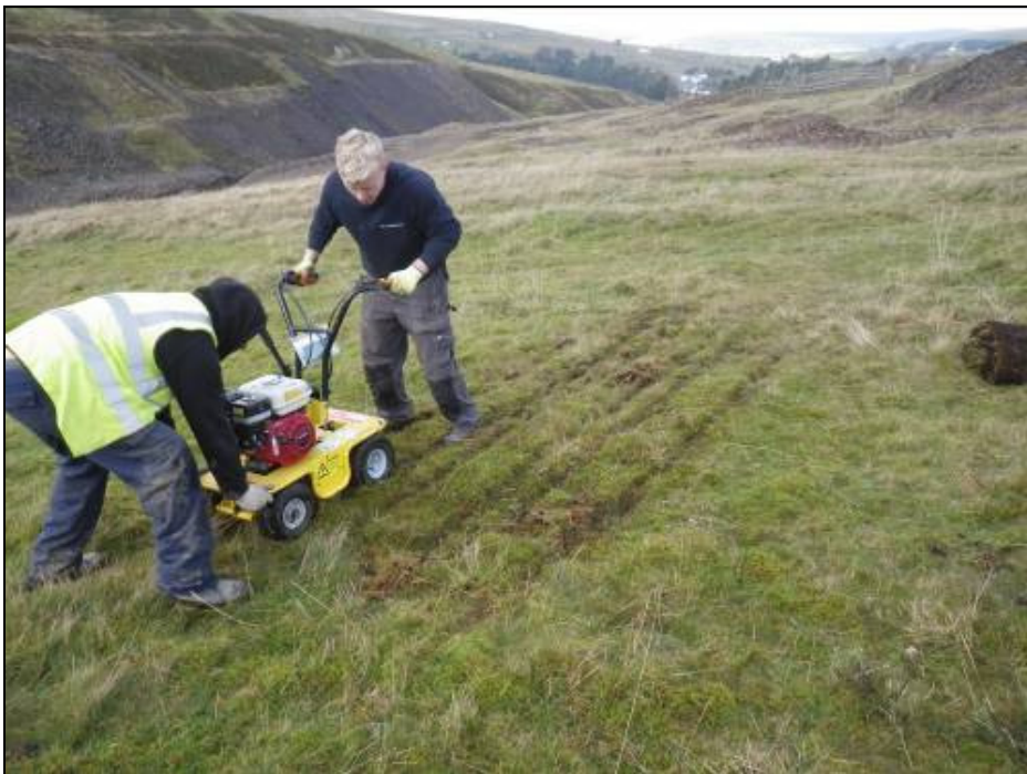
Plate 43: Turf removal for spine wall soft capping.
