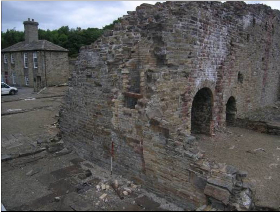
Plate 23: Building F1. Southwest end of spine wall prior to anchor installation.
