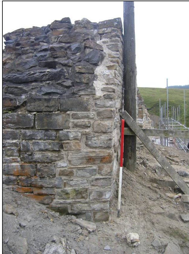
Plate 38: Spine Wall Feature 5 post intervention.
