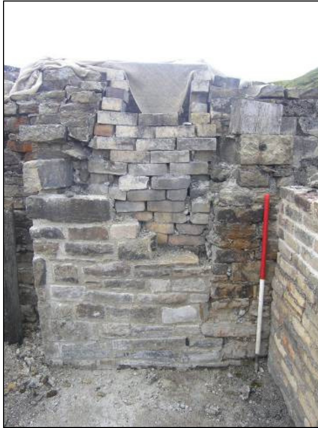
Plate 20: Feature C2 post intervention.
