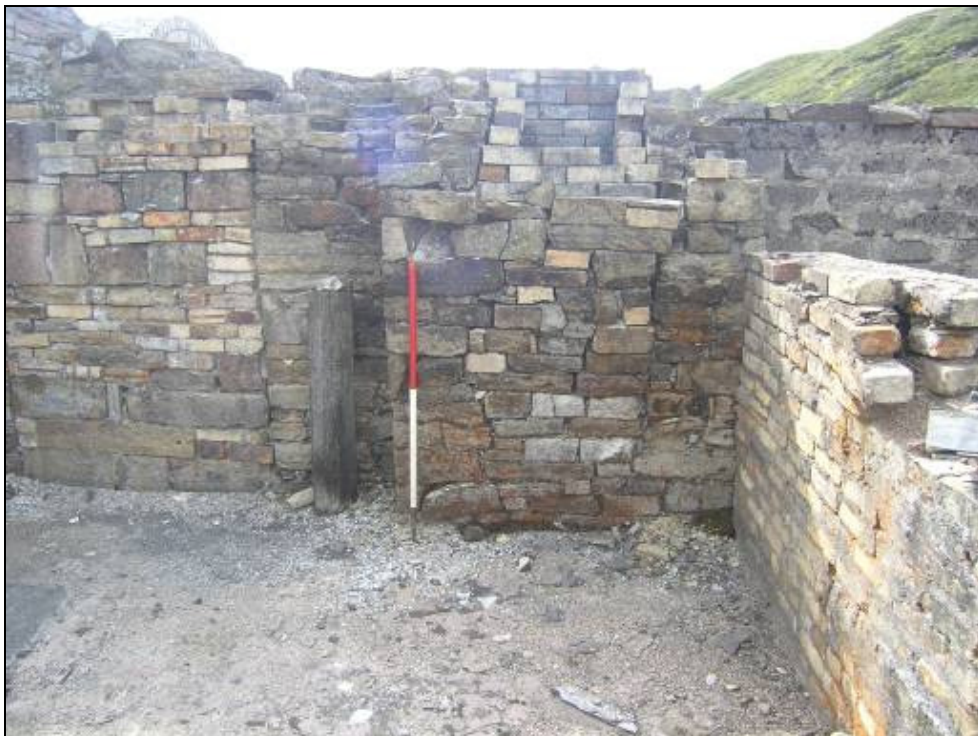
Plate 19: Feature C2 pre-intervention.
