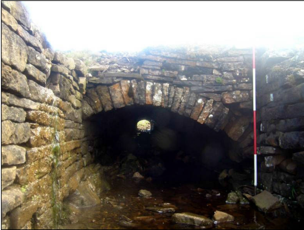
Plate 53: Downstream culvert entrance showing off centre arch.
