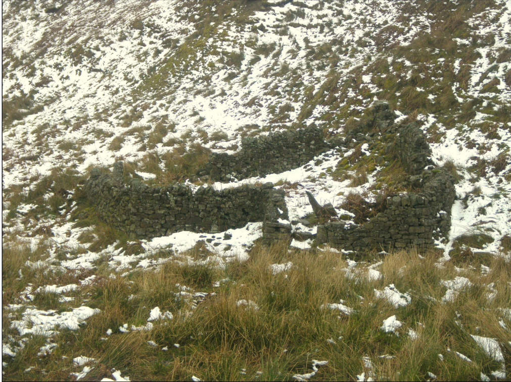
Plate 16: Sheepfold 10259, located on the west side of Heugh Gill, facing west.
