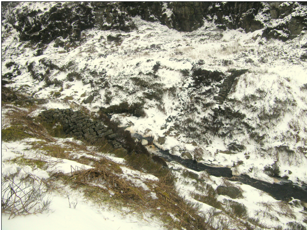
Plate 18: The remains of a substantial bridge (10333) crossing Barden Beck.
