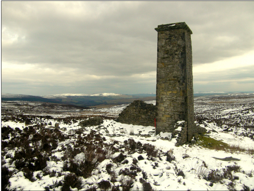
Plate 12: Remains of structure with chimney (10001), facing south-east.
