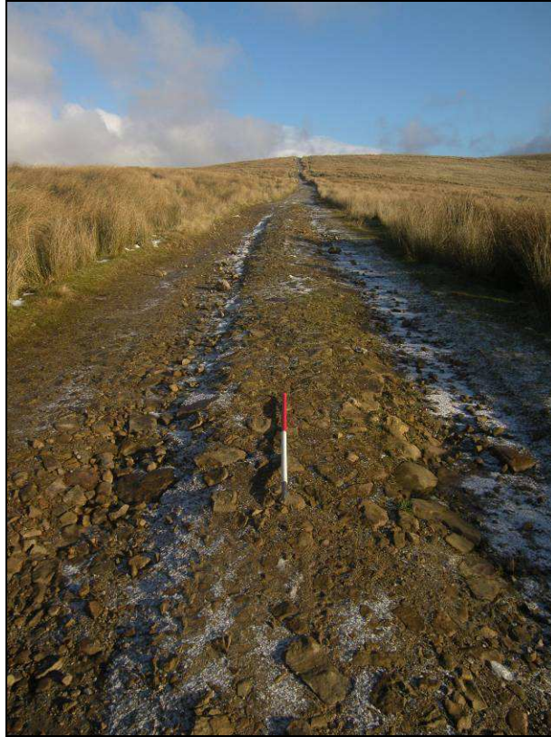
Plate 3: Survey Area 1, Cam High Road, facing north-east
