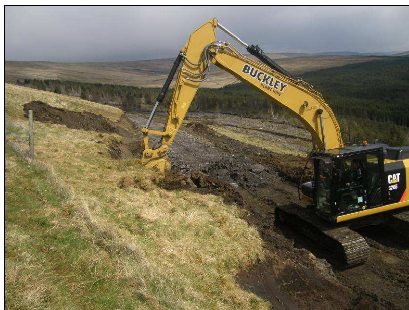
Plate 7: Construction of the new track, facing east
