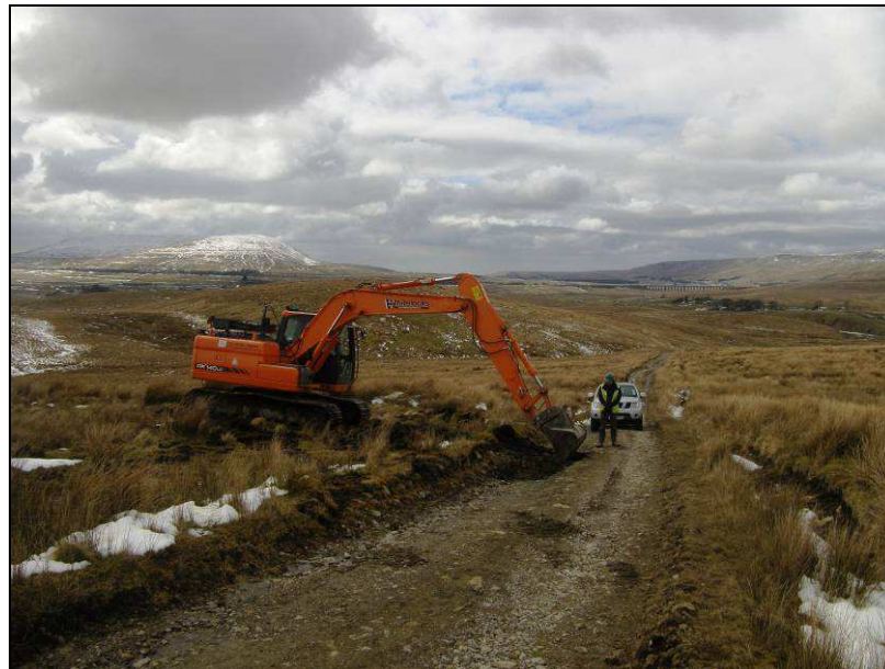
Plate 2: Excavation commences on Cam High Road, facing south-west
