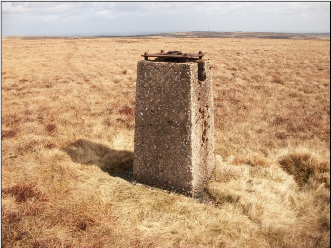
Plate 16 Concrete pillar in open ground between Construction Shaft 4 and Observatory 3
