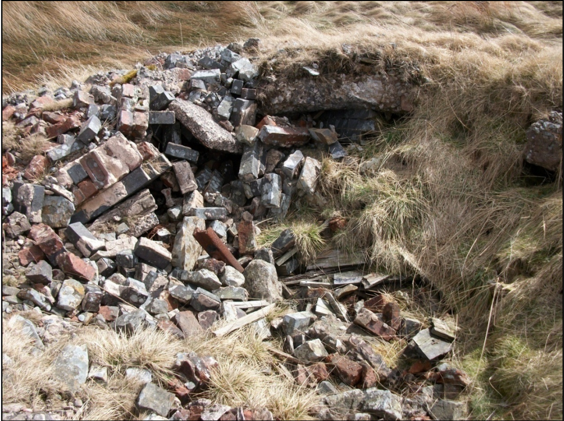
Plate 5 Unconsolidated backfill in Construction Shaft 3
