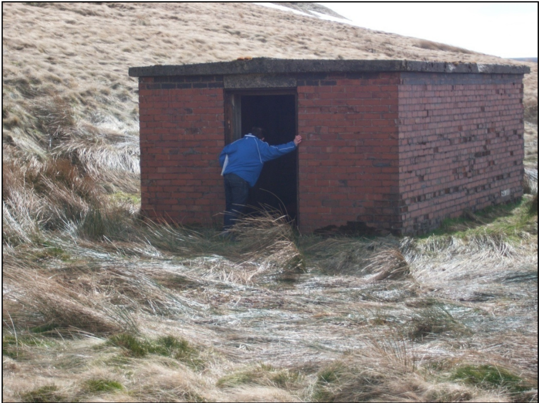
Plate 8 1950s ancillary building from north-west
