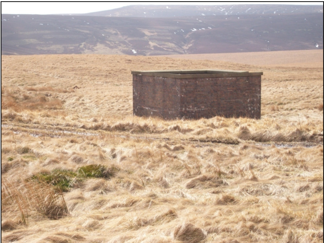
Plate 6 Ventilation tower on site of 1950s Construction Shaft, from the north.
