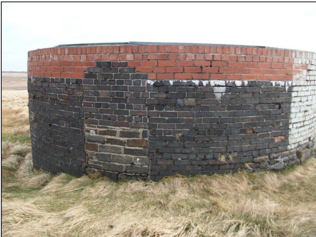
Plate 12 Blocked doorway in ventilation tower, Construction Shaft 5
