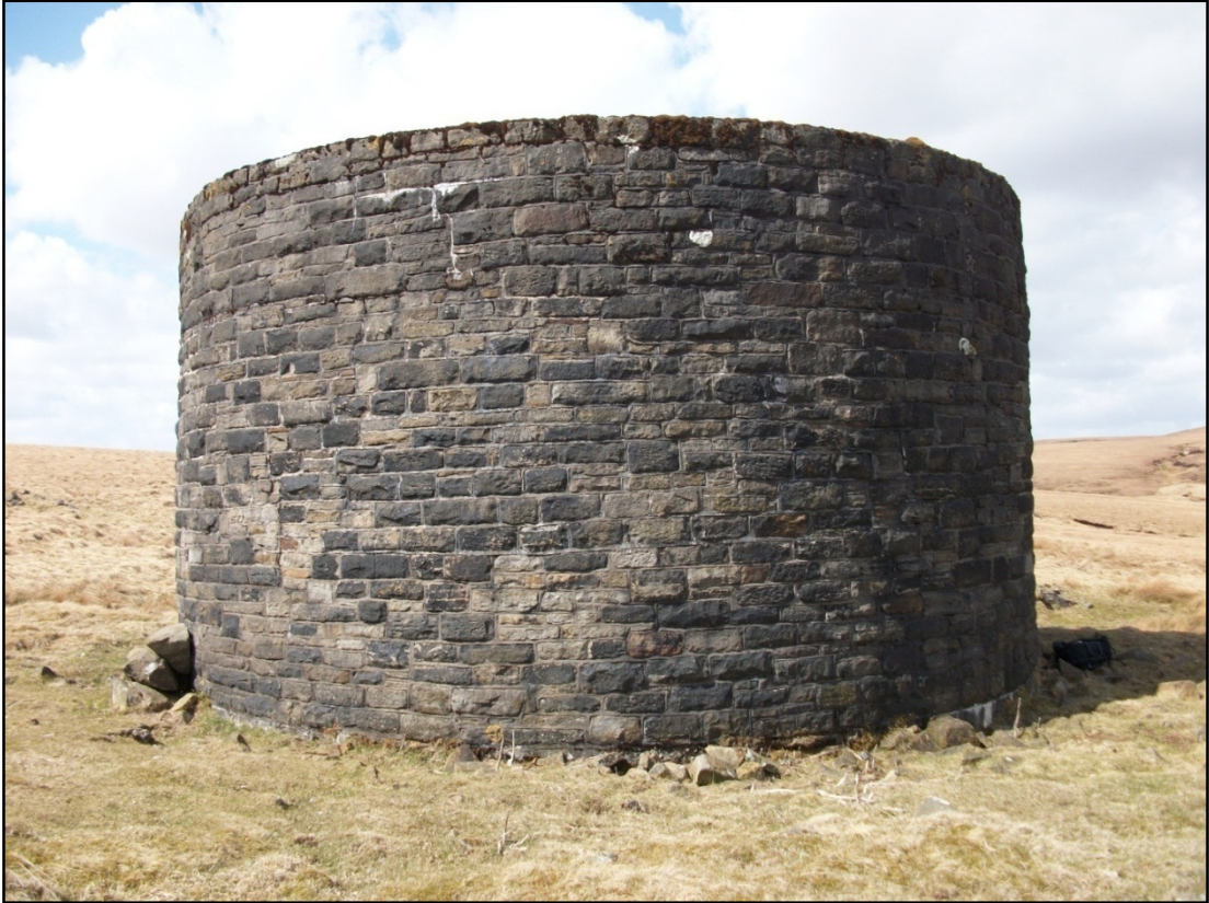
Plate 3 Ventilation tower, Construction Shaft 2 from the south-east
