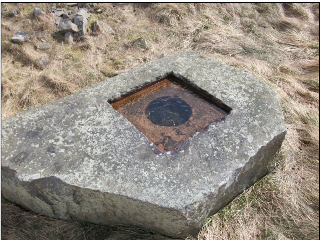
Plate 11 Former bearing-block adjacent to Construction Shaft 4
