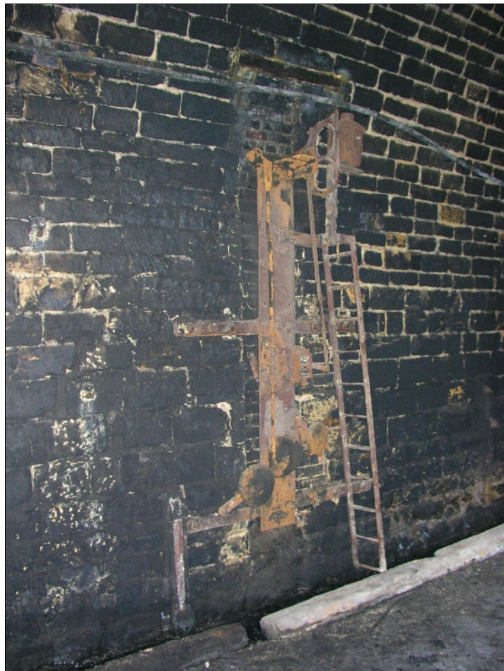
Plate 10 Woodhead Tunnel: Signal Lamp (20th century) and access ladder on south side of South Bore. Lamp faces east
