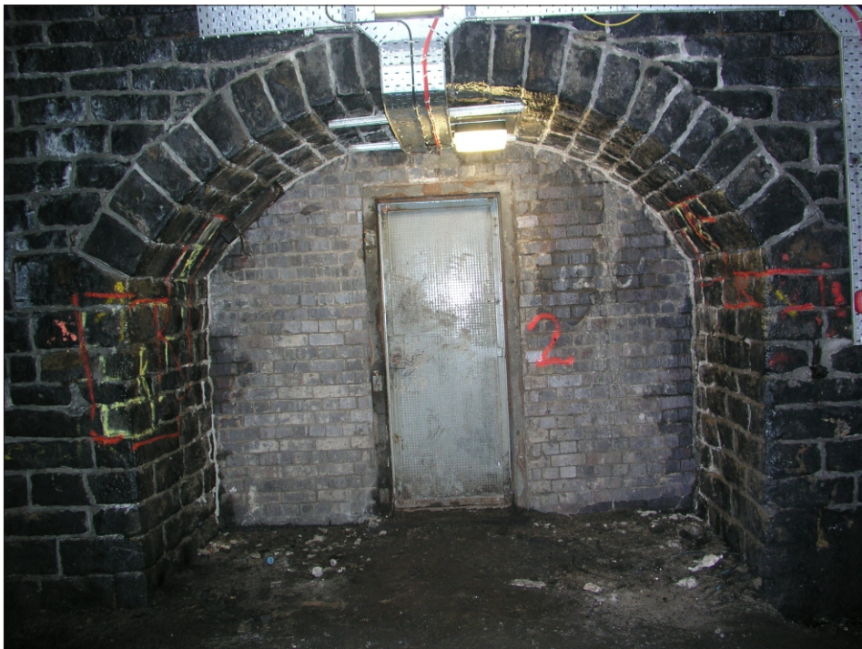
Plate 16 Woodhead Tunnel: Cross passage No.2 incorporating later fire-proof blocking
