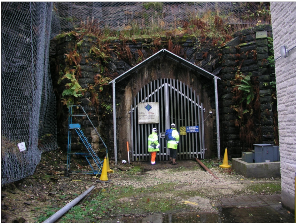
Plate 18 Woodhead Tunnel: Eastern portal to South Bore at Dunford Bridge
