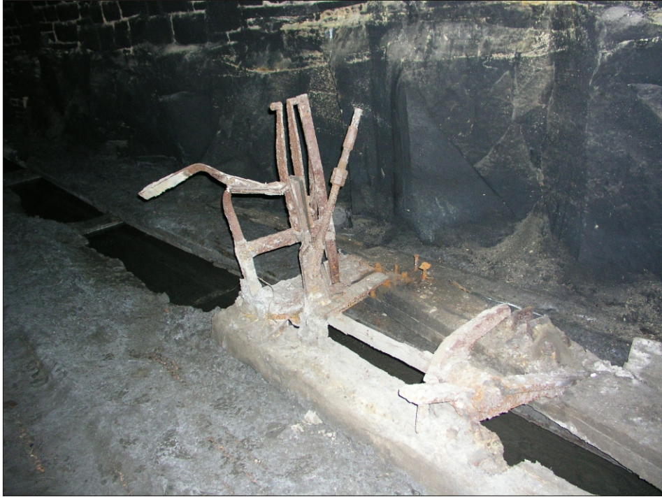
Plate 15 Woodhead Tunnel: Remains of possible points levers
