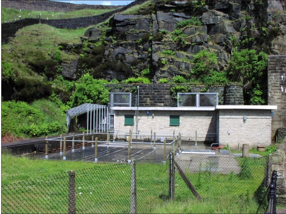
Plate 17 Woodhead Tunnel: View of western portal at Woodhead
