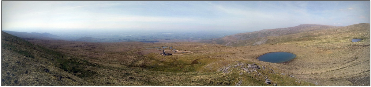
Plate 13: panorama of main mine workings; the Silver Band mine shop is to the centre of the photograph, with Rowpott's Vein hush dam to the extreme right. The land in-between has been scoured out by open cast barytes operations, with the big pond (centre-right) a product of these.
