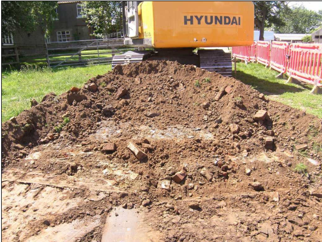
Plate 2. Bricks and rubble within old track surface
