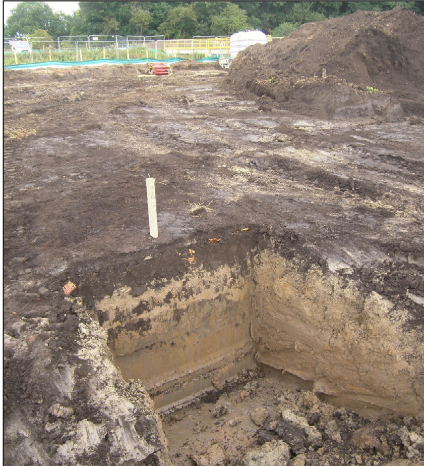
Plate 4: Launch Pit 1 showing organic material and riverine deposits, looking west towards the river.
