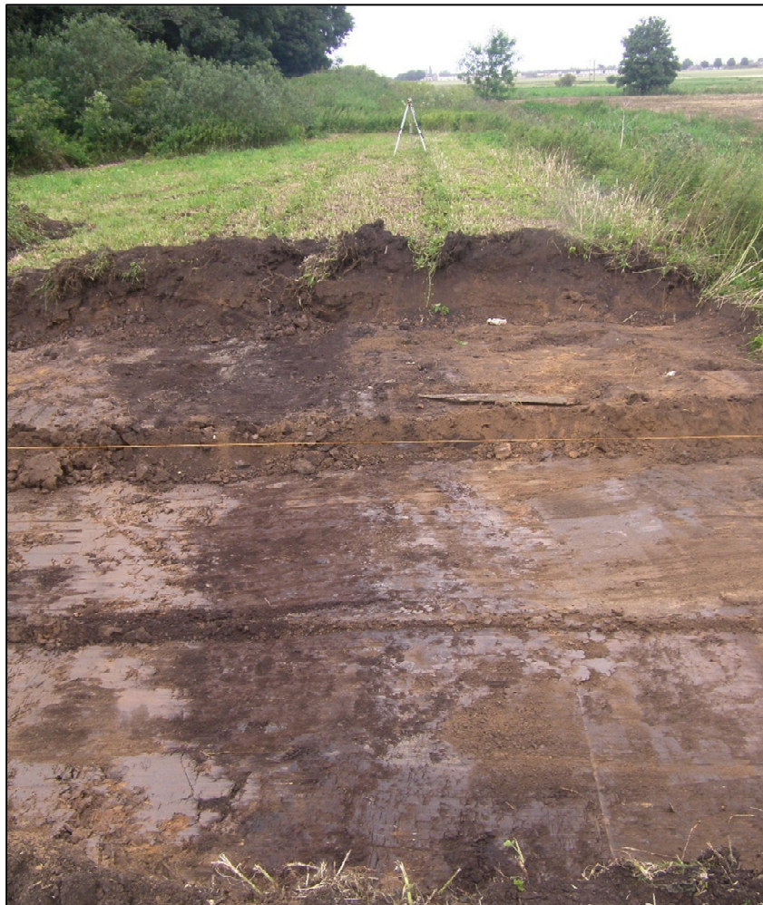
Plate 1: Modern ditch 04 in the bridge footing trench, looking north.
