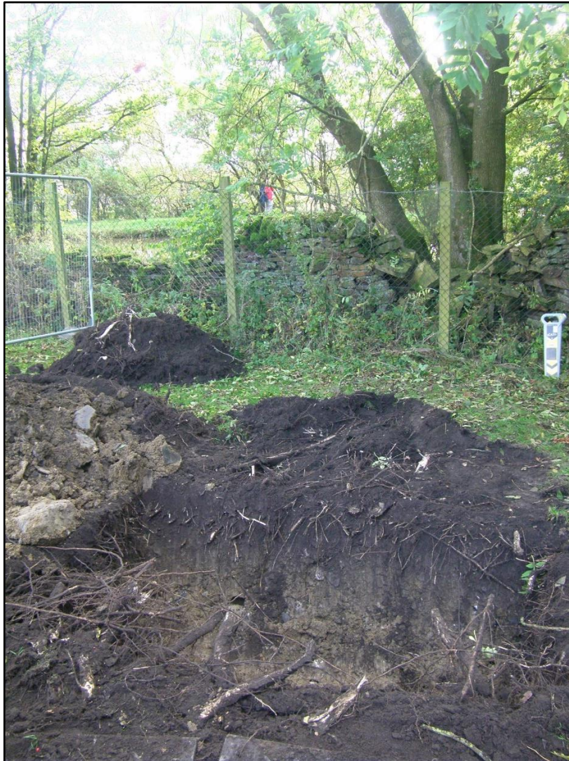
Plate 3: Reception Pit 2 showing accumulation of topsoil and subsoil and substantial root disturbance. Looking south-east towards the Leeds and Liverpool Canal.
