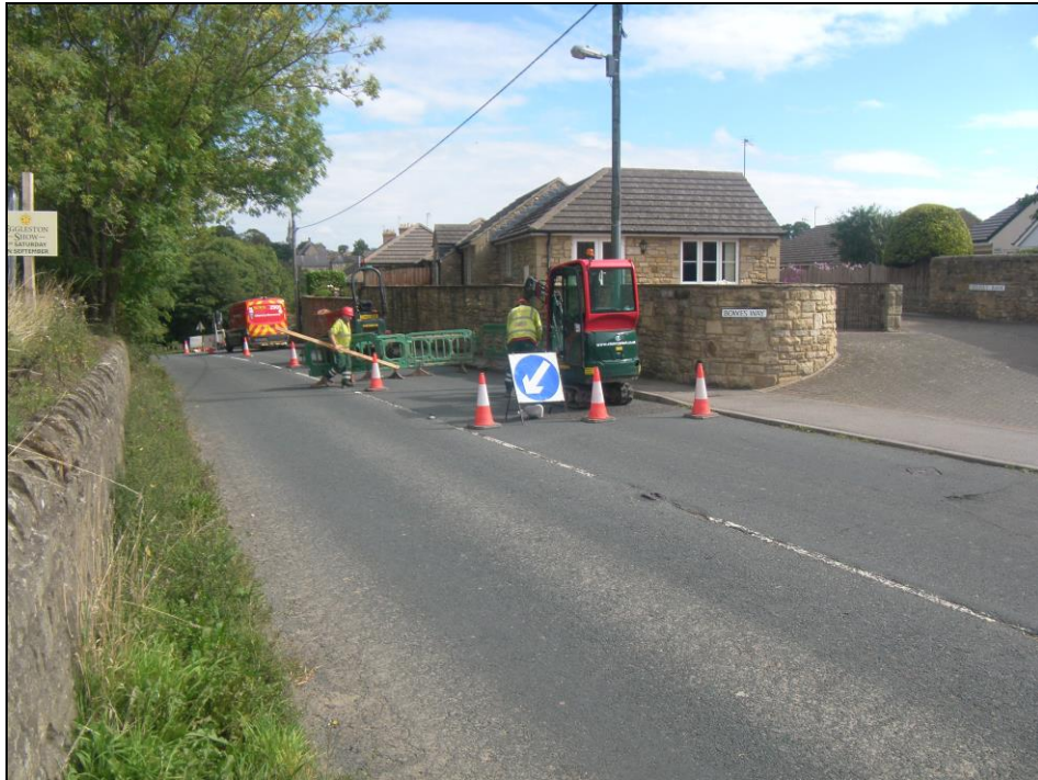
Plate 3. Location of Trench 3, looking north-eastwards towards Barnard Castle.
