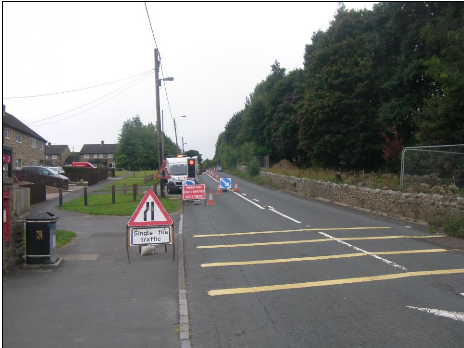
Plate 1: Overview of road crossing Trench 1 looking south-westwards, towards Corn Close.
