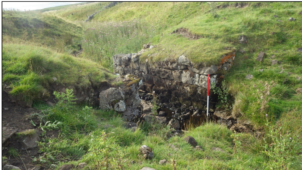
Plate 5: bridge footings HA76, facing south-west
