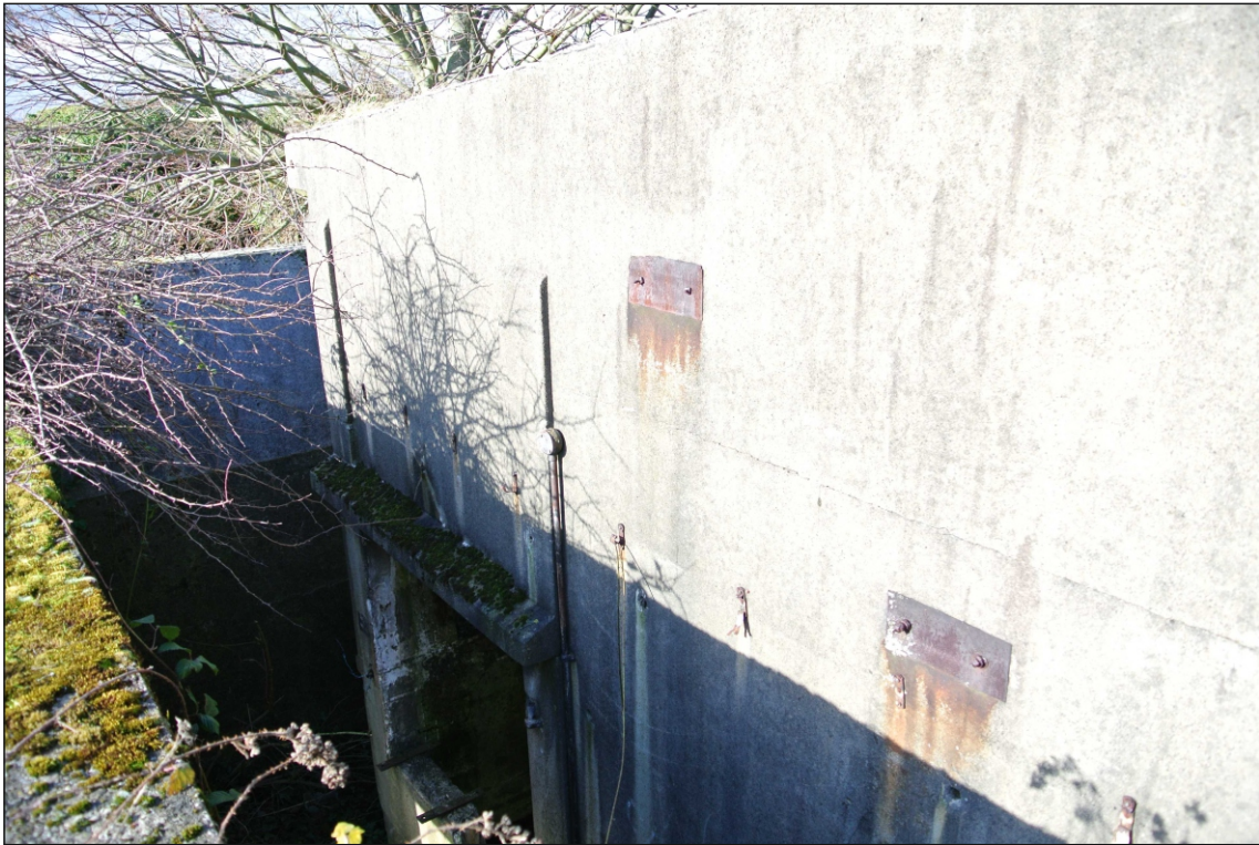
Former Killingworth Stores: Bunker A, south-west corner, showing Plate 19 blast wall around entranceway into the structure
