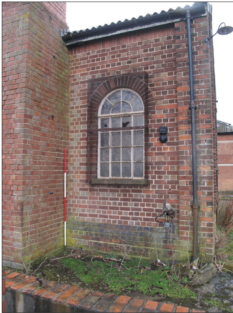
Former Killingworth Stores: Building 10, north bay of the eastern elevation, with arch-headed window and chimney to left
