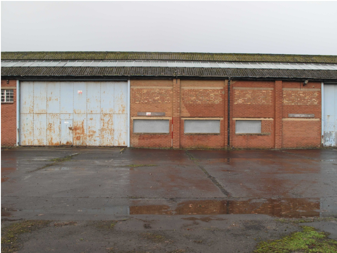
Former Killingworth Stores: Building 12, centre of southern elevation, showing vehicle access door and altered window arrangement
