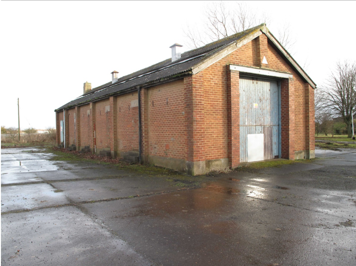
Former Killingworth Stores: Building 14, showing vehicle door in west gable and series of entranceways along north side
