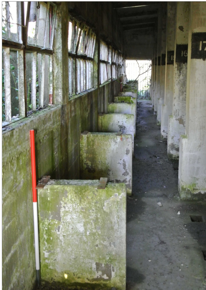
Former Killingworth Stores: Plate 21 Bunker A, showing concrete plinths for conveyor, and position of windows
