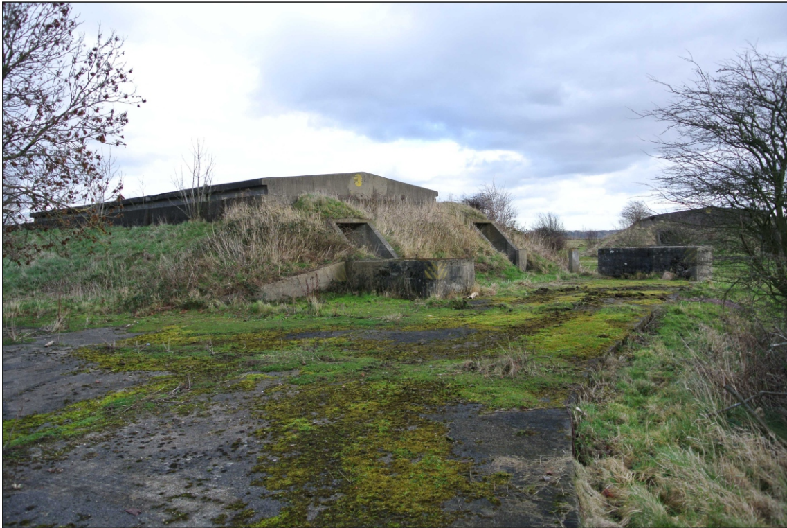
Former Killingworth Stores: Bunker C, south end, showing asymmetrical positioning of external loading platforms
