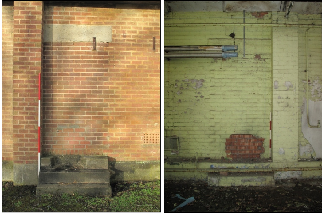
Plate 40: (left) brick patching on one of the southern pedestrian doors. (Right) interior view of same door
