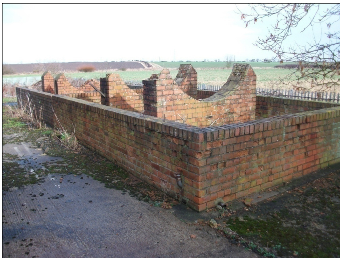
Plate 16: the bunded fuel tank which was situated to the north-east of Building 10
