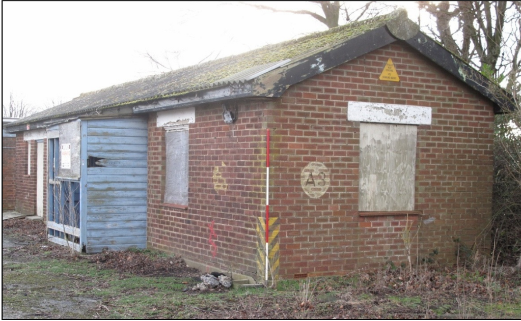
Plate 46: the north-east corner of Building 16
