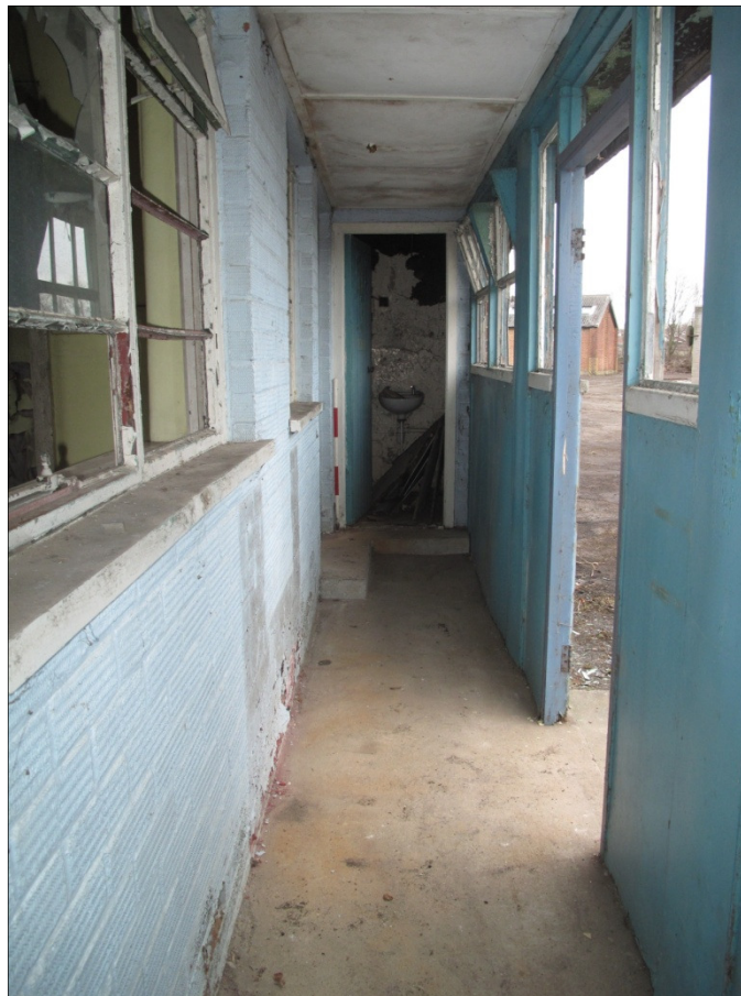
Plate 57: the enclosed porch, looking towards the L-shaped step and toilet room
