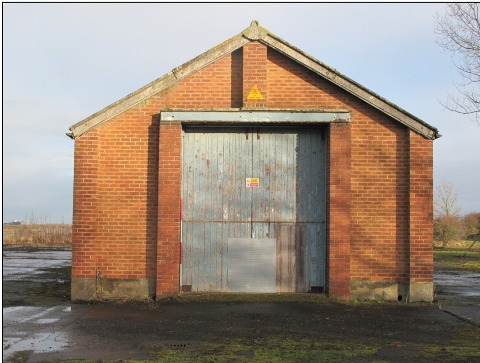
Plate 38: the western elevation of Building 14, showing the reinforced door surround
