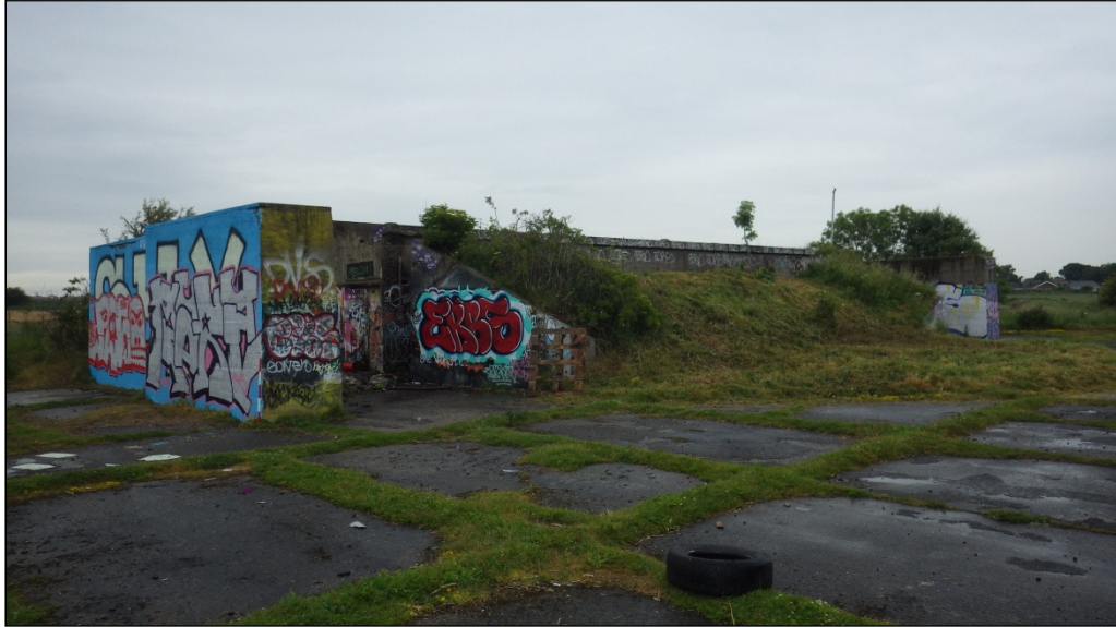
Plate 65: (above) the bunkers at East Boldon – with L-shaped blast walls. (Below) Bunker B, showing the slumped earth bunding, and entrances at the gable end
