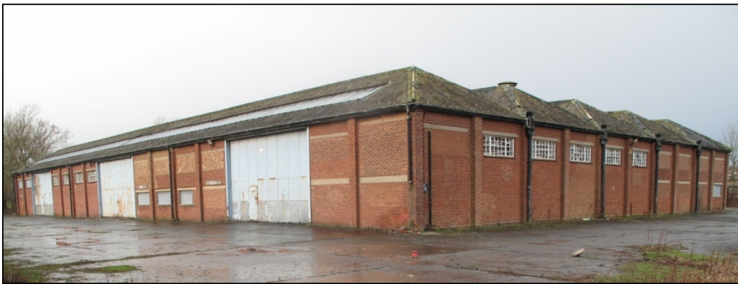
Plate 21: the south and east elevations of Building 12, showing the three large vehicular access doors, the roof structure and considerable alteration to the window positioning (above). A comparable view of the main store at East Boldon (below)
