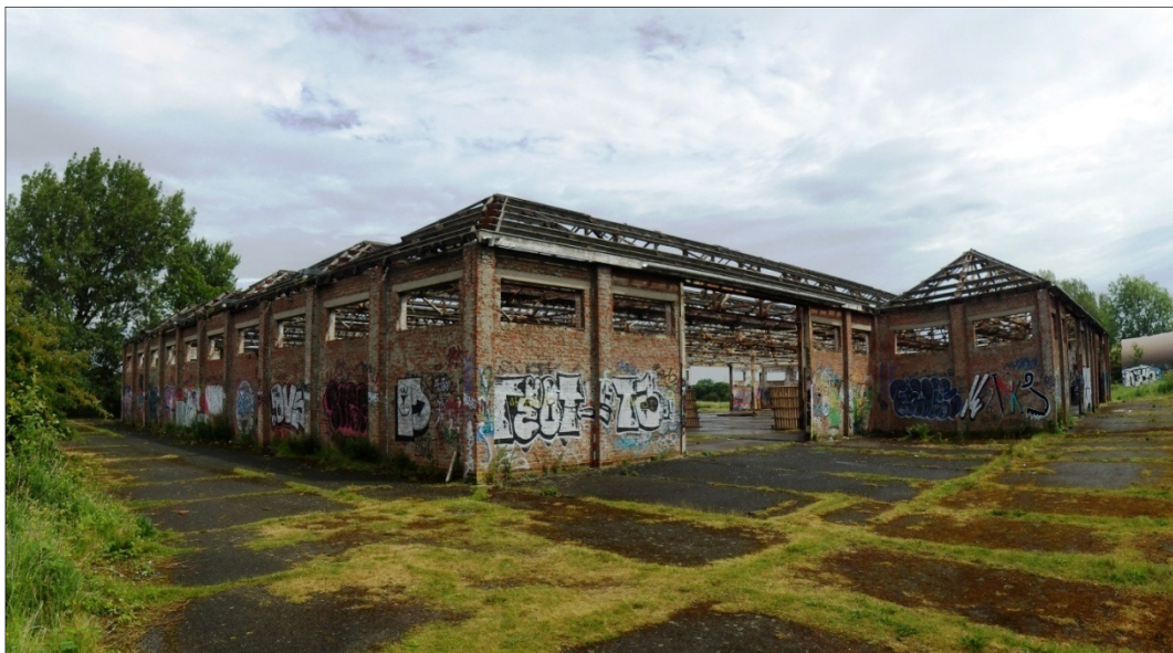
Plate 23: the north elevation of Building 12, showing two of the large vehicular doors, considerable window alteration and some markings on the concrete paving slabs (above). A comparable view of the main store at East Boldon (below)
