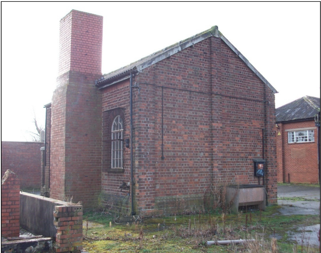
Plate 15: the north-east corner of Building 10, illustrating the later addition to the chimney, the original windows, and its relative position to the former bunded fuel tank. Building 12 can be seen in the background
