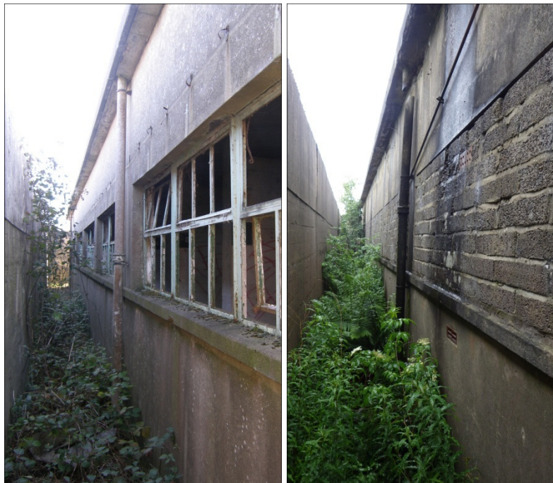
Plate 72: windows, Bunker C (left), and walled up windows, East Boldon bunker
