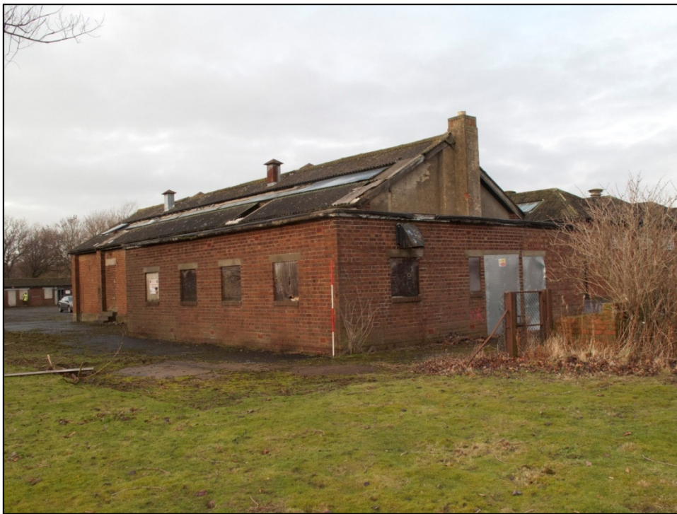
Plate 41: the later extension on the south-eastern corner of Building 14
