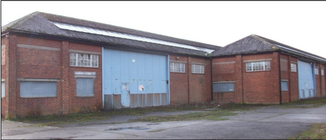
Plate 23: the north elevation of Building 12, showing two of the large vehicular doors, considerable window alteration and some markings on the concrete paving slabs (above). A comparable view of the main store at East Boldon (below)
