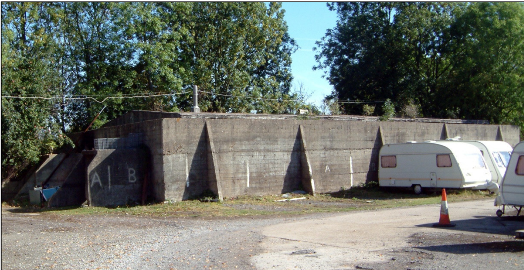
Plate 68: (top) Bunker E after the removal of bund, revealing the underlying concrete structure. (Below) denuded bunker at Banstead, Surrey, 2003 (courtesy Roger Thomas)
