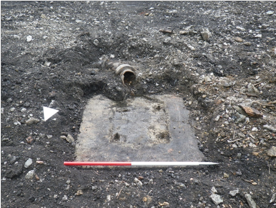
Plate 29: concrete RSJ foundations with remains of down-pipe on south side
