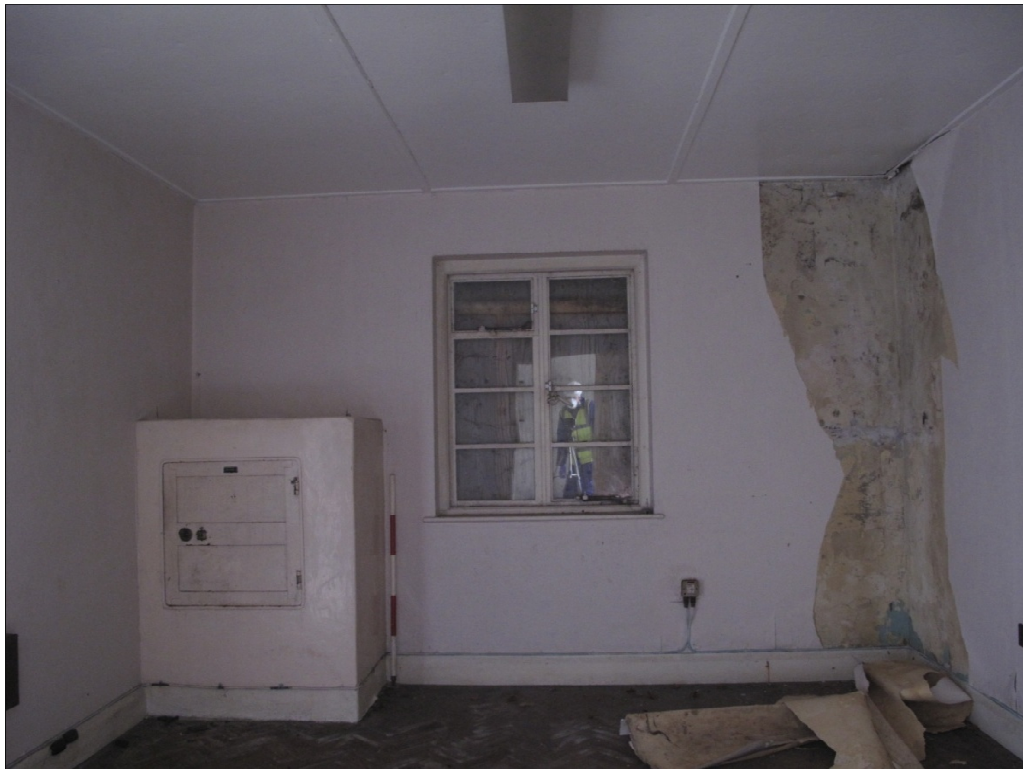
Plate 50: the northern room, looking north towards the safe
