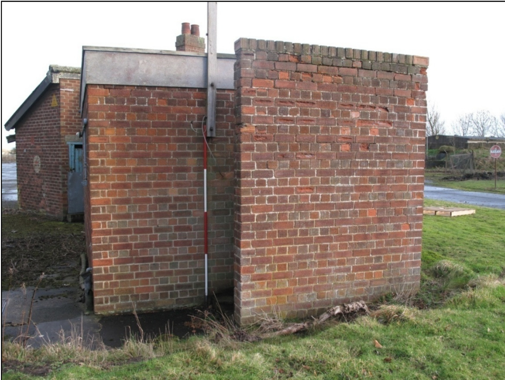
Plate 60: the west elevation of Building 19, showing the unroofed extension sheltering the main entrance. Building 17 can be seen in the background to the left
