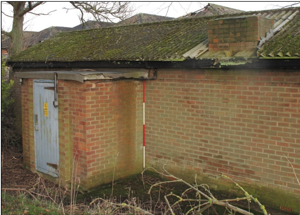
Plate 47: the rear extension, and the chimney, on the western elevation
