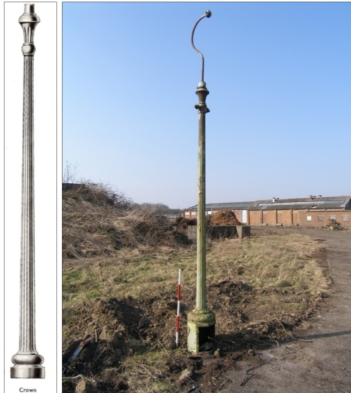
Plate 76: 'Crown' post from contemporary catalogue (left) and adjacent to road (right)
