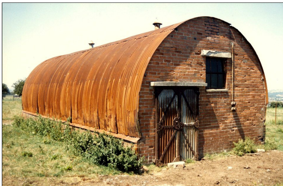
Plate 8: storage building at Burnett, Shropshire (© Folly Books) 5 ; note steel security door common for bunkers
