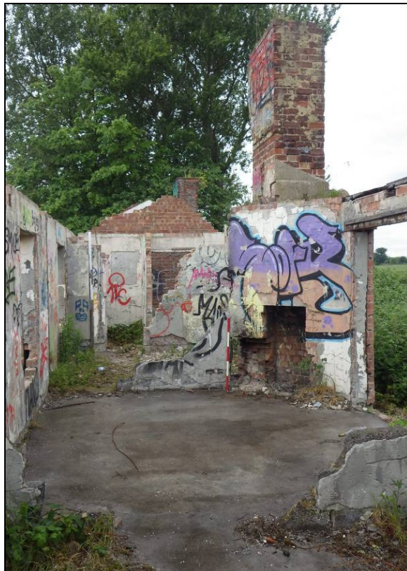
Plate 49: the main reception area in the admin block at East Boldon
