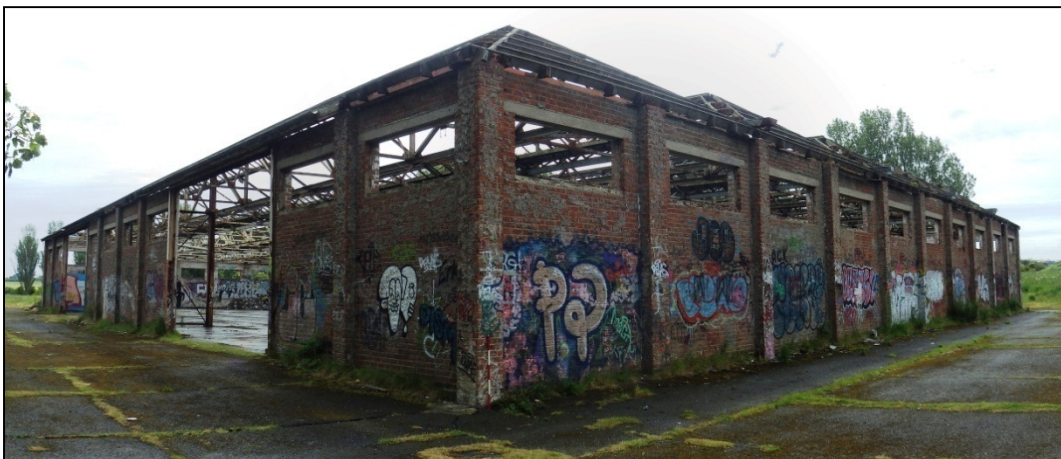
Plate 21: the south and east elevations of Building 12, showing the three large vehicular access doors, the roof structure and considerable alteration to the window positioning (above). A comparable view of the main store at East Boldon (below)
