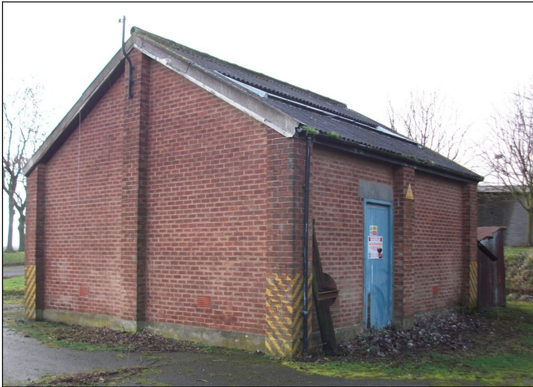
Plate 10: Building 4, facing south-west
