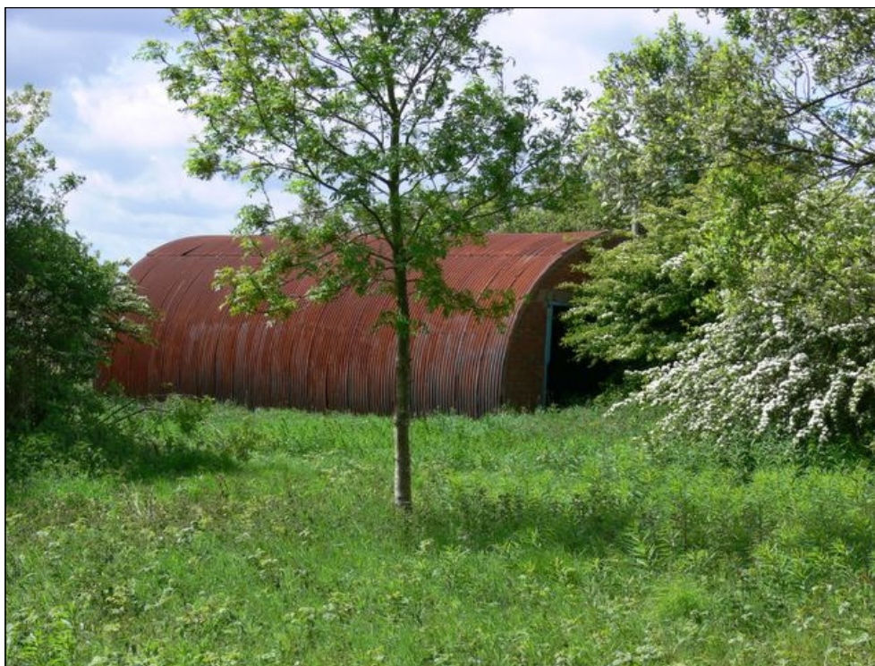
Plate 7: southern building in the cluster forming Building 2 – a probable Nissen hut (© Cannybevvy 4 )
