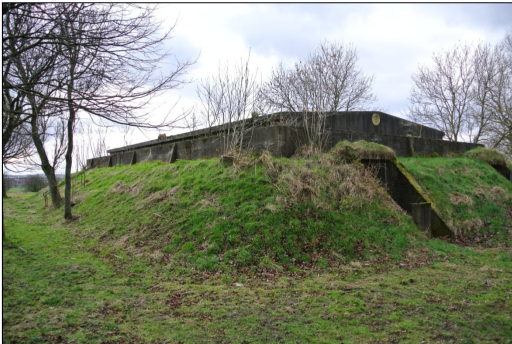
Plate 65: (above) the bunkers at East Boldon – with L-shaped blast walls. (Below) Bunker B, showing the slumped earth bunding, and entrances at the gable end
