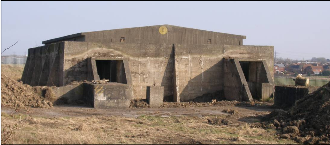
Plate 68: (top) Bunker E after the removal of bund, revealing the underlying concrete structure. (Below) denuded bunker at Banstead, Surrey, 2003 (courtesy Roger Thomas)
