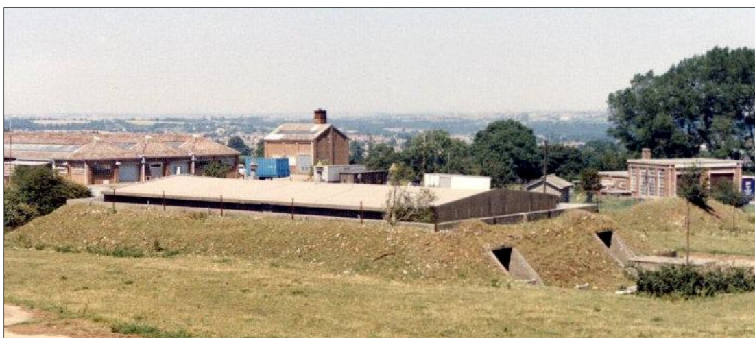
Plate 12: Burnett AAOD, Shropshire; main store and boiler house, with bunker in the foreground and double garage/tender shed to the right (© Folly Books) 8
