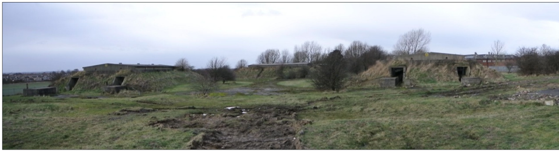
Plate 64: Bunkers E and D, facing west
