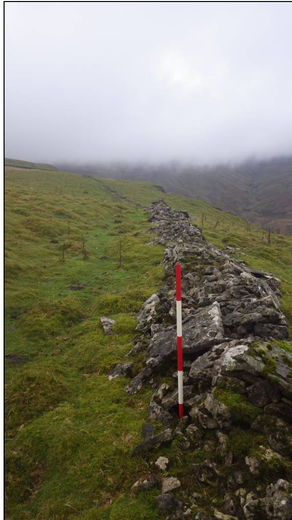
Plate 3: drystone wall 10002, facing south
