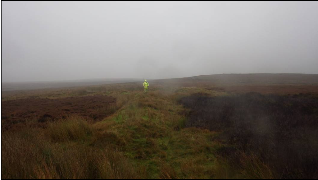
Plate 7: Merryfield Old Dams 10011 , facing east
