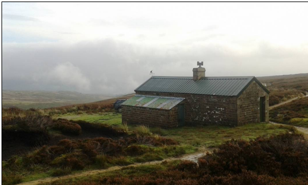
Plate 1: Burn Edge House, on Burn Gill, towards the northern edge of the survey area
