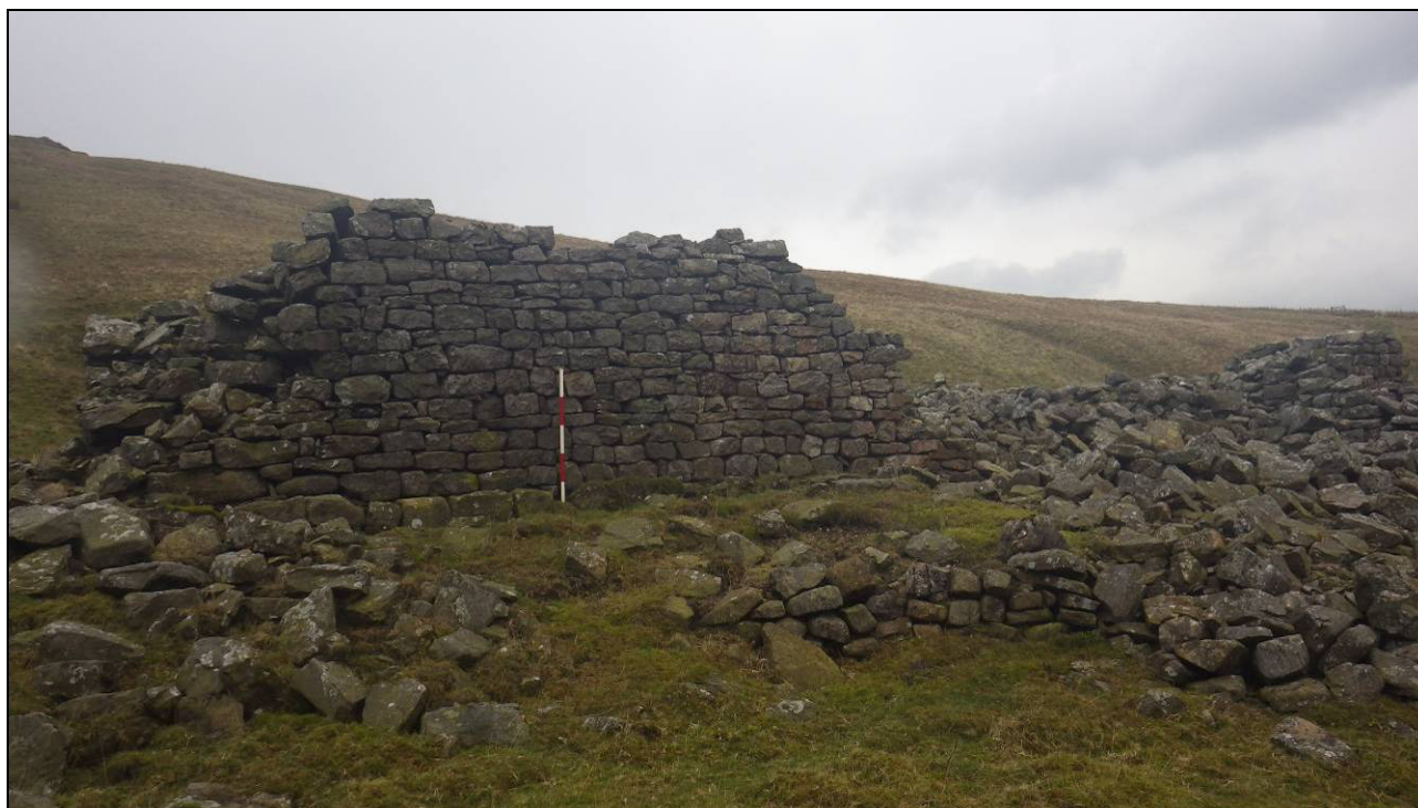
Plate 7: the north (exterior) side of room F, showing the fine stone work. The smaller wall in the foreground D was used to divert water off the wheel-pit, which lies to the right of the photograph.
