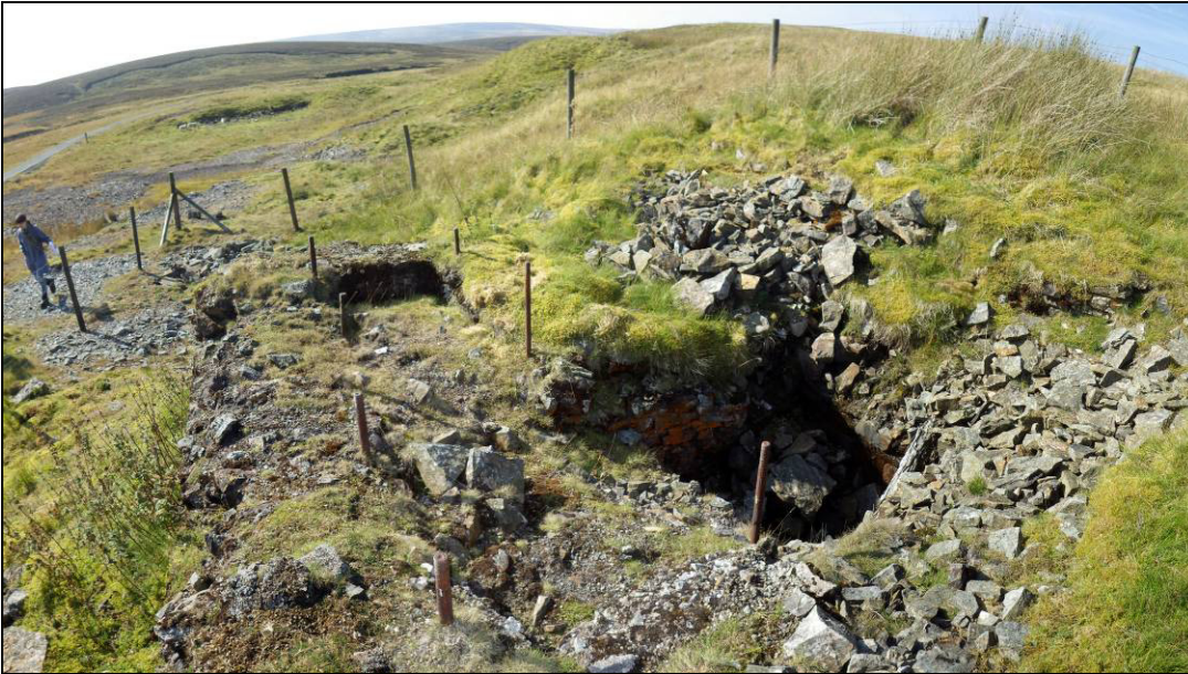
Plate 14: Providence Shaft, facing south; the dressing floor and Troutbeck Foot Level lie in the middle distance
