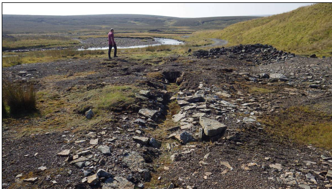
Plate 13: culvert with crushing mill adjacent (right of picture), facing east
