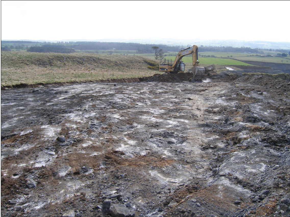
Barrasford Quarry: bedrock below shallow topsoil at north western half of site
