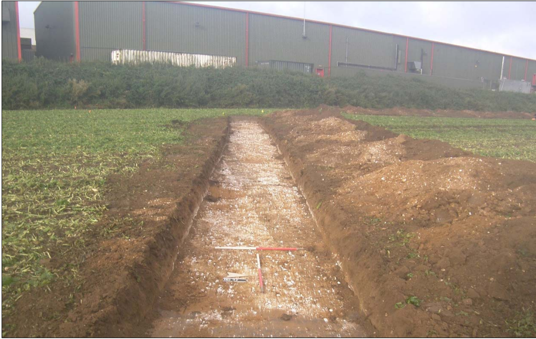
Plate 5: Trench 37, cable trench 26, pre-excitation, looking west.
