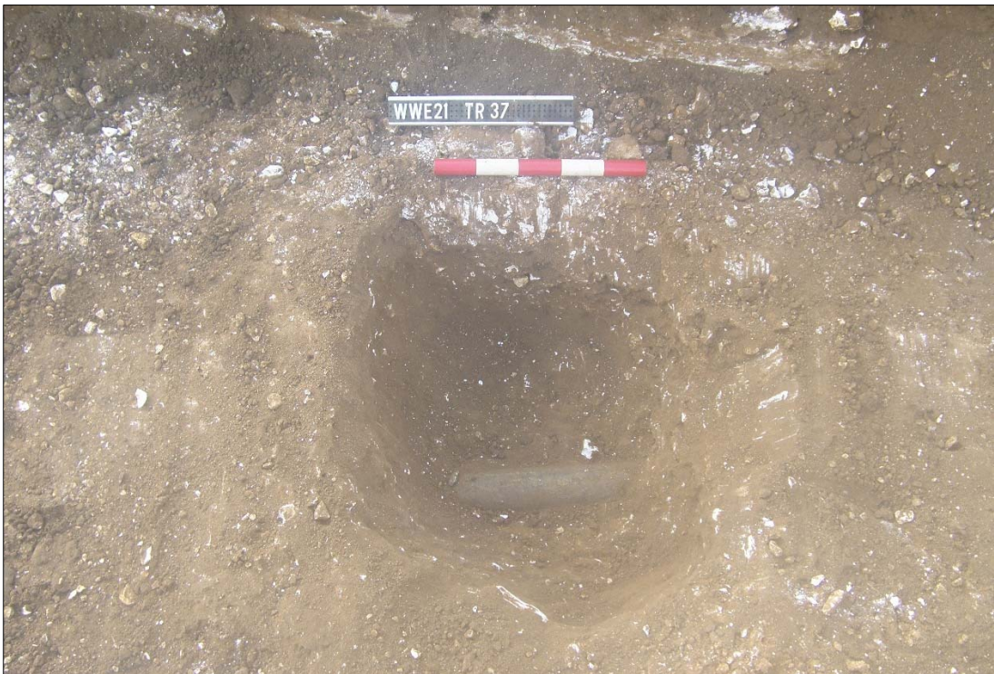
Plate 6: Trench 37, slot excavated in cable trench 26 showing original metal cable-housing in situ.
