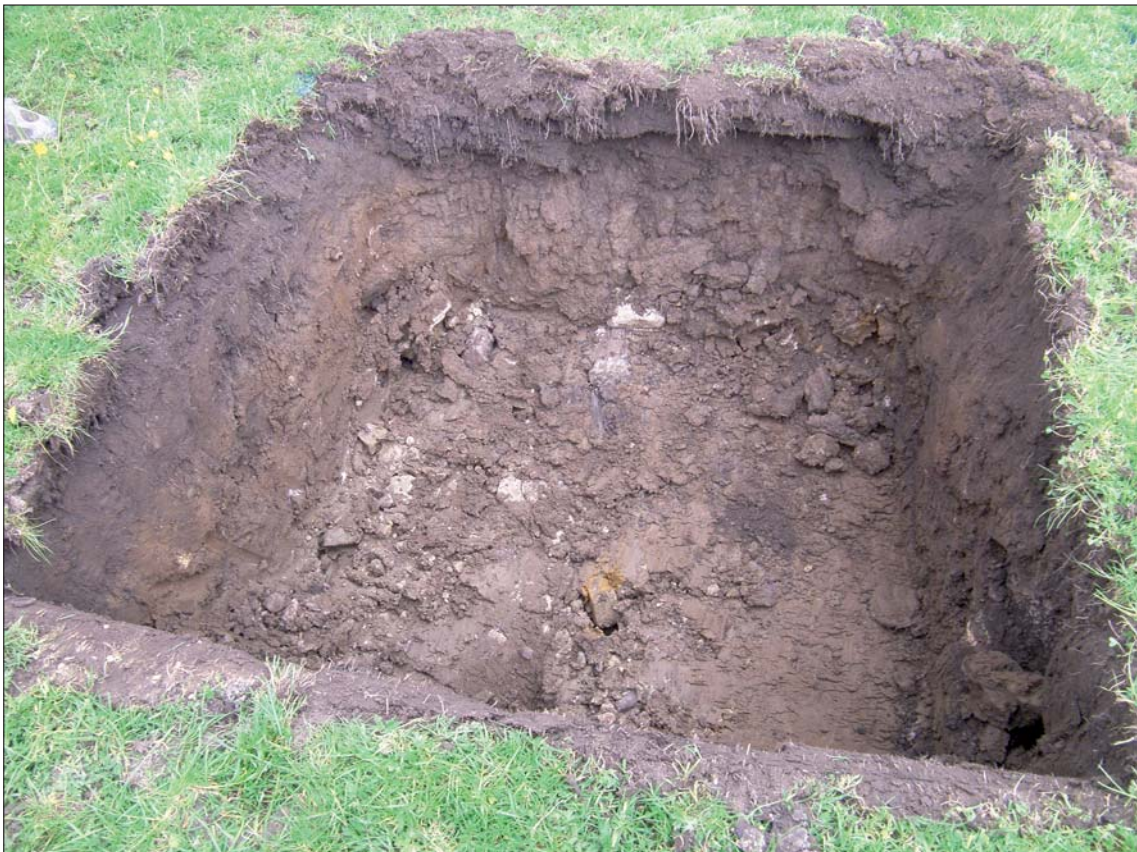
Cracoe to Rylstone Pipeline Scheme: the Launch Pit, excavated to the upper level of the natural boulder clay
