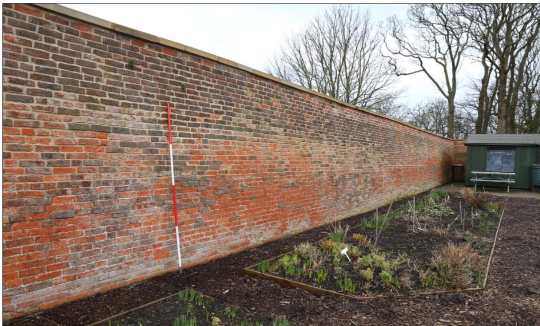
Plates 26: east end of the south-facing elevation of the north wall.
