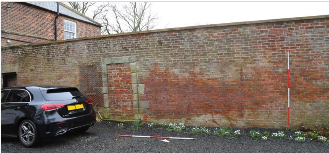
Plate 28: doorway 311 and opening 314 just visible behind the car.
