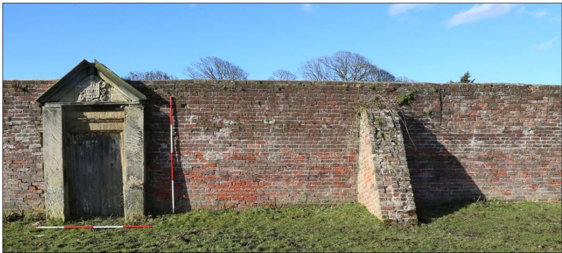
Plate 37: doorcase 413, buttress 411 and infill section 412.
