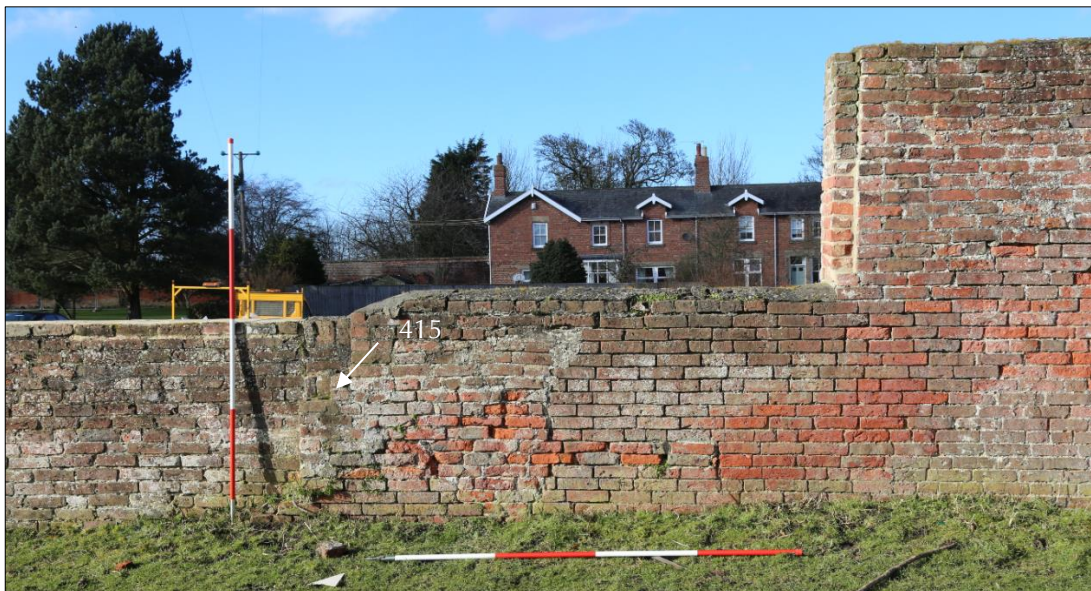
Plate 41: change in wall height and section of blocking 415 .
