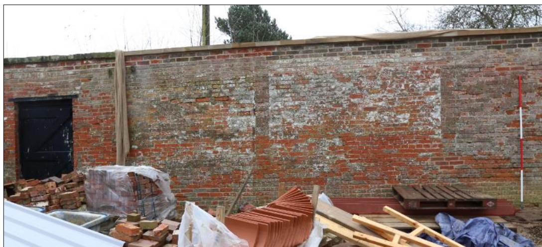
Plate 14: wall render, wall scars ( 213 ) and door ( 214 ); all evidence of early 20th-century buildings which formerly stood against the north-facing elevation at the west end of the walled garden.
