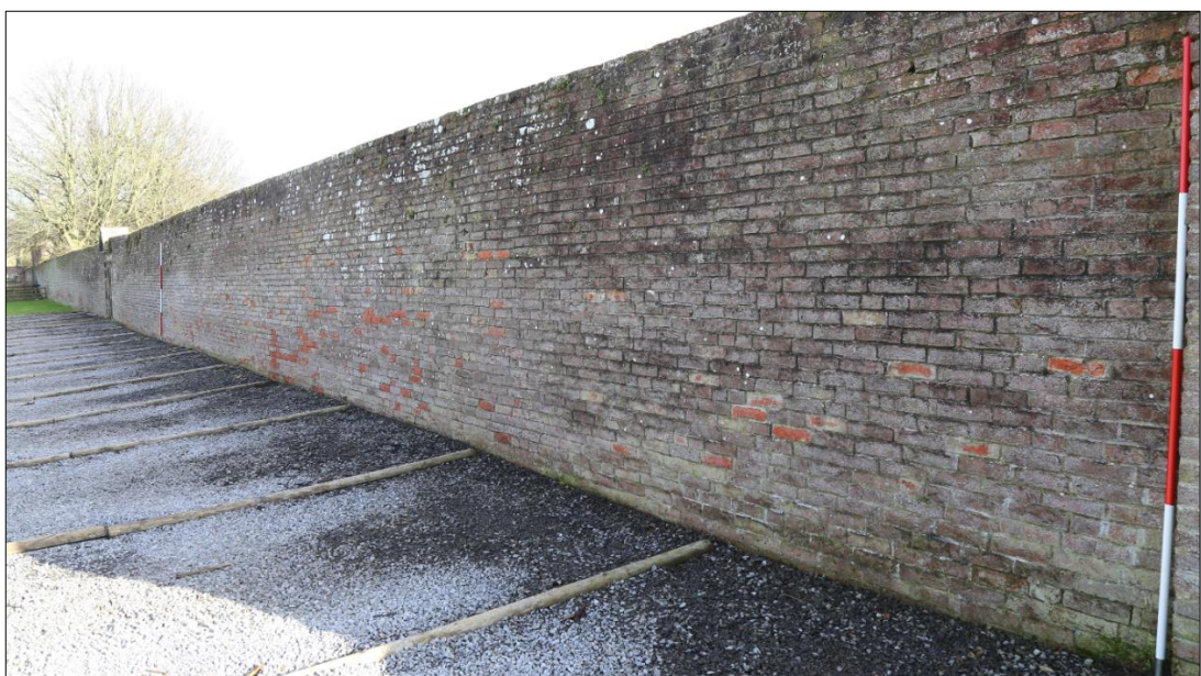
Plate 48: north-facing elevation with door 413 just east (left) of second ranging rod.
