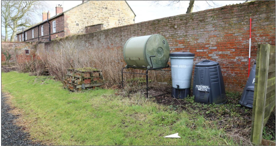
Plate 49: east end of north-facing elevation.
