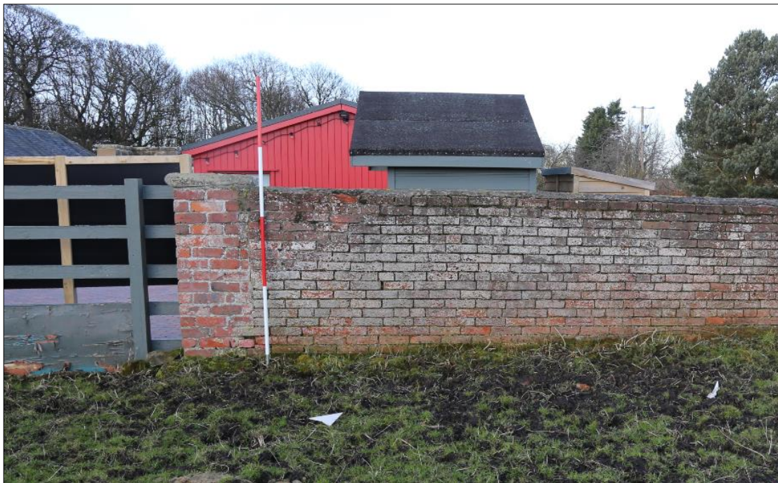
Plate 46: gatepost 421 at the west end of south wall.
