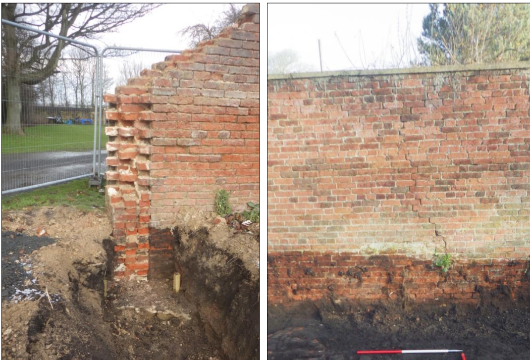
Plates 51 and 52: (left) cross-section through the wall exposed during dismantling; (right) sample section of brickwork with concrete capping.
