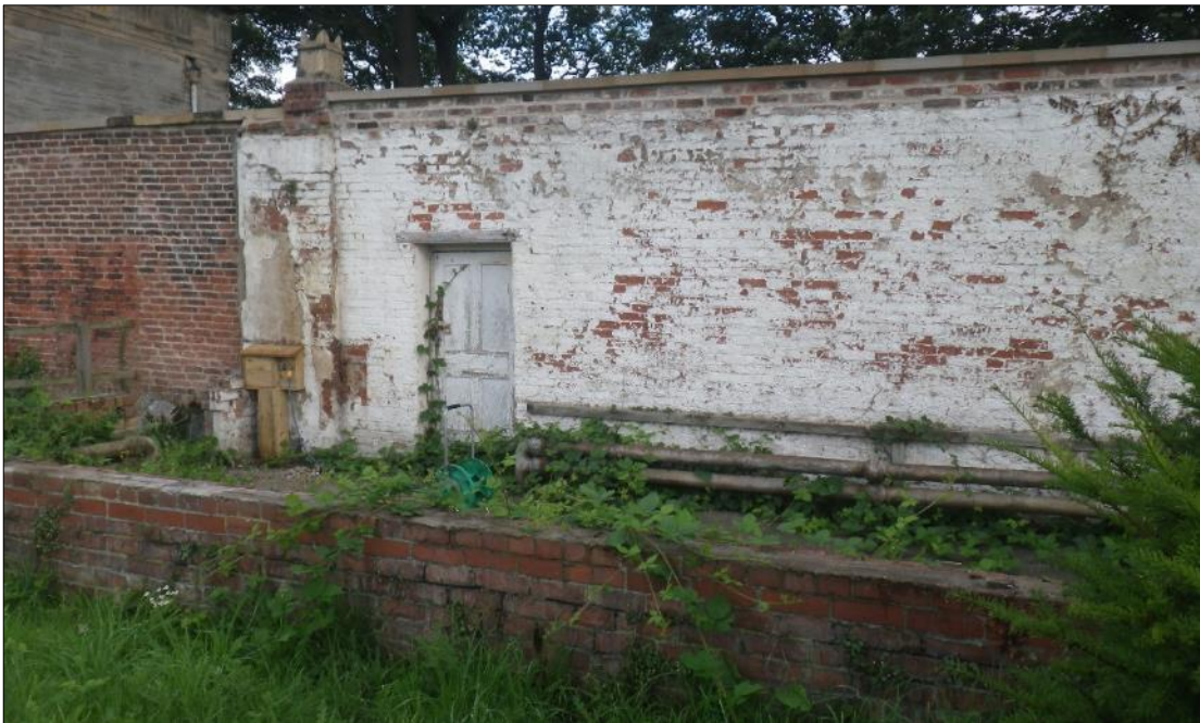
Plate 6: greenhouse site after demolition with chimney and cast-iron pipes.
