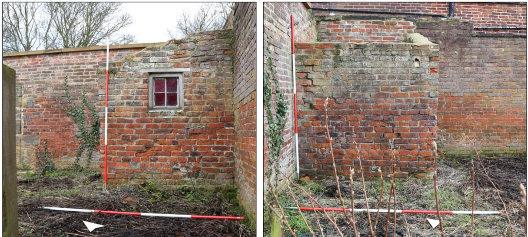
Plates 31 and 32: structure 321 (left) west-facing elevation; (right) north-facing elevation.
