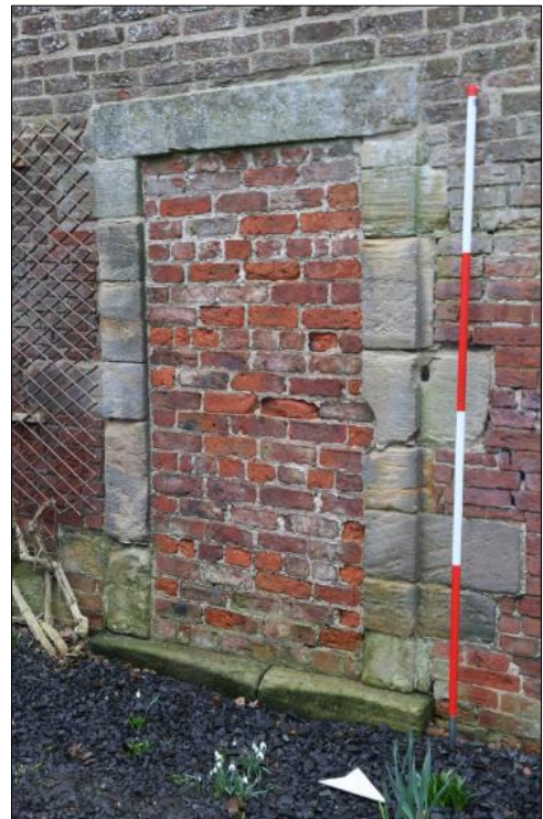
Plates 12 and 13: (left) blocked doorway (211) prior to consolidation. Reproduced with kind permission Mosedale Gillatt Architects; (right) door at the southern end of the east wall (311).
