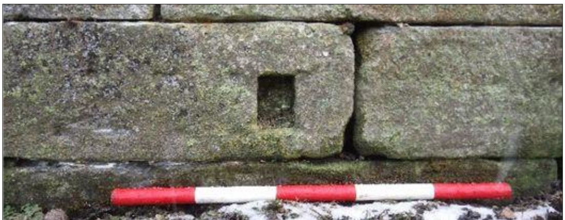
Plates 54: carved recess in north-east bastion wall for gate.
