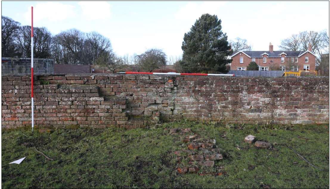
Plate 44: stepped brickwork (417) and buttress 418.
