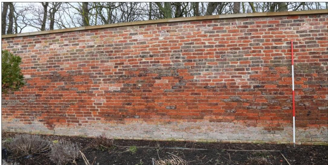
Plate 33: example section of west-facing (internal) elevation of east wall, showing brickwork.
