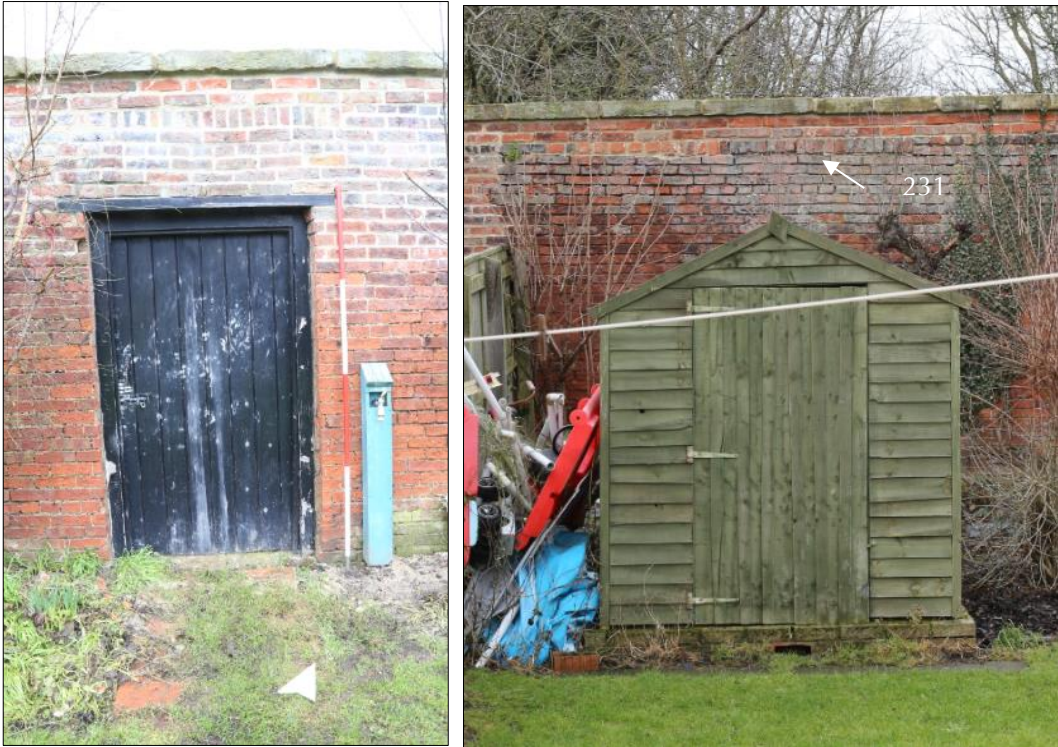
Plates 21 and 22: (left) doorway 214; (right) line of slightly protruding headers (231).
