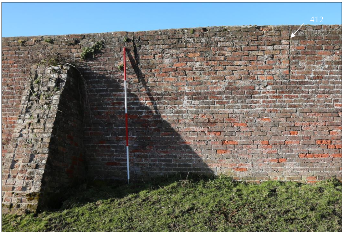
Plate 38: buttress and rectangular infilled brick panel (412).
