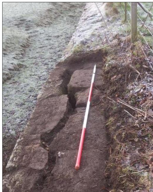
Plate 9: damage to the ha-ha wall.
