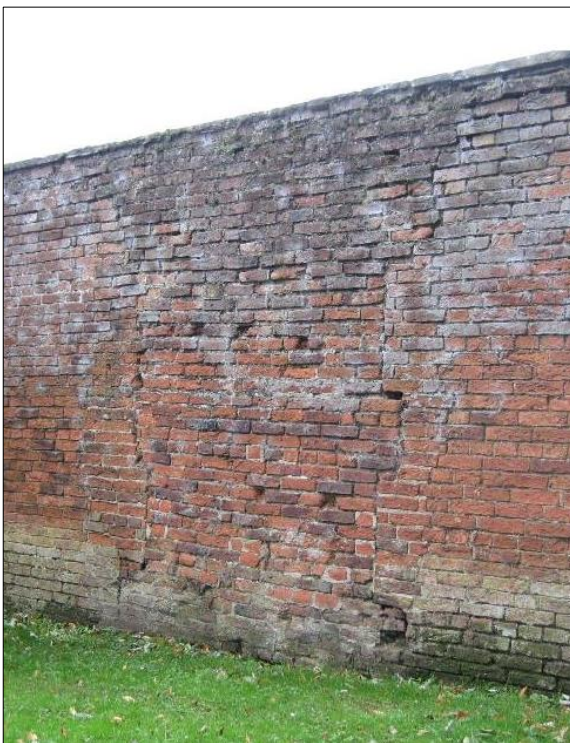
Plates 12 and 13: (left) blocked doorway (211) prior to consolidation. Reproduced with kind permission Mosedale Gillatt Architects; (right) door at the southern end of the east wall (311).
