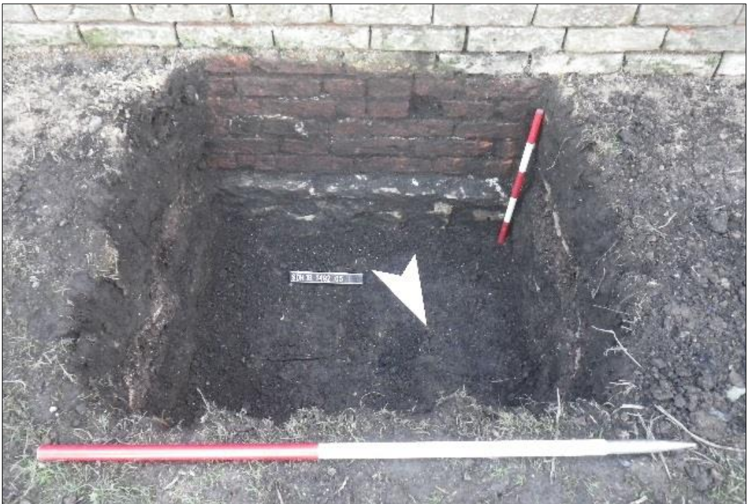
Plate 3: FP 2 – buttress trench showing the wall foundations.
