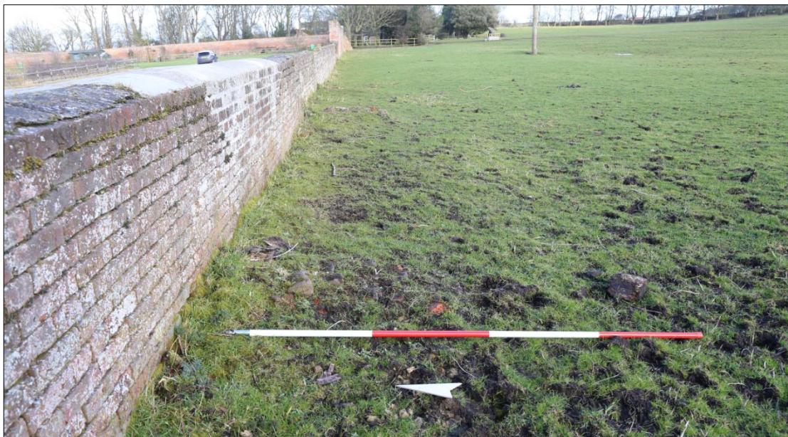
Plate 45: buttress 419 on south side of south wall.
