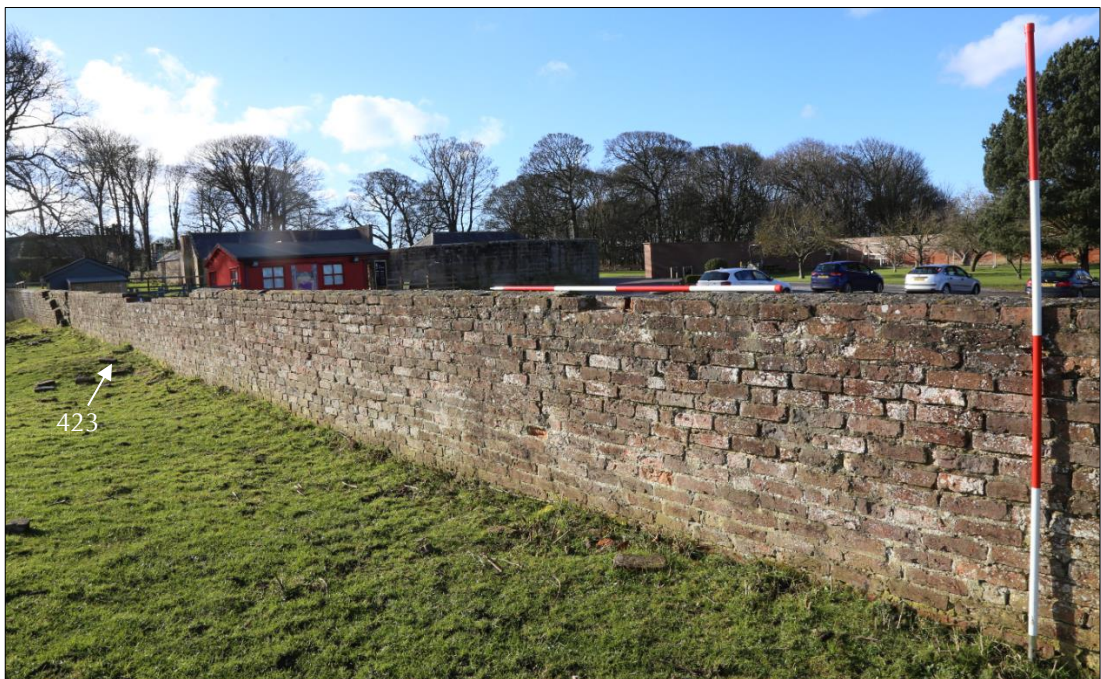
Plate 43: rebuilt section of south wall ( 416 ) with buttress 423 visible.
