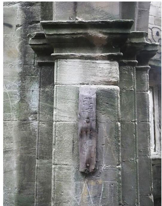
Plate 11: timber remains of wall 2006.
