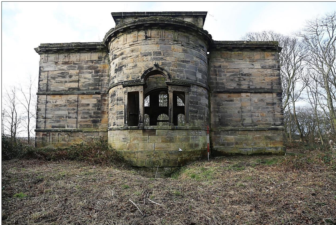
Plate 2: east-facing elevation with apse and vault entrance at ground level.
