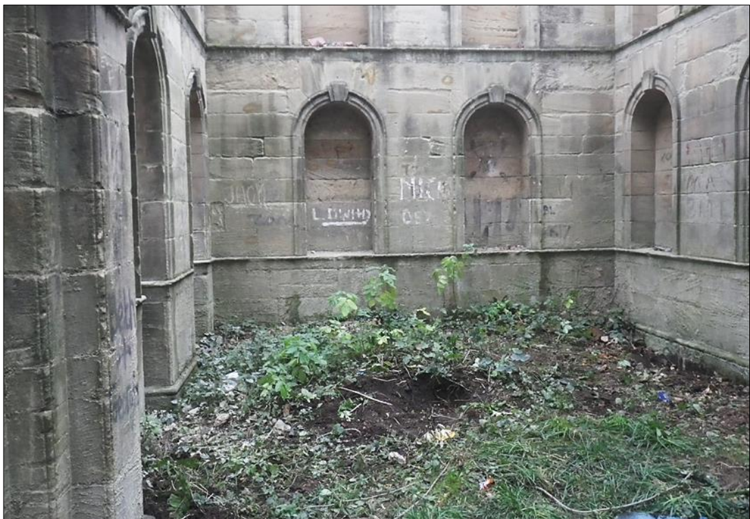
Plate 3: interior during initial clearance, facing north.
