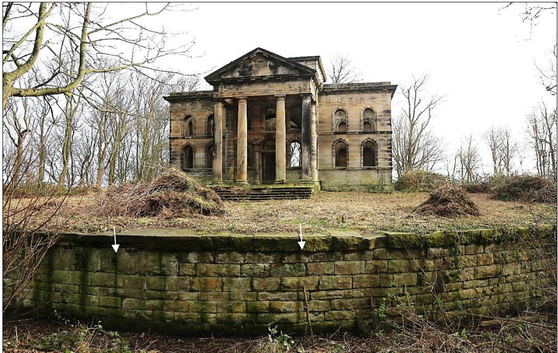
Plate 1: view across the ha-ha, showing the west-facing elevation and portico, with drawbridge masonry in foreground (between two white arrows).
