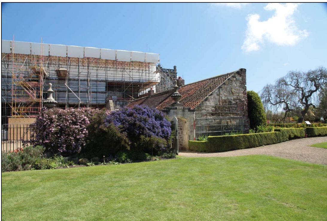
Plate 162: The Potting Shed makes a positive contribution to the settings of the gardens and hall, creating a pleasing contrast with the more formal architectural style of the Hall.
