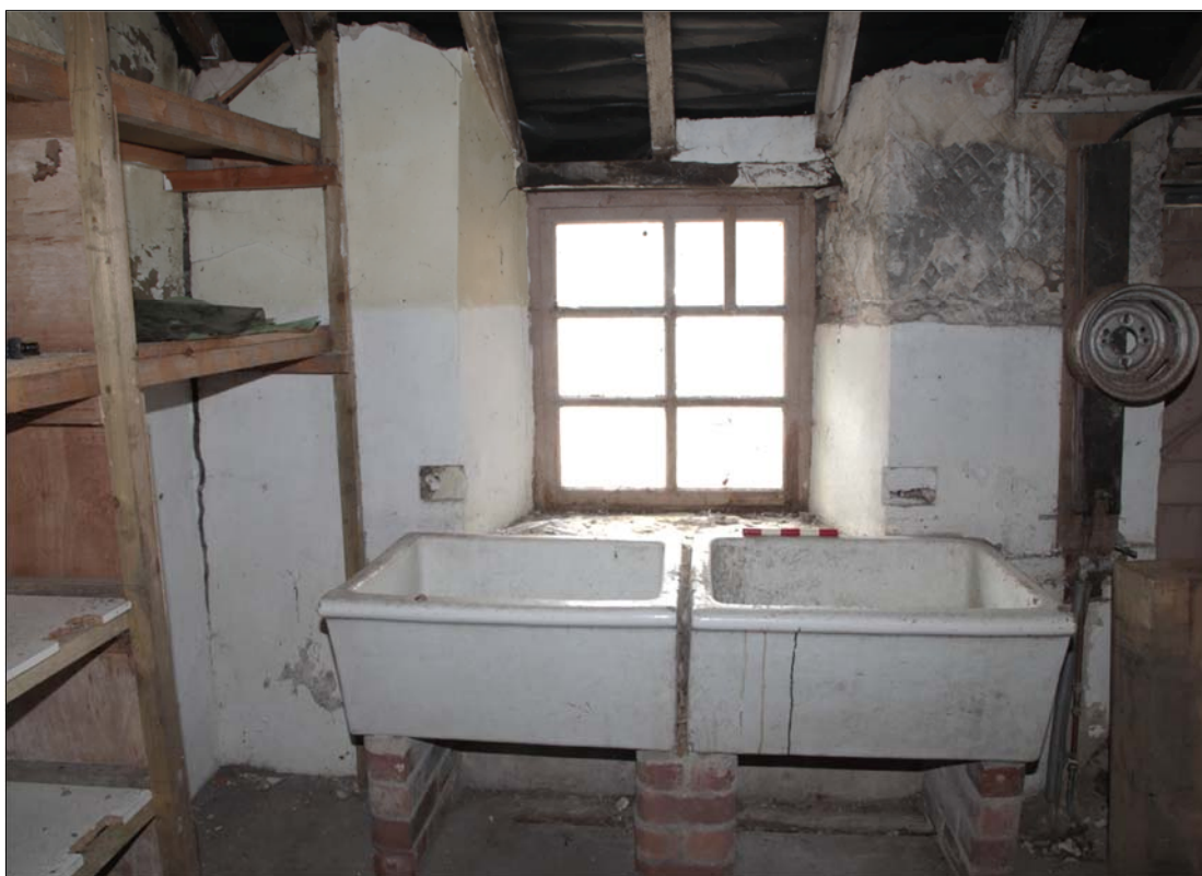
Plate 5: North wall (1130) of room (1100) showing the scullery sinks 1134 and window 1132.
