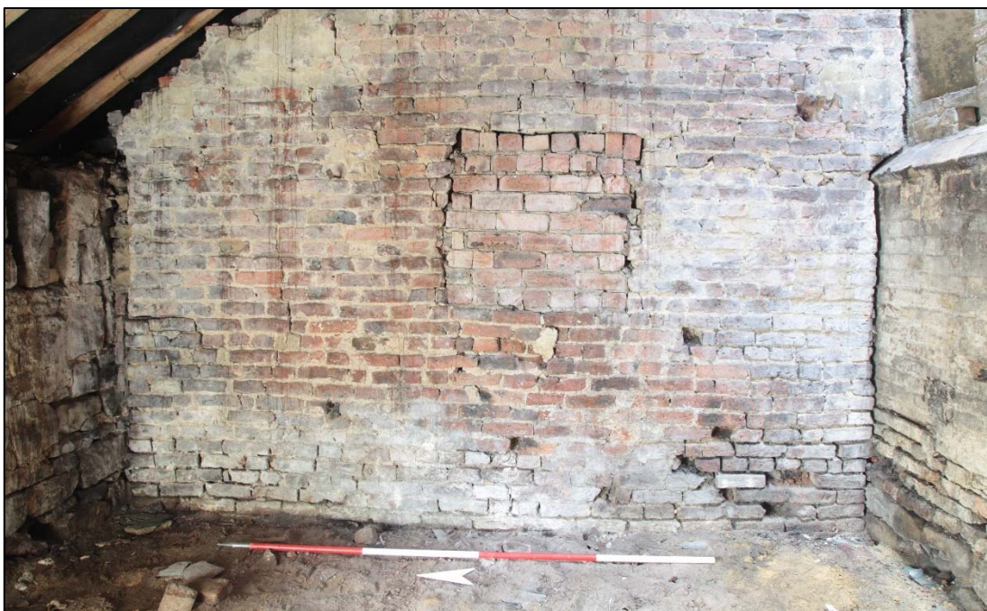
Plate 8: North-east elevation 1240 of the east-central room.
