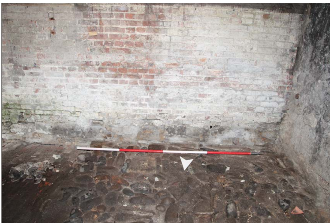
Plate 17: Foundation course (1413) of brick wall, visible in the south-west corner of 1400.
