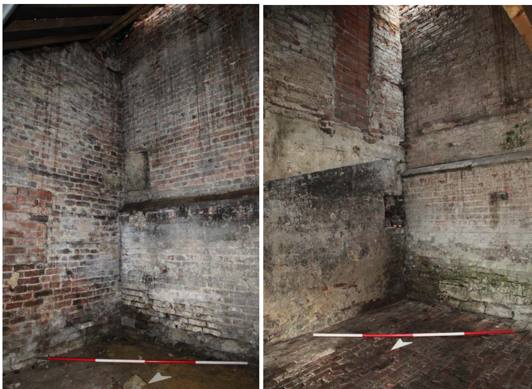
Plates 15: Later partition walls abutting rear brick boundary wall (300); (left) wall 1220 on the east side of room 1200, and (right) wall 1440 on the east side of room 1400.
