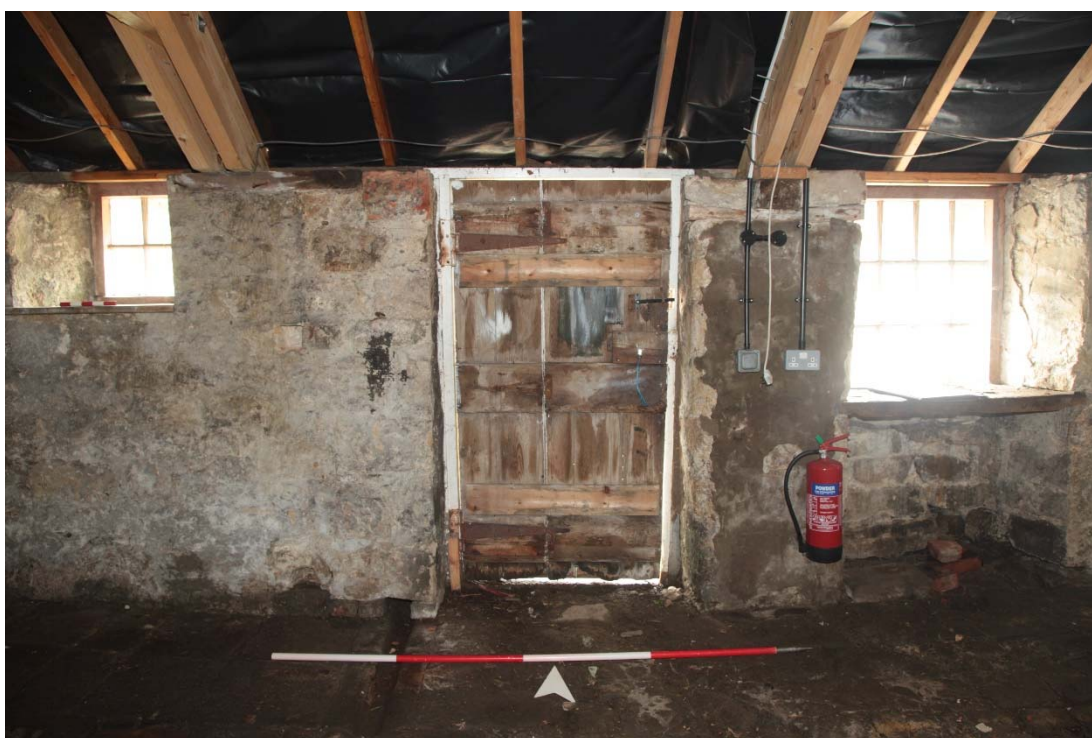
Plate 13: North-west wall 1430 of the west room.
