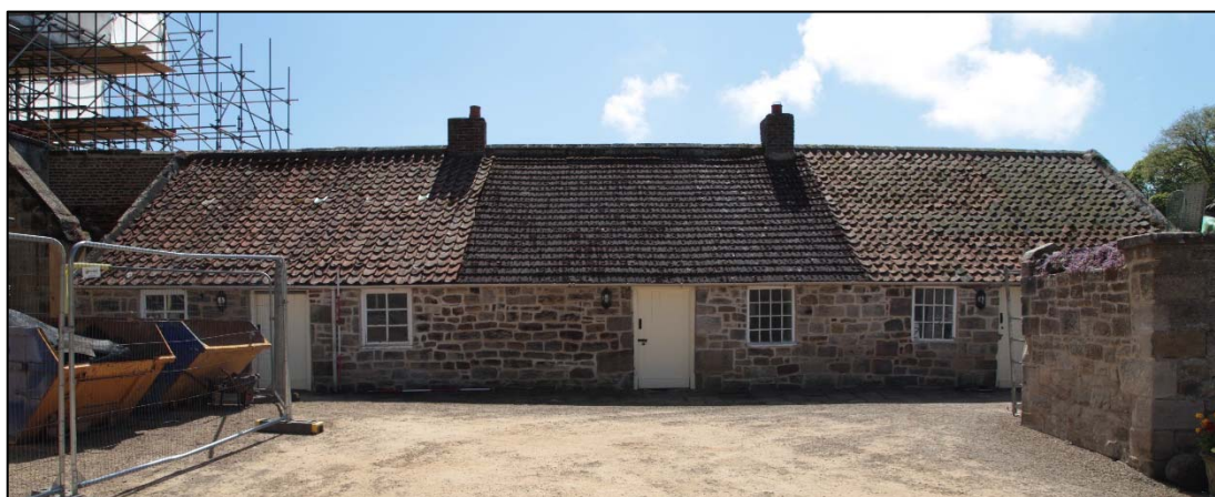
Plate 1: Front (north-facing) elevation of the Potting Shed looking south-east.
